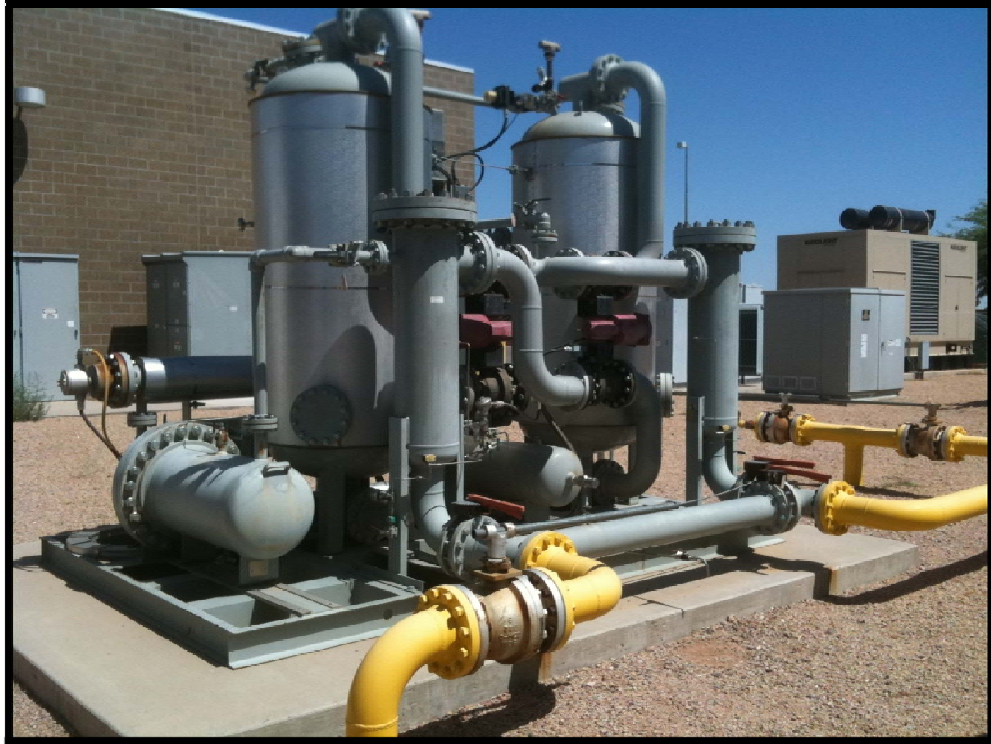
Figure 2-2 Gas Dryer at RPTA in Phoenix, Arizona
