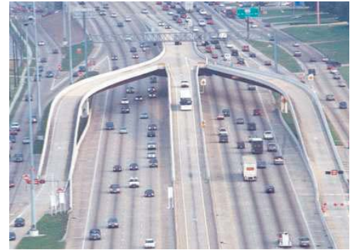
High Occupancy Vehicle lane in Houston
