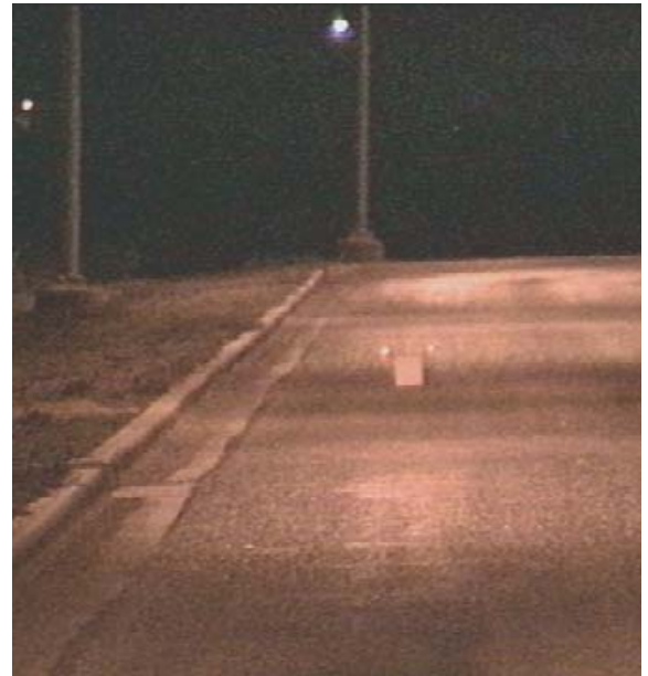
STV testing of roadway lighting
