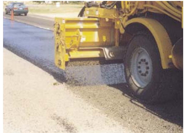
Application of aggregate during seal coat construction
