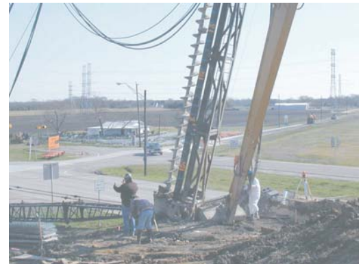
CFA pile installation for bridge foundation at Krenek Road and US 290 in Houston.
