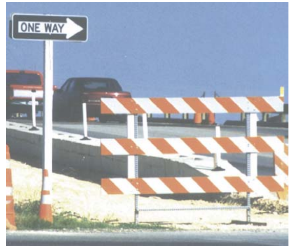
Barricades and temporary signing in construction work zone
