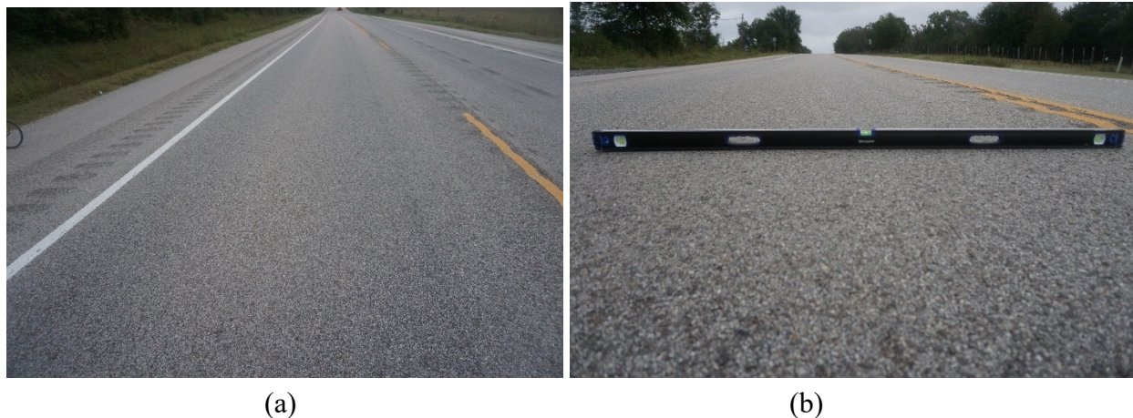
Figure 67. SH 7 Pavement Surface: (a) Cracking and (b) Rutting.
