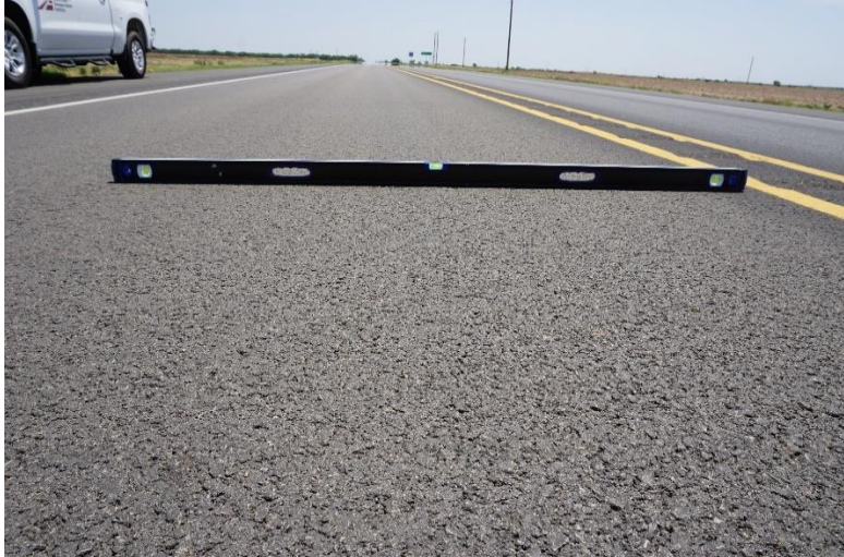
Figure 66. No Rutting on the Test Section with PG70-22 on FM 2105.
