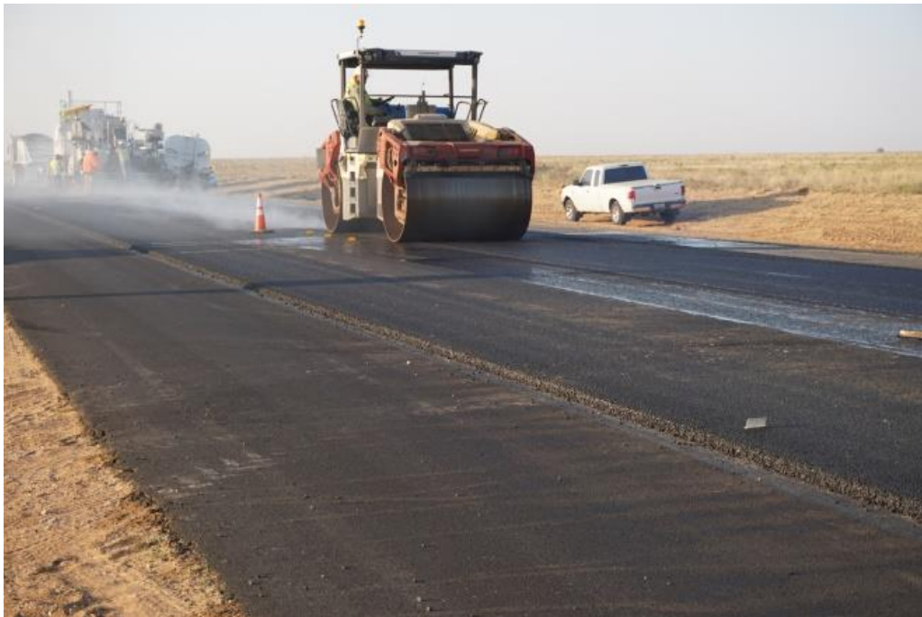
Figure 50. Compacting the Mat.
