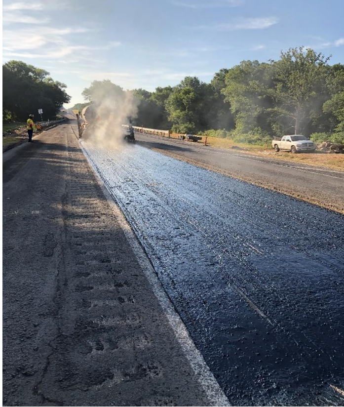
Figure 39. Applying Tack Coat.
