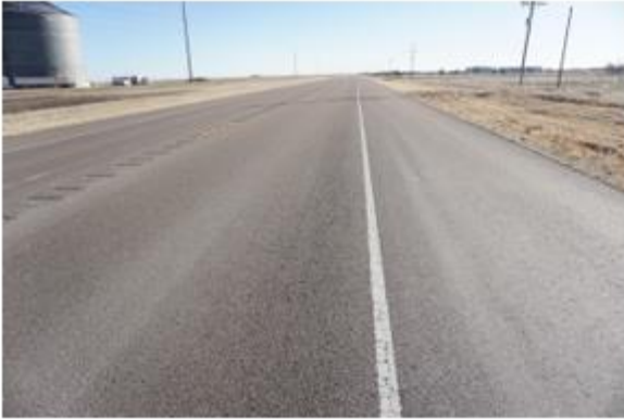
Alligator Cracking: 03/07/2017
