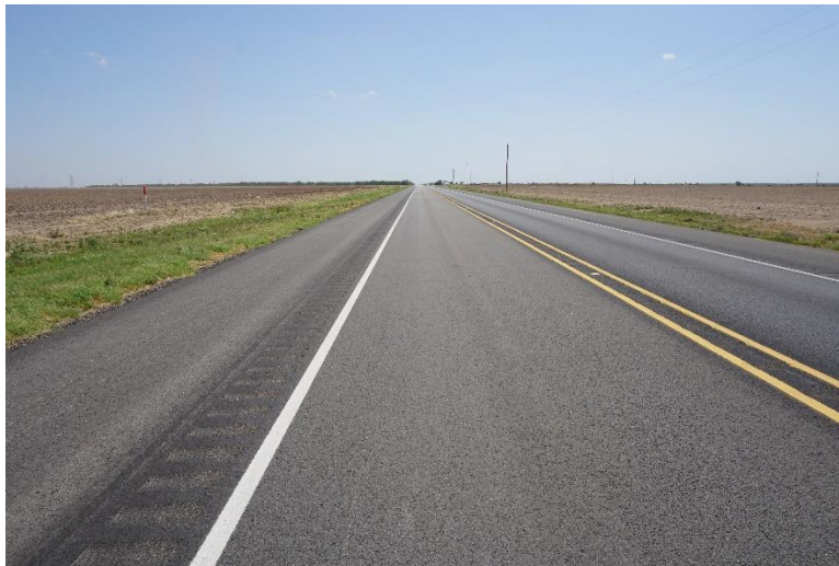
Figure 67. No Cracking on the Test Section with PG70-22 on FM 2105.
