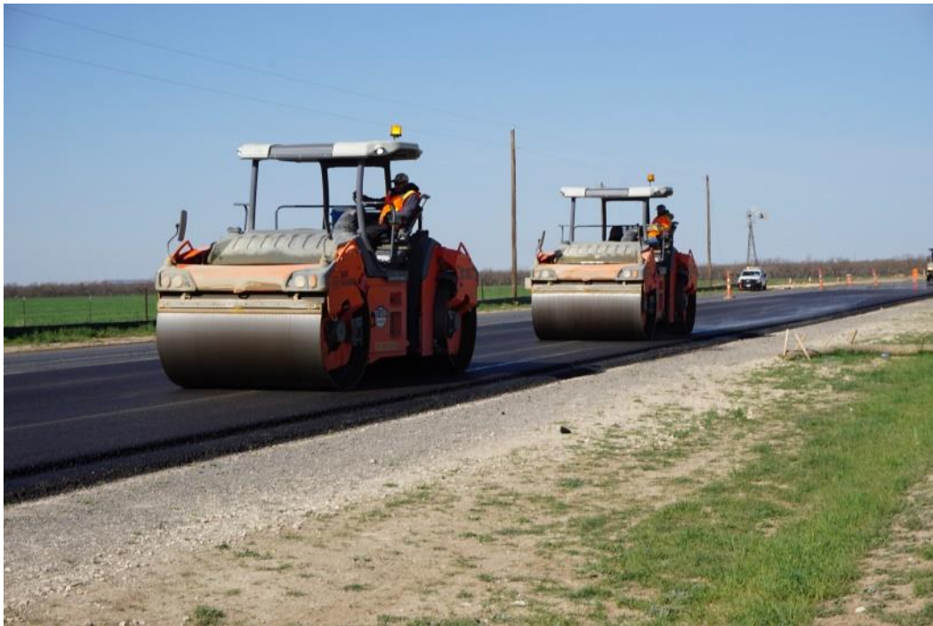
Figure 63. Compacting Test Sections on FM 2105.
