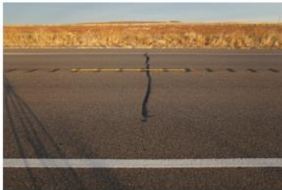
Transverse Cracking: 01/10/2018
