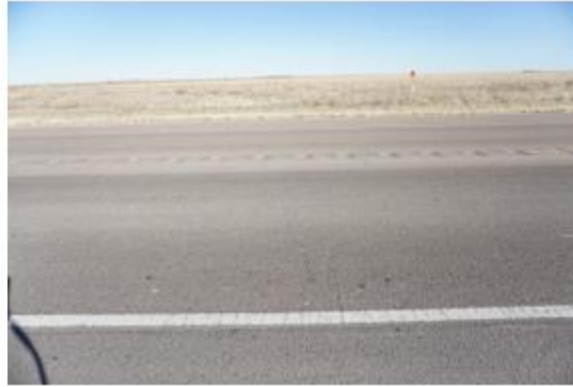
Transverse Cracking: 03/07/2017
