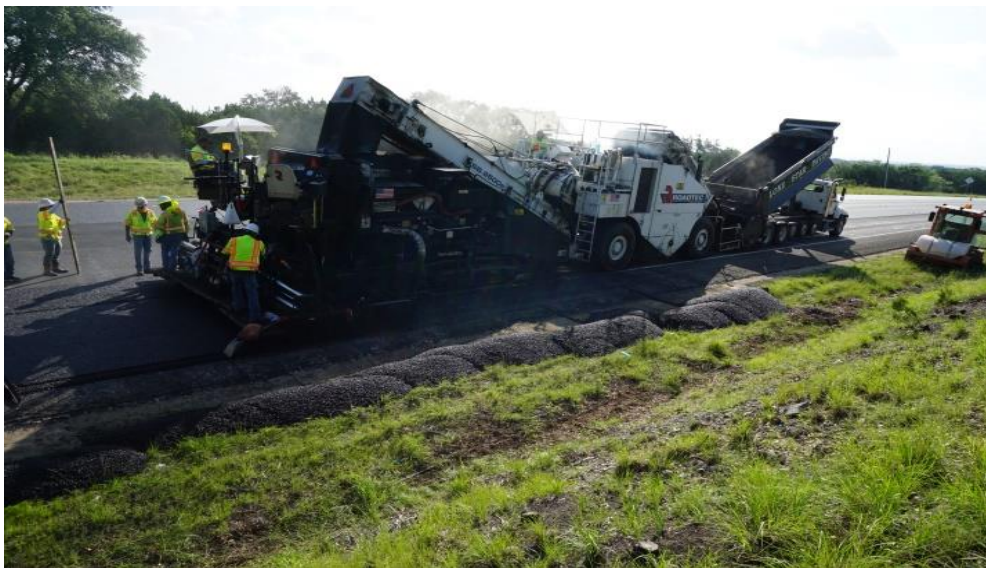
Figure 69. Paving Operation on SH 71.
