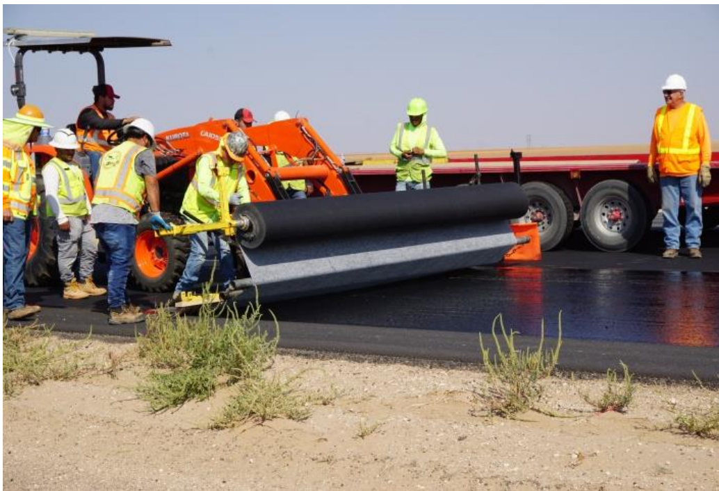
Figure 48. Paving Fiberglass Fabric Interlayer.
