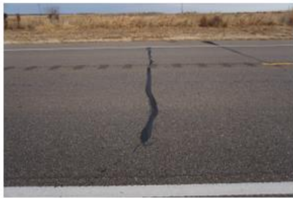
Transverse Cracking: 01/10/2018
