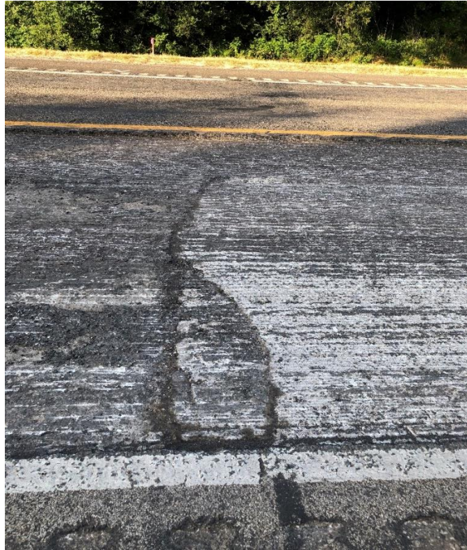
Figure 38. Example of SH 7 Pavement Condition after the 2-In. Milling.
