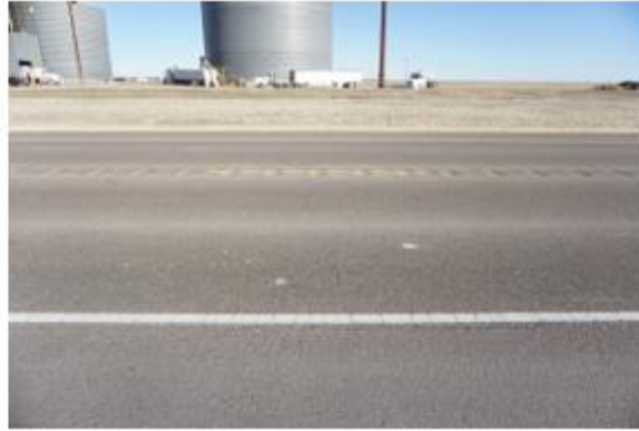
Transverse Cracking: 03/07/2017
