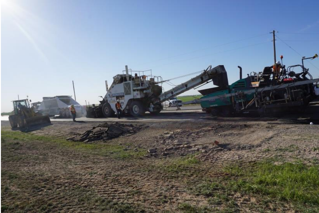
Figure 62. Paving Operation on FM 2105.
