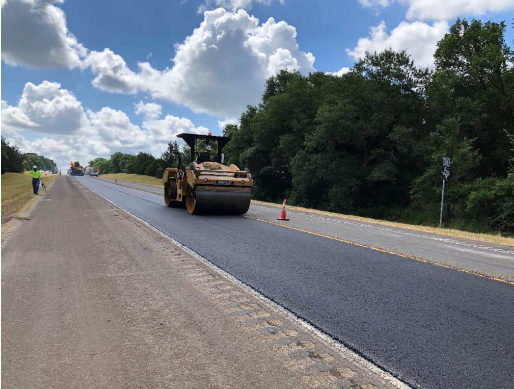
Figure 41. Compacting the Mat.
