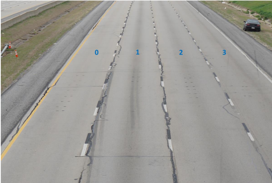
View from Quebec Bridge on 03/26/2018
