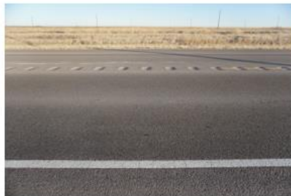
Transverse Cracking: 03/07/2017
