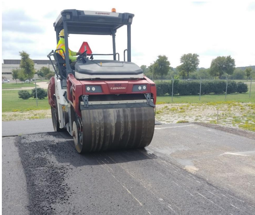
Figure 58. Compacting Test Sections at Dallas Test Sections.
