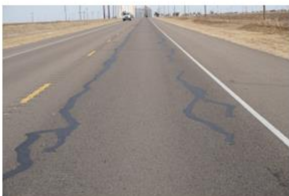
Overall Cracking: 01/10/2018
