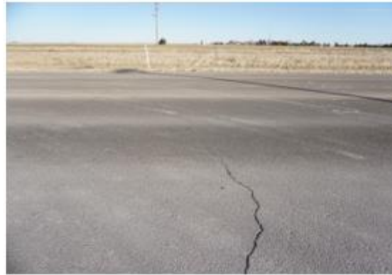
Transverse Cracking: 03/07/2017
