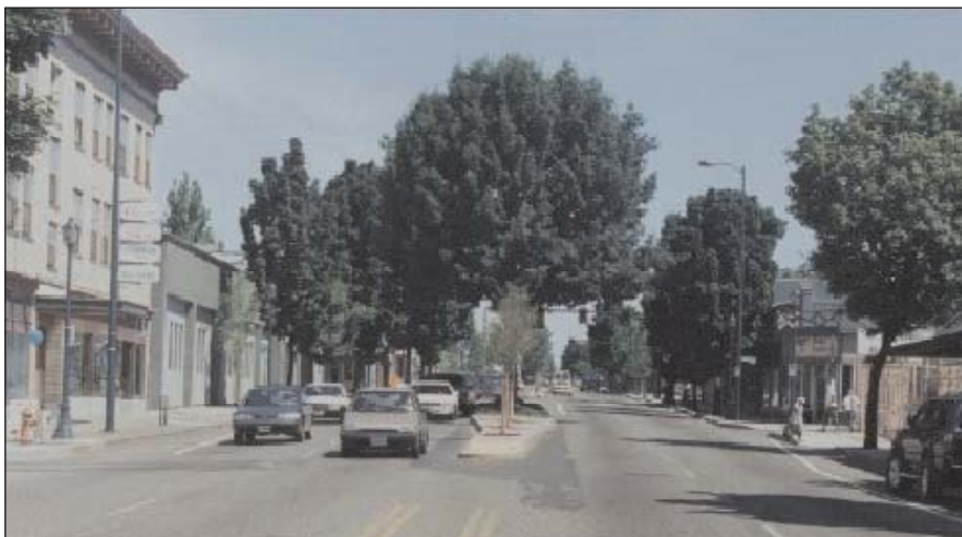
Figure 5. Martin Luther King Boulevard (State Highway 99) in Portland, Oregon, was a major state highway; it has been modified to four lanes with curb parking, landscaped median, and sidewalk landscaping in keeping with its new use as a local arterial.
