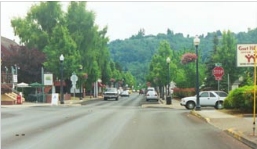
Figure 3. Main Street, downtown Gresham, Oregon; principal commercial section of Main Street converted from four-lane street with parking and narrow sidewalks (foreground) to two lanes with parking and sidewalks widened to accommodate more pedestrians and sidewalk amenities (background).
