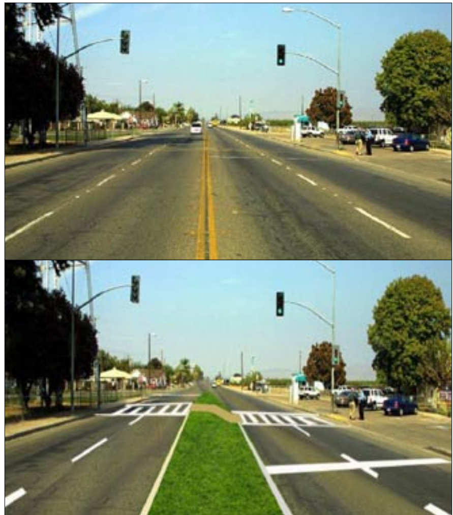
Figure 2. California State Route 63 in Orosi, before and after (simulated). Z-crosswalk and median added to improve safety and aesthetics.
