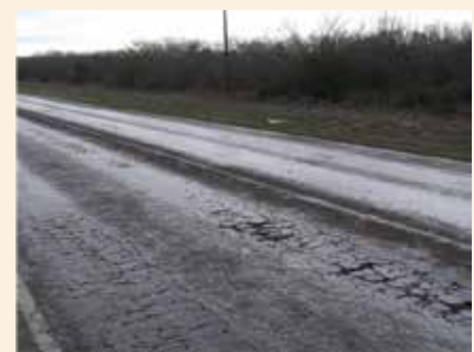
Figure 1. Fatigue Cracking.
