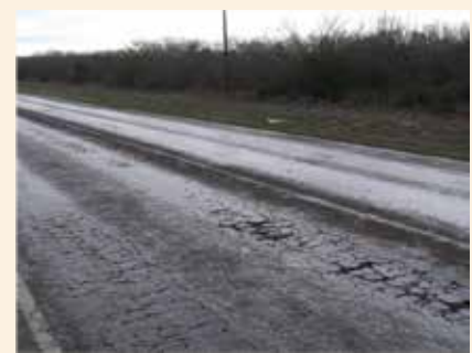
Figure 1. Fatigue Cracking.
