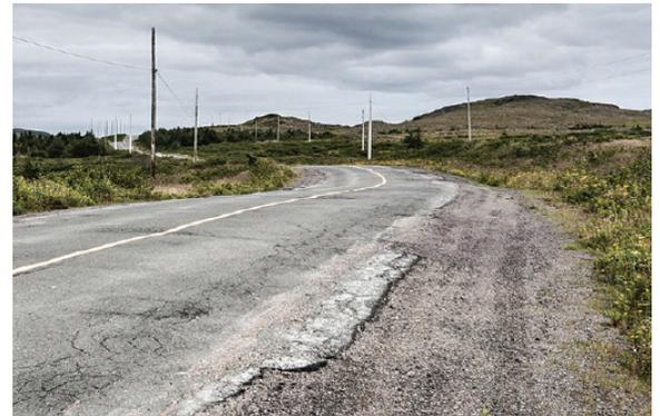
*A shoulder exhibiting signs of degradation due to traffic loads.*
