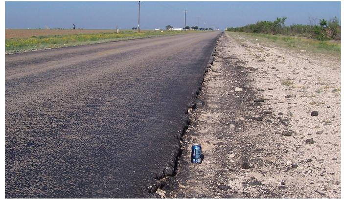
The photo above shows a dangerous failure at the edge of the pavement.
