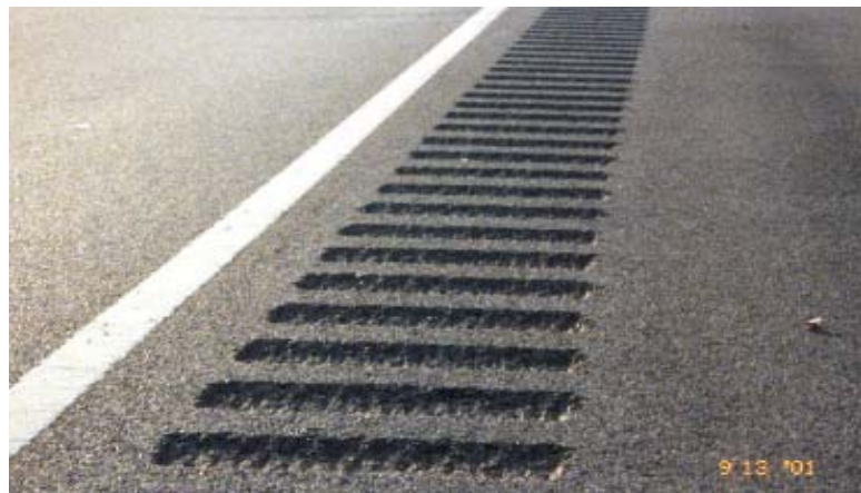
Figure 7-17. Close-Up of Edge Line Rumble Strips.
