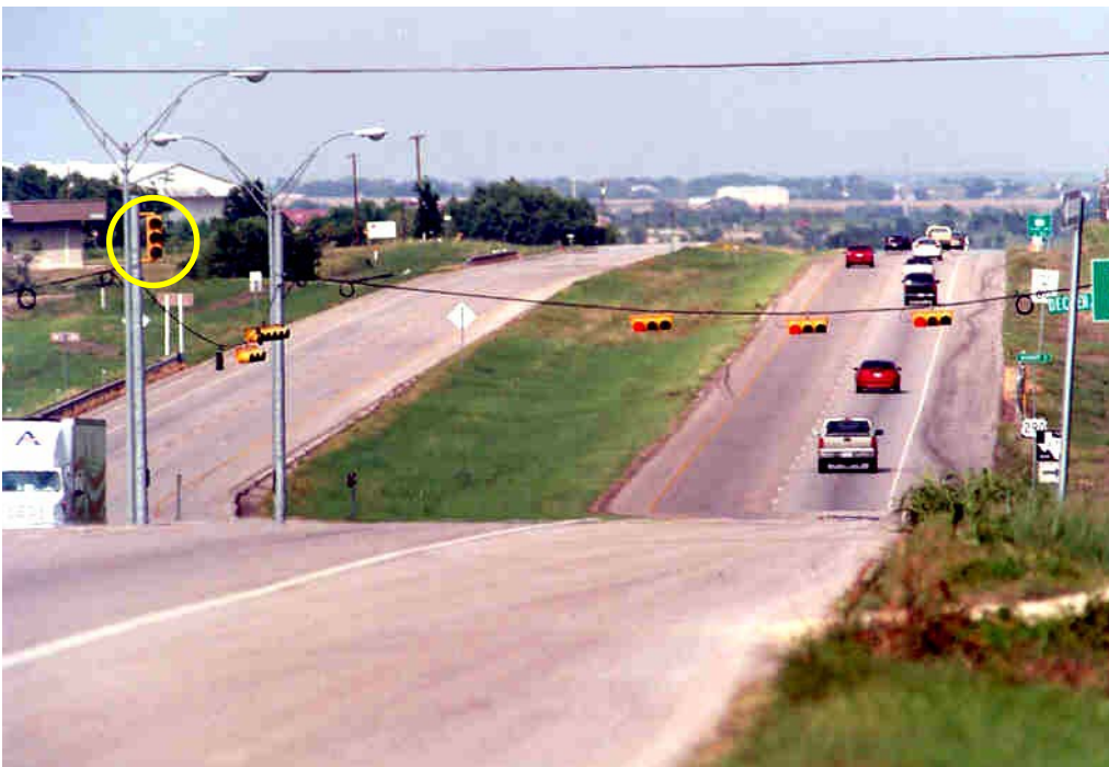
(b) Traffic Signal More Visible Beyond Crest.
