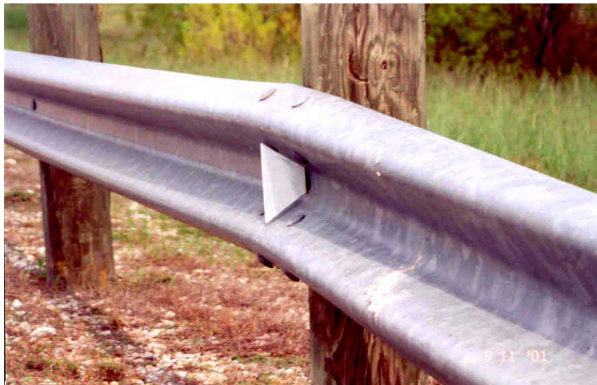
Figure 5-26. Reflector Installed in Guardrail.
