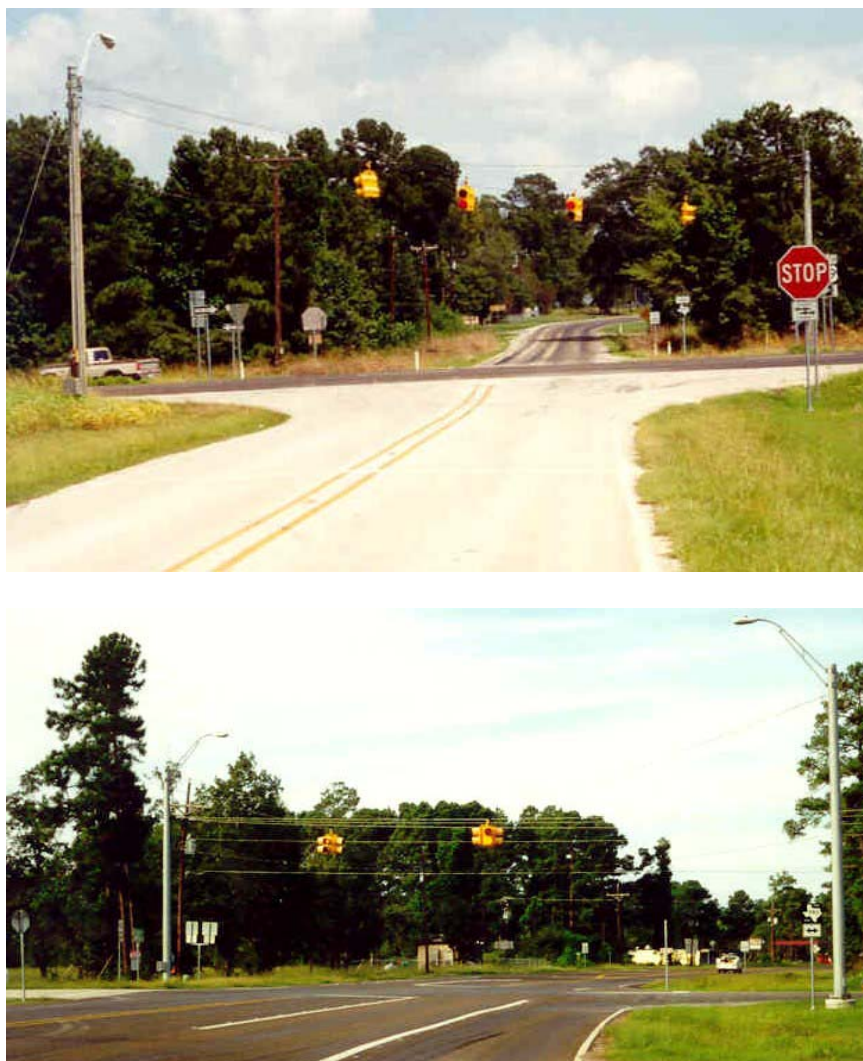
Figure 6-11. Examples of Intersections with Flashing Beacons.
