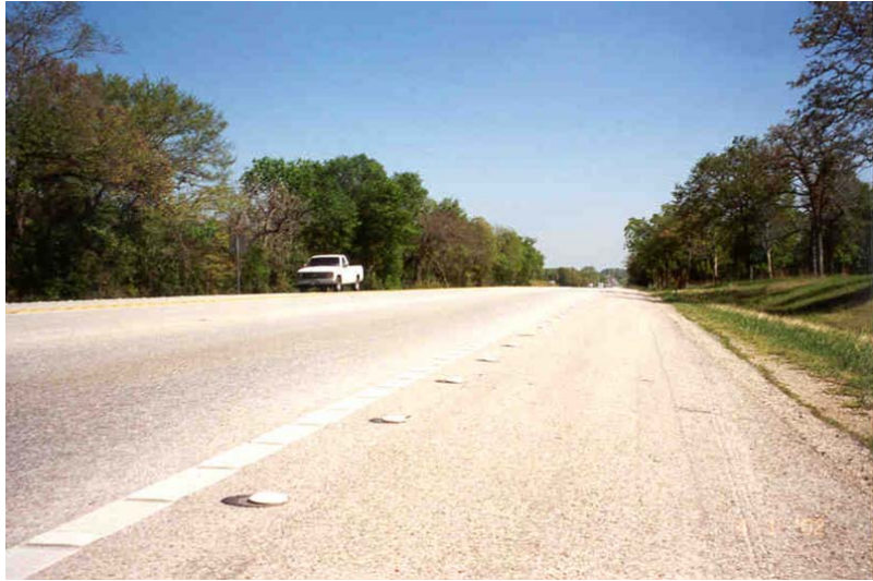
Figure 7-34. Shoulder Texturing with Traffic Buttons.
