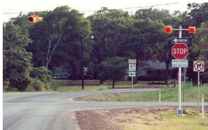
Figure 7-41. Another View of the Intersection of Villa Maria and SH 47.
