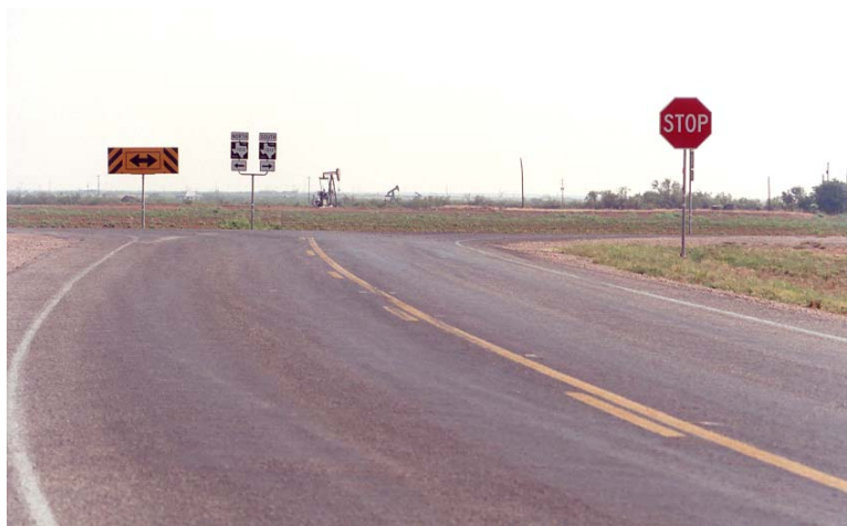
Figure 7-9. New Roadway Intersection.
