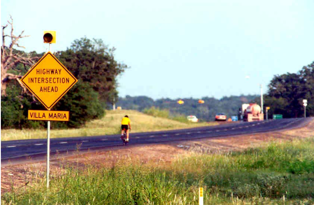
Figure 7-45. Solar-Powered Flashers on Intersection Warning Sign.
