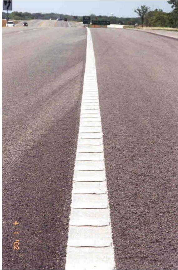
Figure 7-36. Edge Line Profile Markings.
