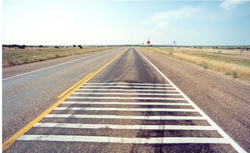
Figure 7-21. Rumble Strips Preceding Flasher and Sign on US 62/82.
