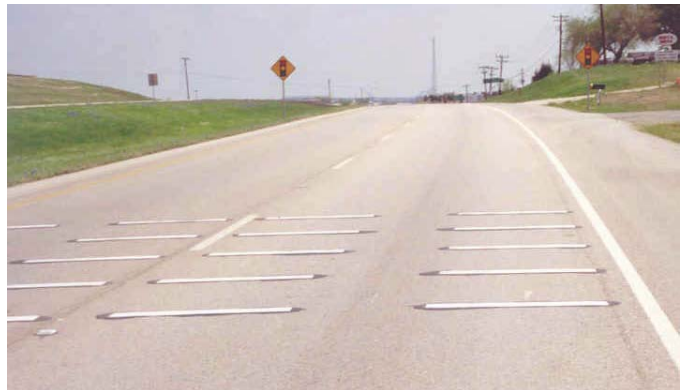
Figure 7-37. Rumble Strips and Warning Signs on an Approach to Signal Just Beyond Crest of Vertical Curve.
