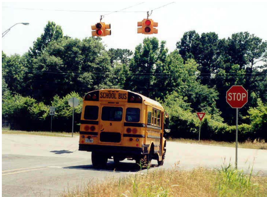
Figure 6-10. Intersection Flashing Beacons.
