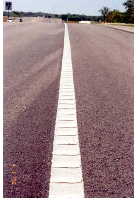
Figure 5-2. Examples of Thermoplastic Profile Markings.
