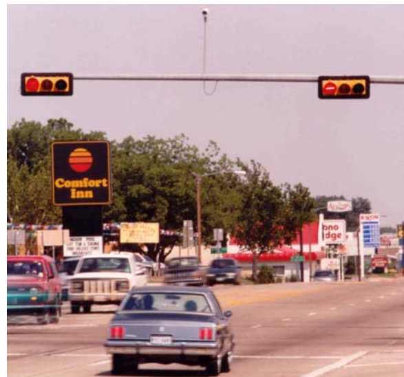
Figure 6-14. Strobe-Enhanced Signal Heads.
