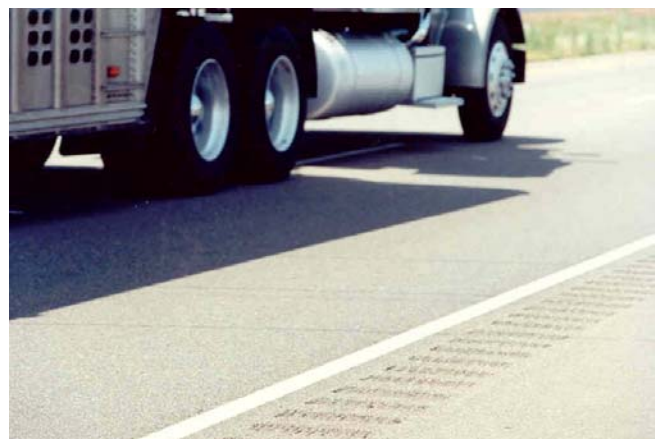
Figure 5-1. Example of Edge Line Rumble Strips (2).
