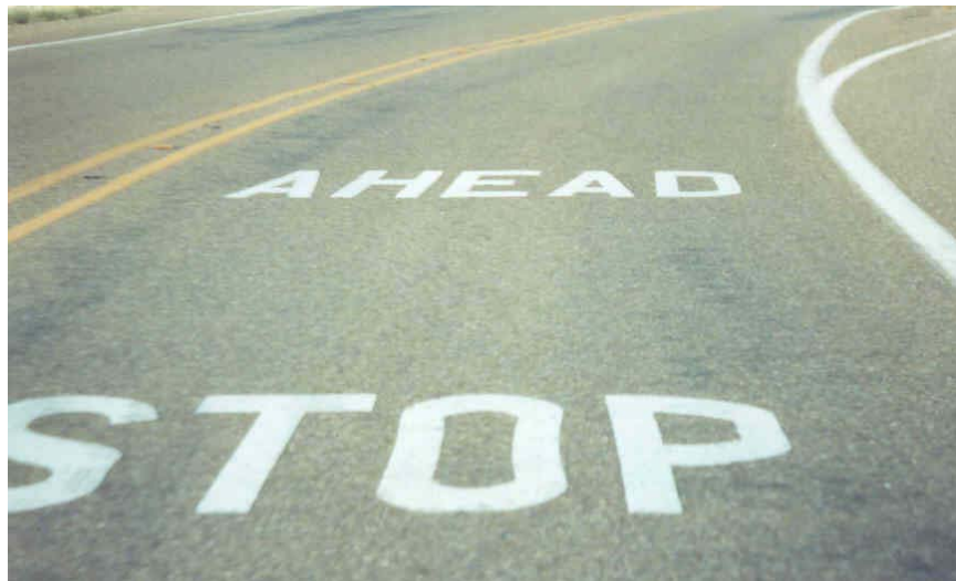
Figure 7-22. "Stop Ahead" Pavement Marking on US 62/82.
