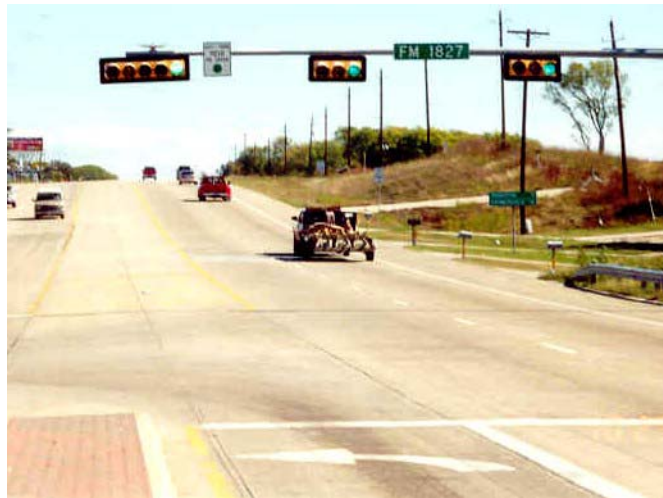
Figure 6-16. Backplates at Local Intersection.
