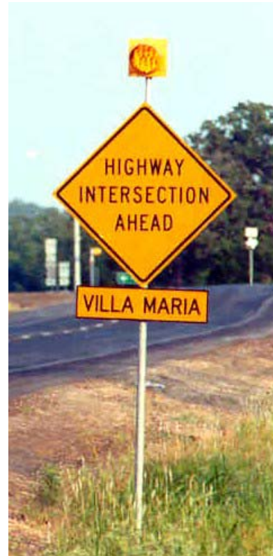
Figure 6-3. Example of Flasher on Advance Intersection Sign.
