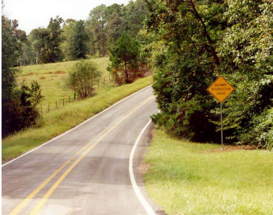
Figure 5-12. Example of Centerline and Edge Line Pavement Markings.
