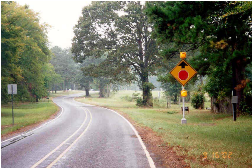
Figure 6-4. Example of Flasher on a Stop Ahead Sign.
