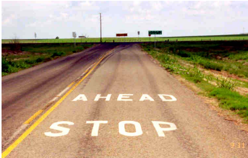
Figure 6-2. Example of Advance Warning Pavement Markings.
