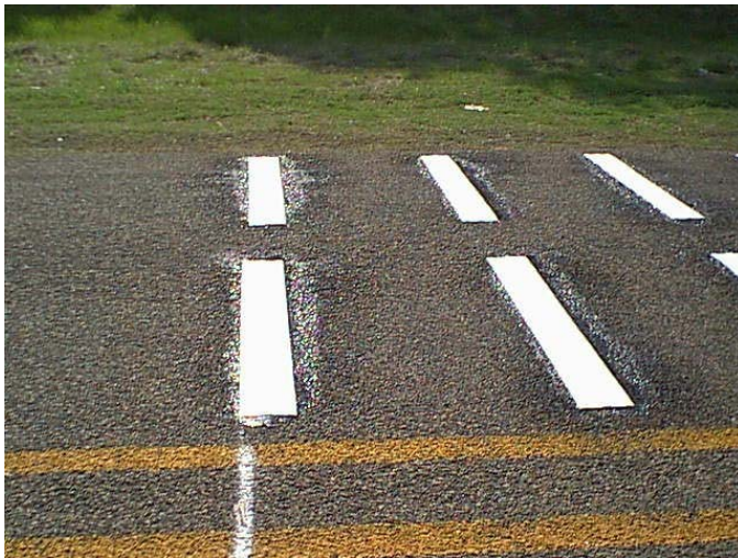
Figure 7-25. Recently Replaced Rumble Strips.
