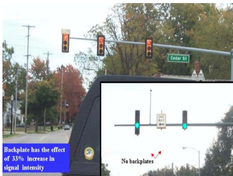
Figure 6-15. Heads with and without Backplates (111).
