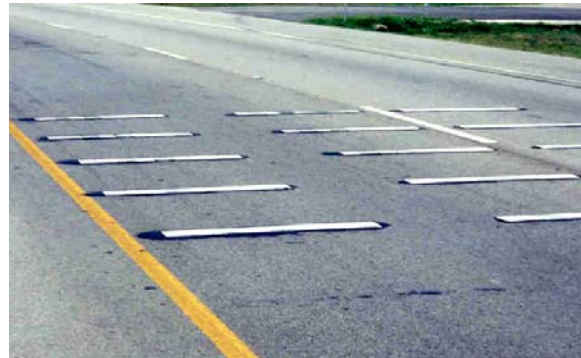
Figure 6-7. Application of Partial-Width Approach Rumble Strips.
