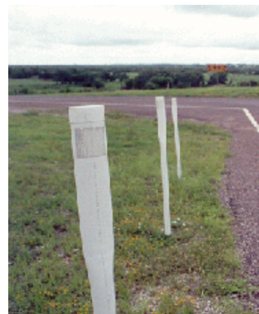
Figure 5-24. Example of Post-Mounted Delineator.
