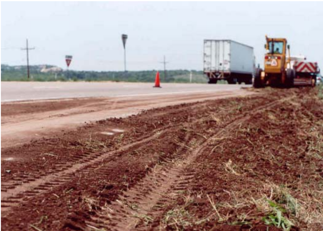
Figure 7-31. Motor Grader Adding Fill Material to Shoulder.
