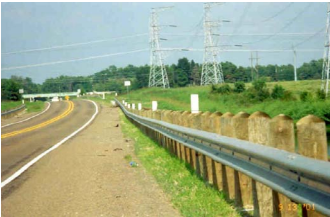
Figure 5-25. Post-Mounted Delineators with a Guard Rail.
