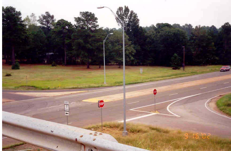
Figure 6-18. Example of Lighting at Complex Intersection.
