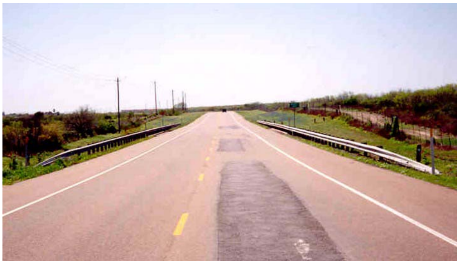
Figure 7-2. Guardrails on SH 16, North of Hebbronville.
