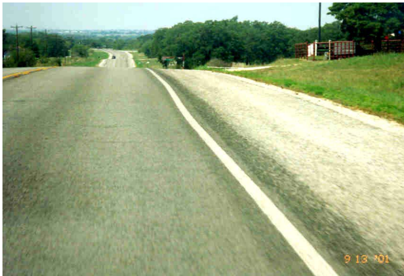
Figure 7-18. Shoulder Treatment on FM 3002.
