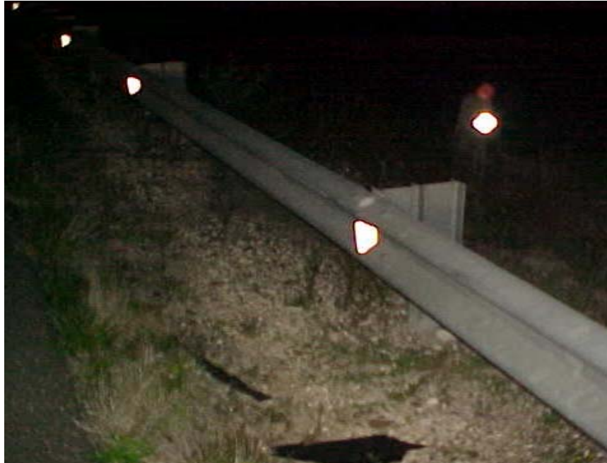
Figure 7-3. Barrier Reflectors on SH 16 at Night.
