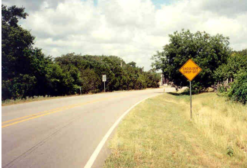
Figure 5-14. Mowed Area on an Inclined Shoulder.
