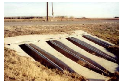
Figure 5-20. Example of a Culvert.
