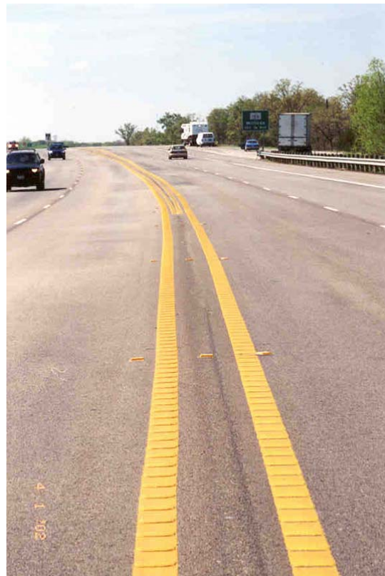
Figure 7-35. Centerline Profile Markings.
