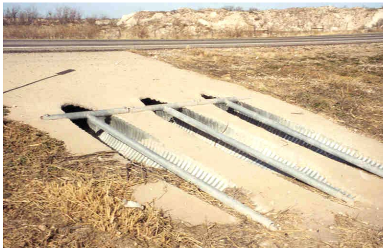
Figure 7-10. New Safety End Treatment on FM 1212.
