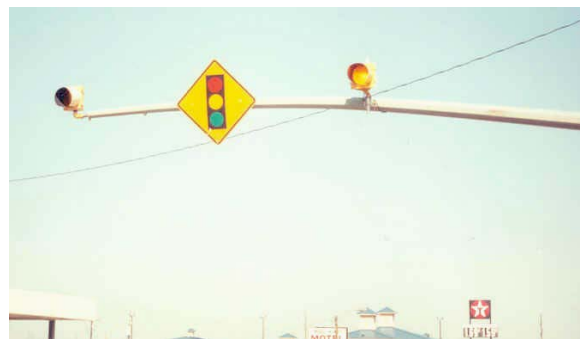
Figure 6-1. Example of Overhead Advance Signing.
