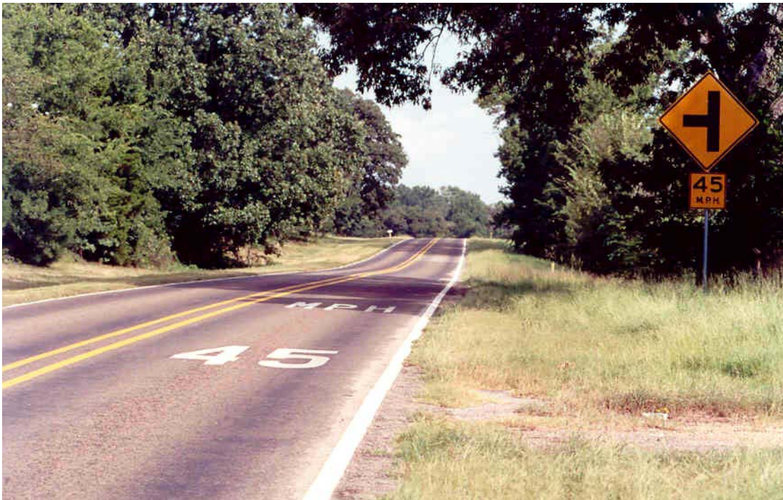
Figure 7-13. Pavement Markings Supplementing Advisory Speed Sign.
