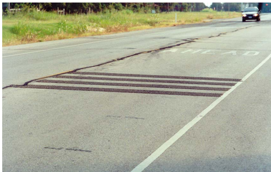
Figure 7-43. Rumble Strips and Pavement Markings on FM 1179.
