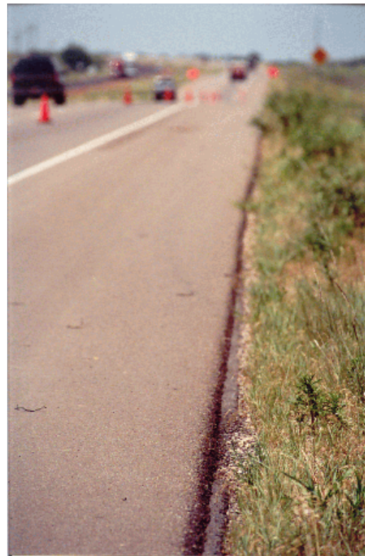
Figure 5-9. Shoulder Drop-Off.
