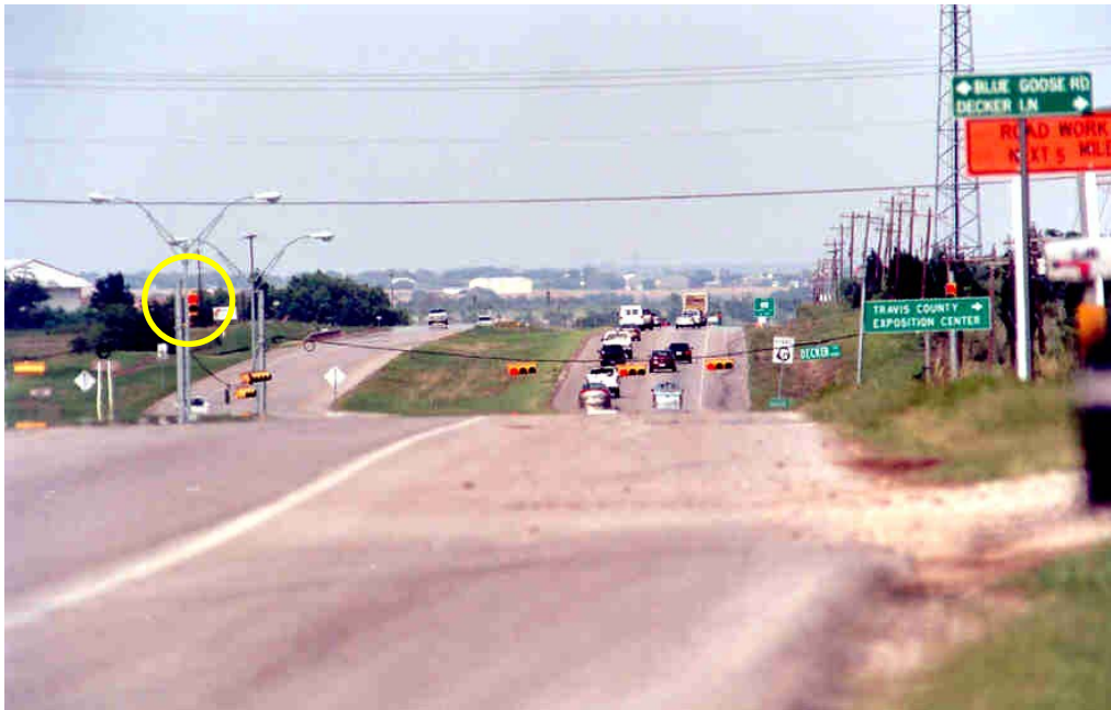
(a) Traffic Signal Just Visible Beyond Crest of Hill.
