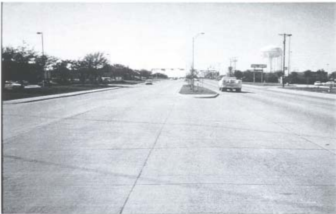
Figure 2-25. Westbound University Drive near Graves Street.
