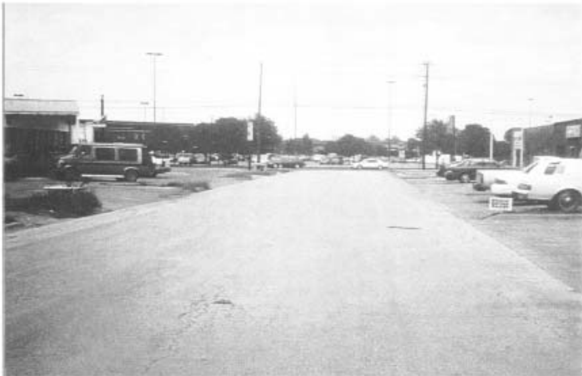
Figure 2-32. Northbound Faith Road near Call Field Road.
