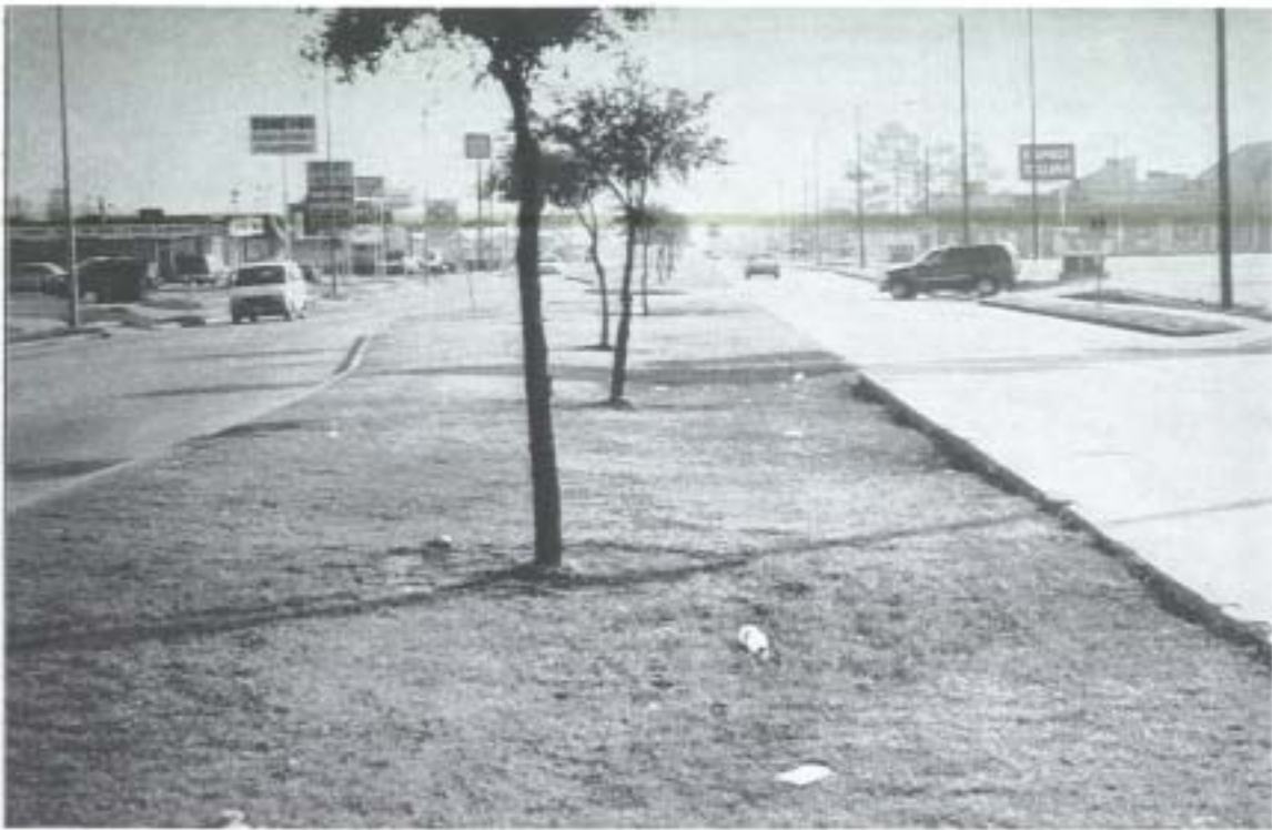
Figure 2-13. Eastbound West Fuqua Road at Hiram Clarke Road.
