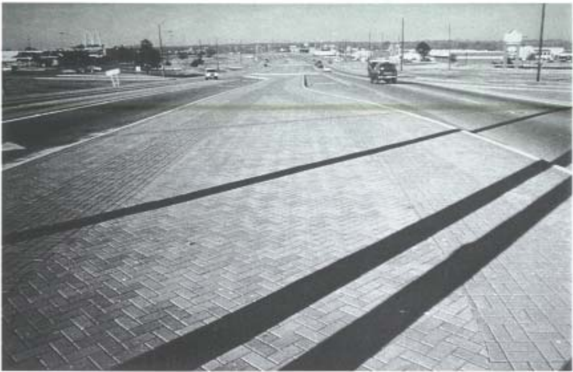
Figure 2-26. Westbound Loop 281 near Judson Road.
