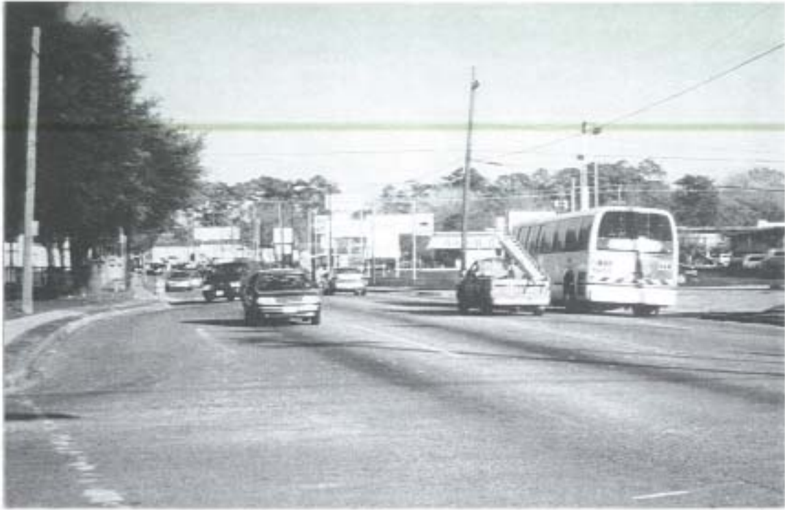
Figure 2-18. Eastbound Long Point Road at Campbell Road.
