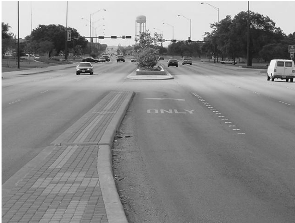
Figure 2-1. Median Treatment along Texas Avenue.
