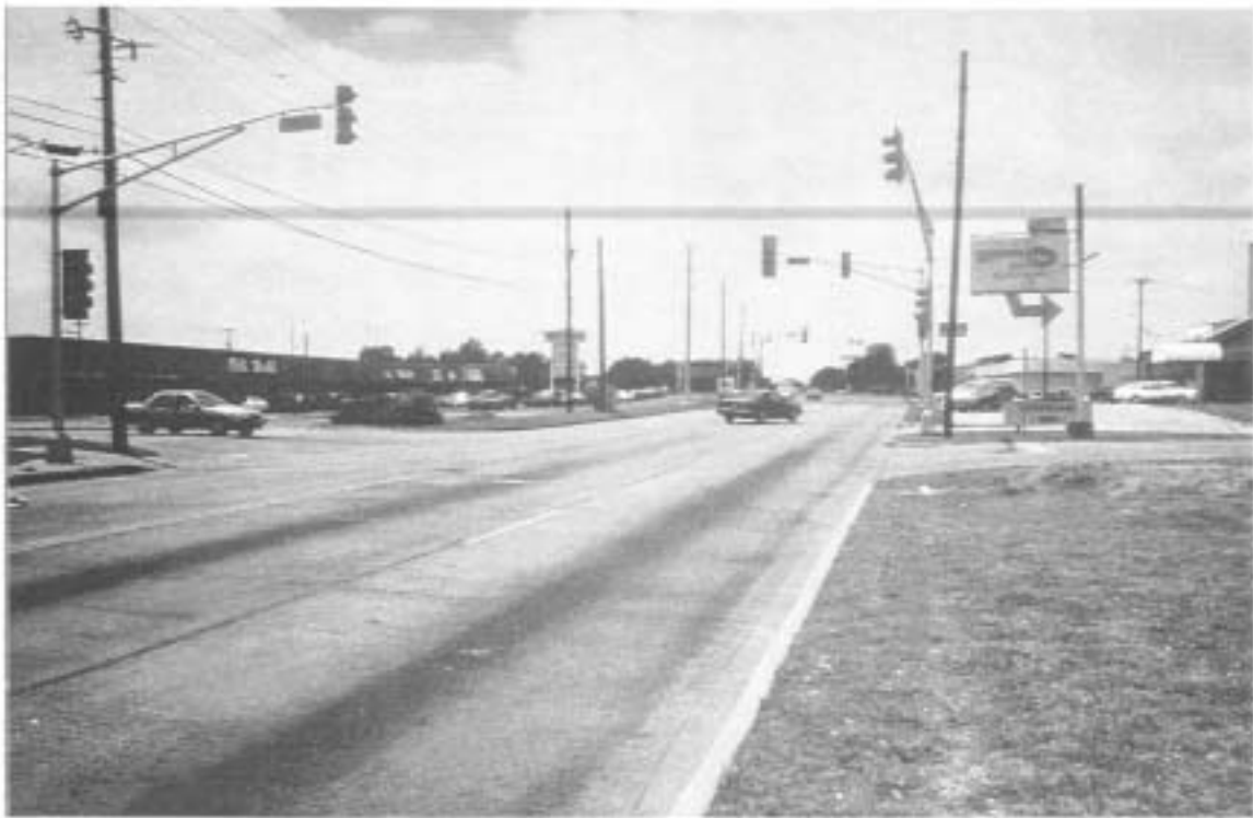
Figure 2-31. Westbound Call Field Road at Rhea Road.
