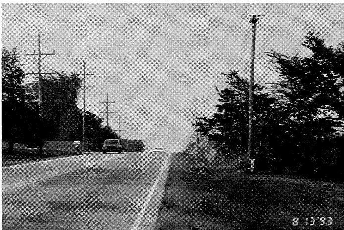
Figure 7. A Crest Vertical Curve.
