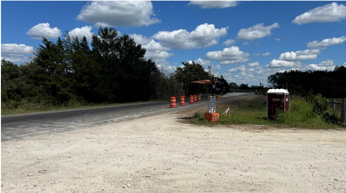
Figure 12. DAD at D1 Looking Southbound.
