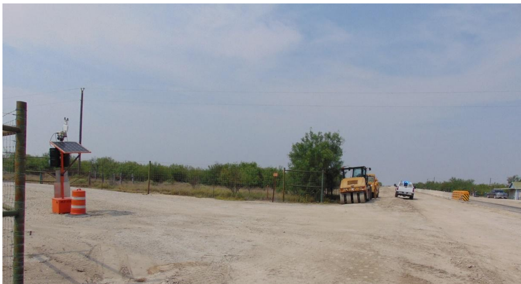
Figure 3. DAD at D9 Looking Westbound.
