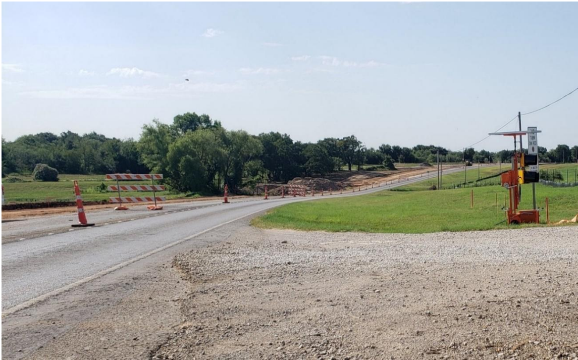
Figure 6. DAD at D21 Looking Southbound.
