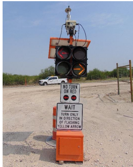
Figure 1. Four-Section Stacked DAD Deployed on FM 2688 at D9.
