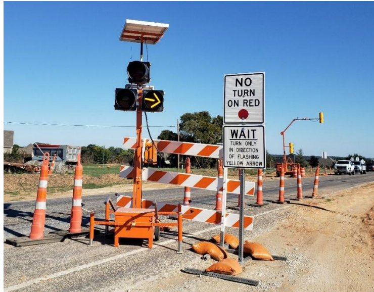
Figure 4. Three-Section Doghouse DAD Deployed on FM 730 at D18.
