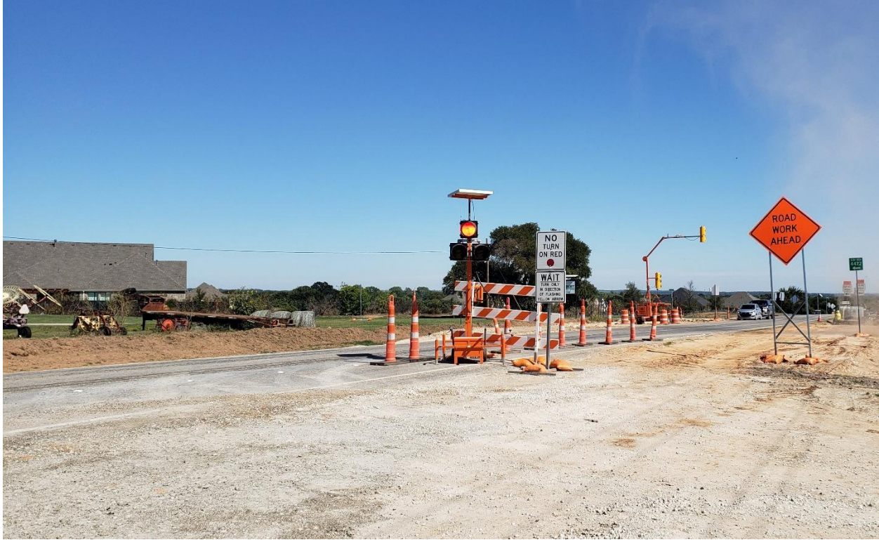
Figure 8. DAD at D18 Looking Southbound.
