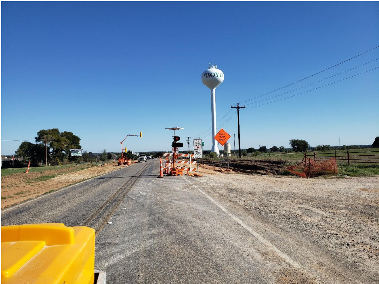
Figure 16. End of Concrete Barrier and DAD at D18 Looking Southbound.
