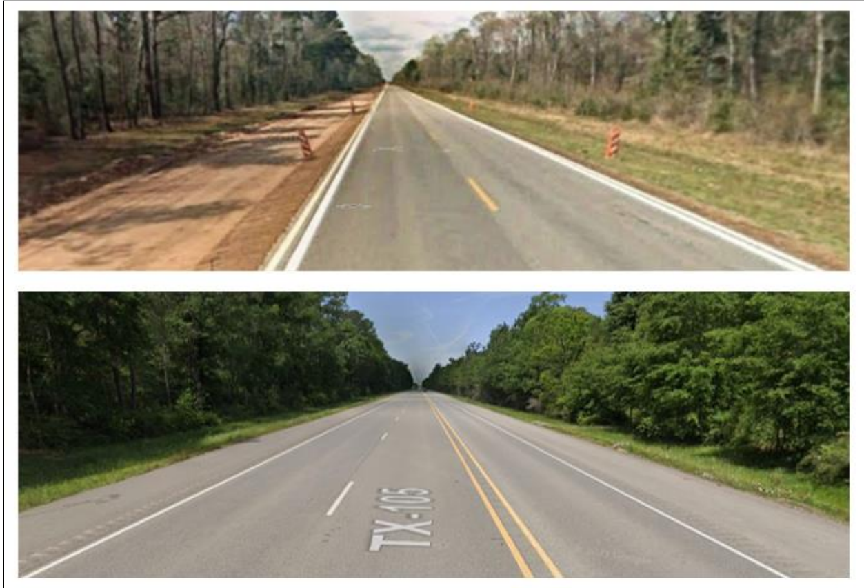
Figure 45. Construction (2008) and Current Pavement (2021), Project 1.
