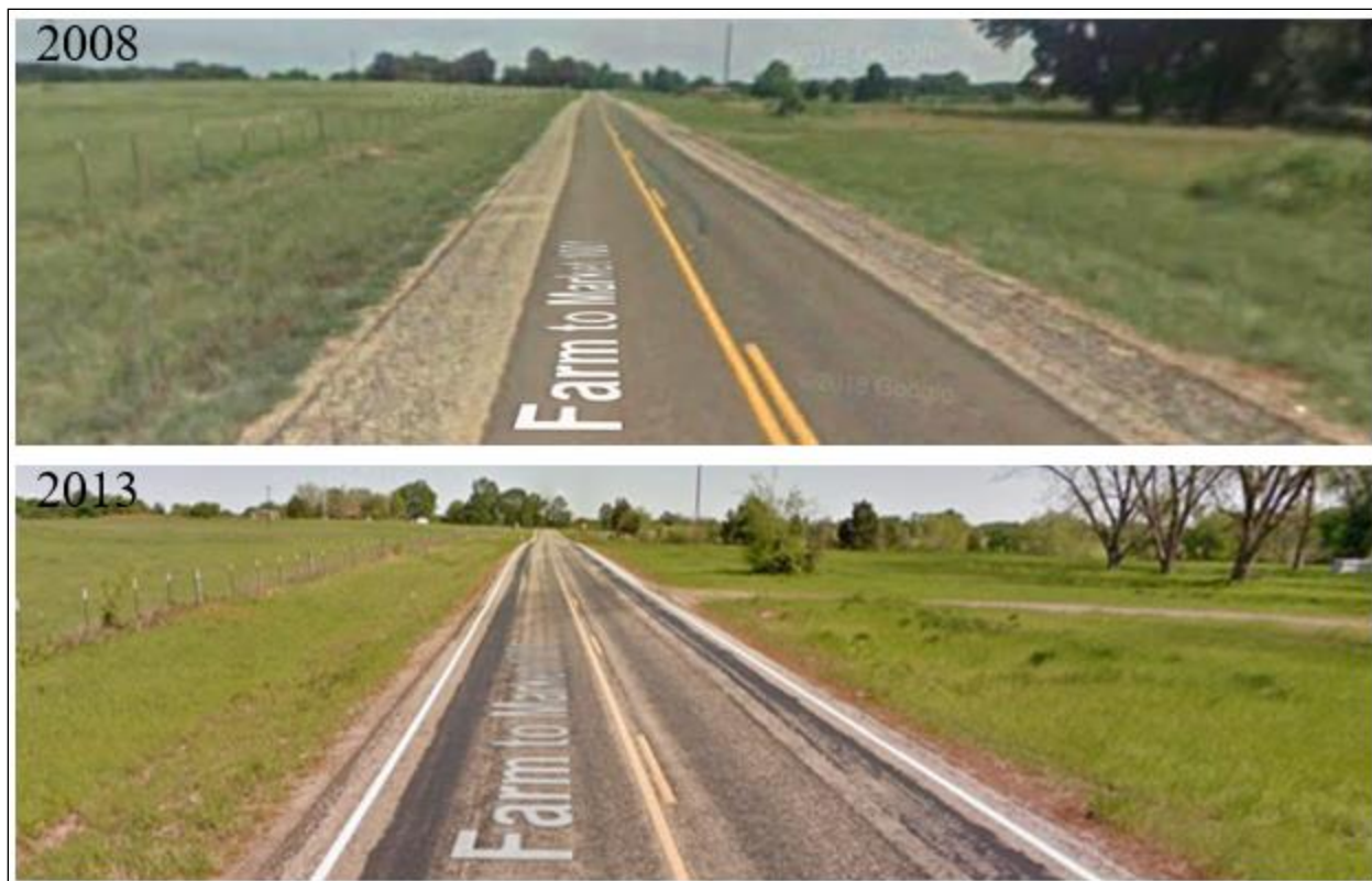
Figure 52. Existing (2008) and Widened Pavement (2013), Project 2.
