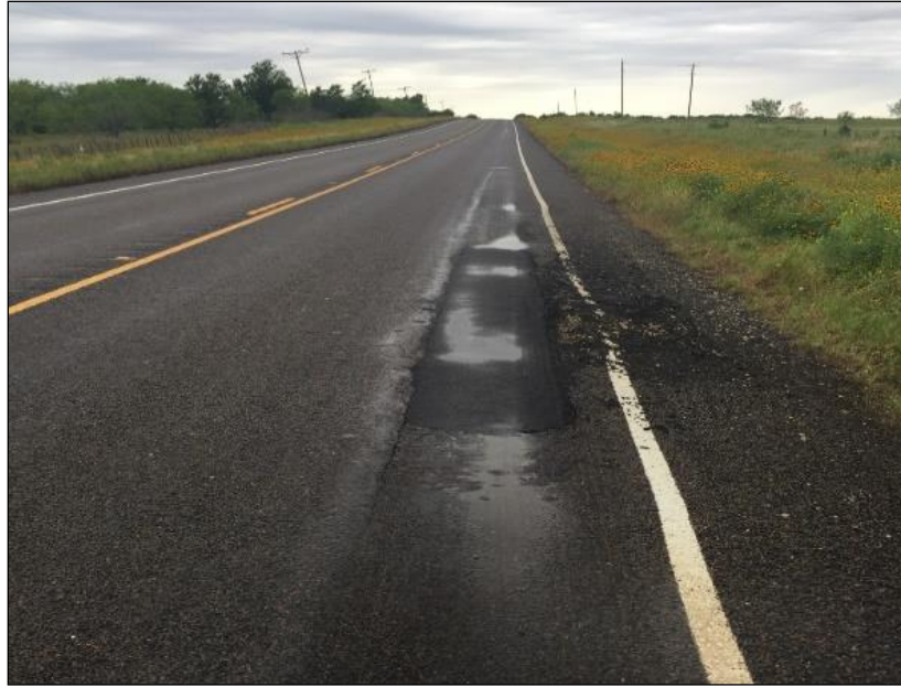
Figure 70. Deflection in Lane versus Shoulder in 2019, Project 4.
