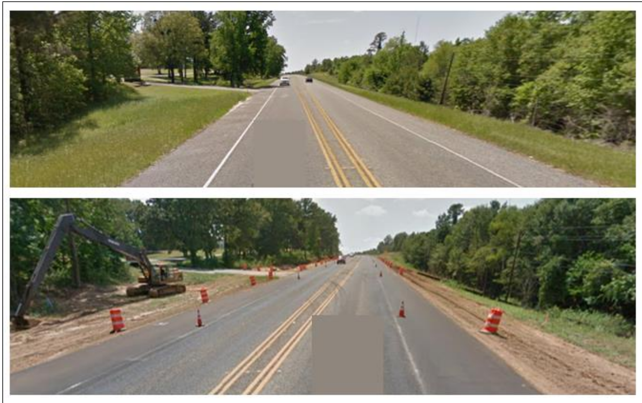
Figure 59. Existing Roadway and during Construction, Project 3.
