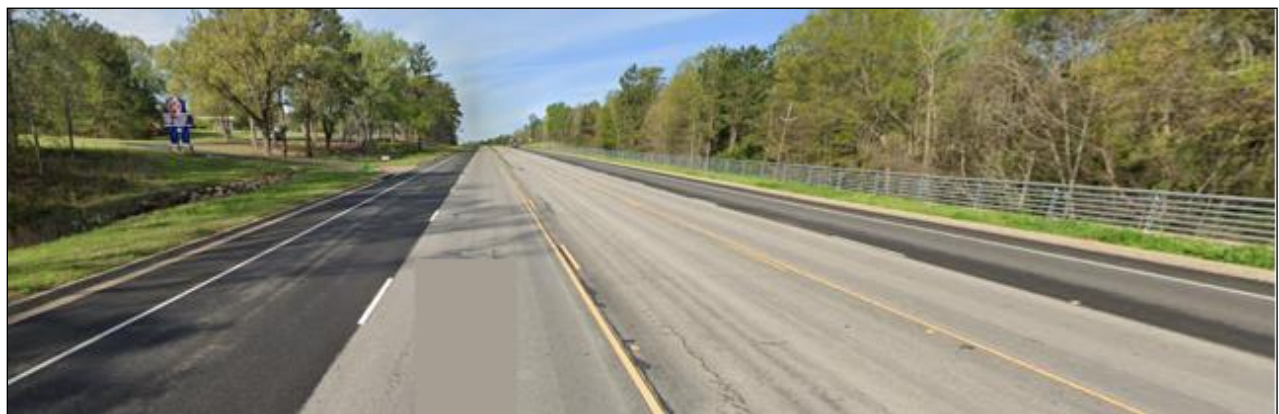
Figure 63. Repaired Outside Widened Lanes, Project 3.
