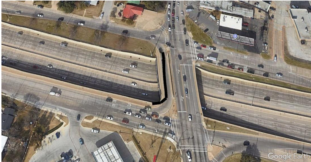
(a) Aerial view of the turnaround bridge at I-20 and McCarter Ave
