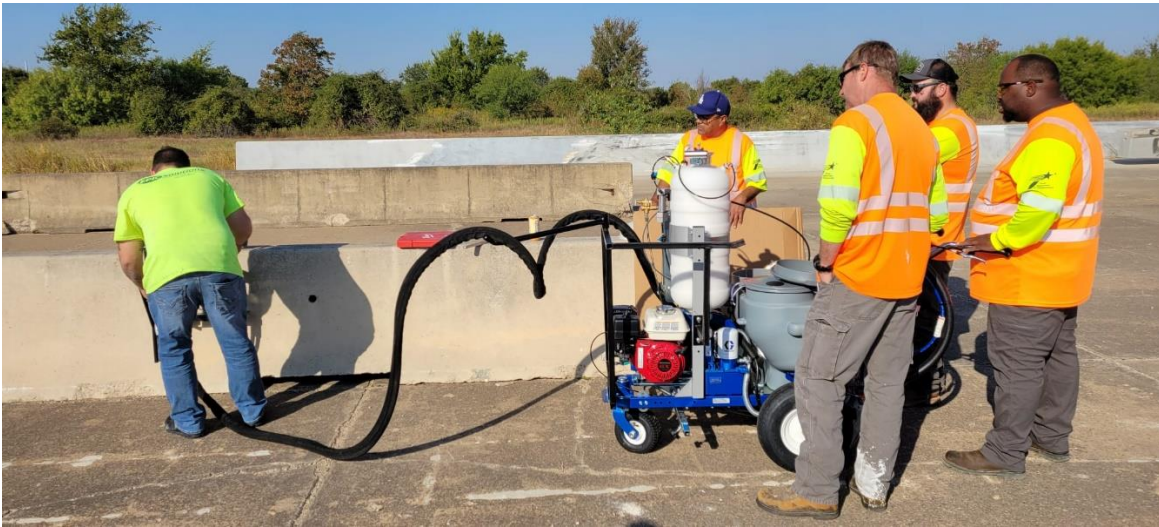
Figure 29. Trainer Illustrating the Use of Barrier Striping Sprayer.
