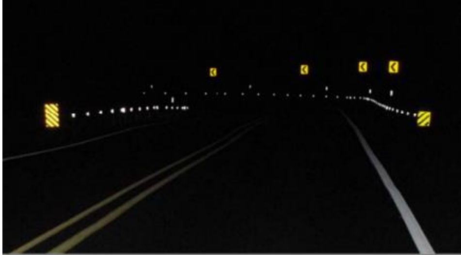
Figure 4. Combination of Delineated Guardrails and Chevrons in Michigan (5).
