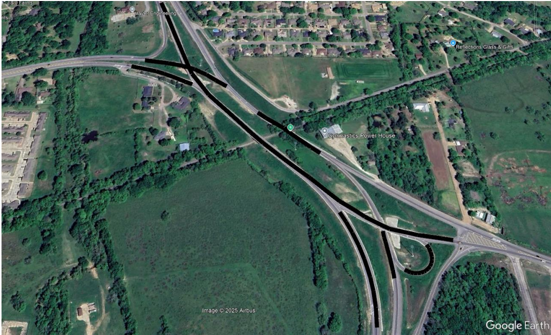
(a) Plan view of the treated sections along SH 286 and US 271 in Paris
