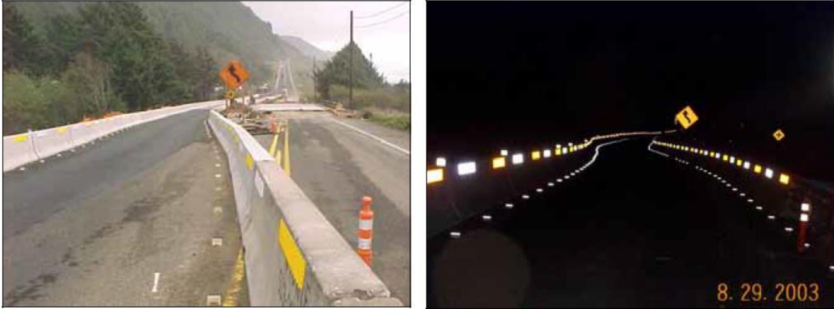
Figure 2. Day and Night Comparison of Bob Creek Bridge (4).
