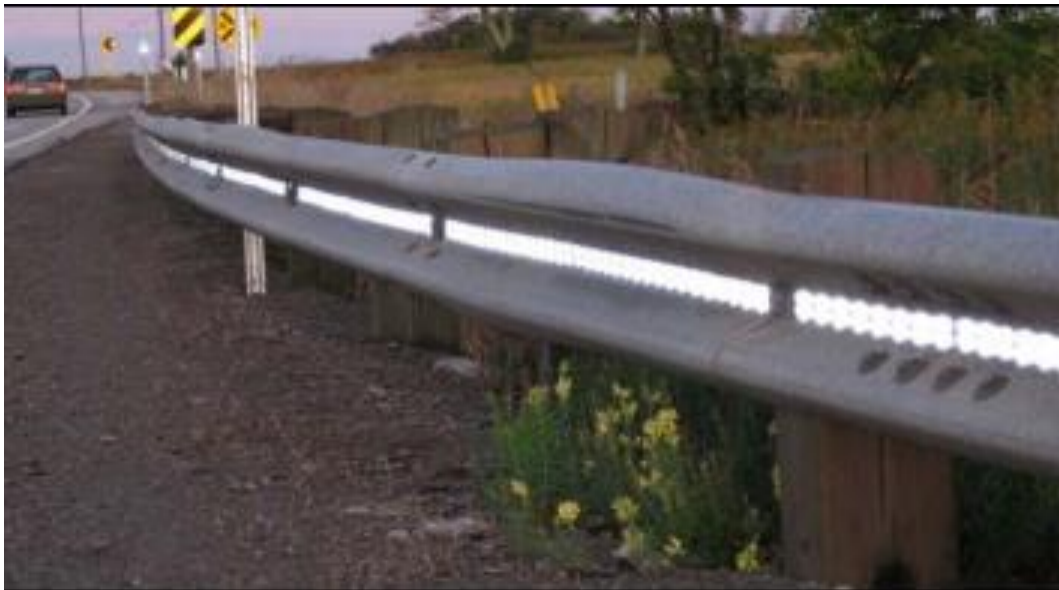
Figure 3. 3M LDS Panels on a Guardrail in Michigan (5).
