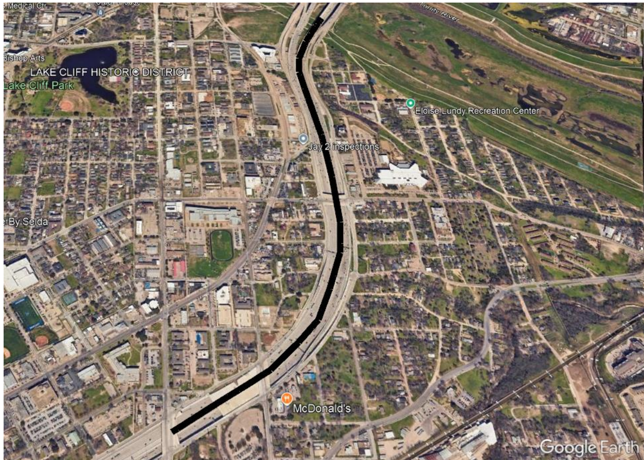
Figure 28. I-35E near S Ewing Ave in Dallas.
