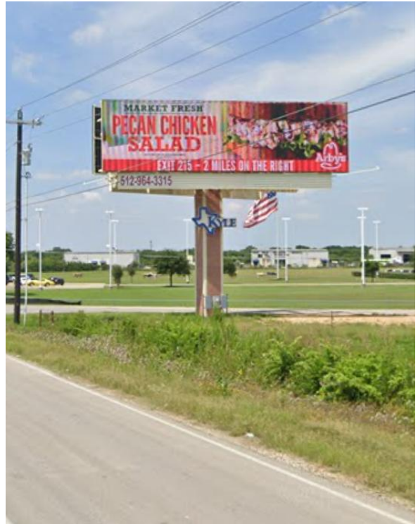
b) After Installation (June 2019)
