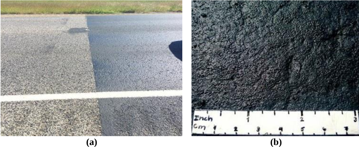
Figure 9. IH 35 in the San Antonio District: (a) beginning of Onyx product application, and (b) surface of the pavement after Onyx application (Scullion et al. 2020).
