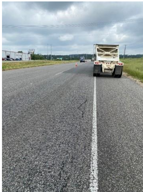
Figure 97. Newer PFC inlaid patch in the travel lane.
