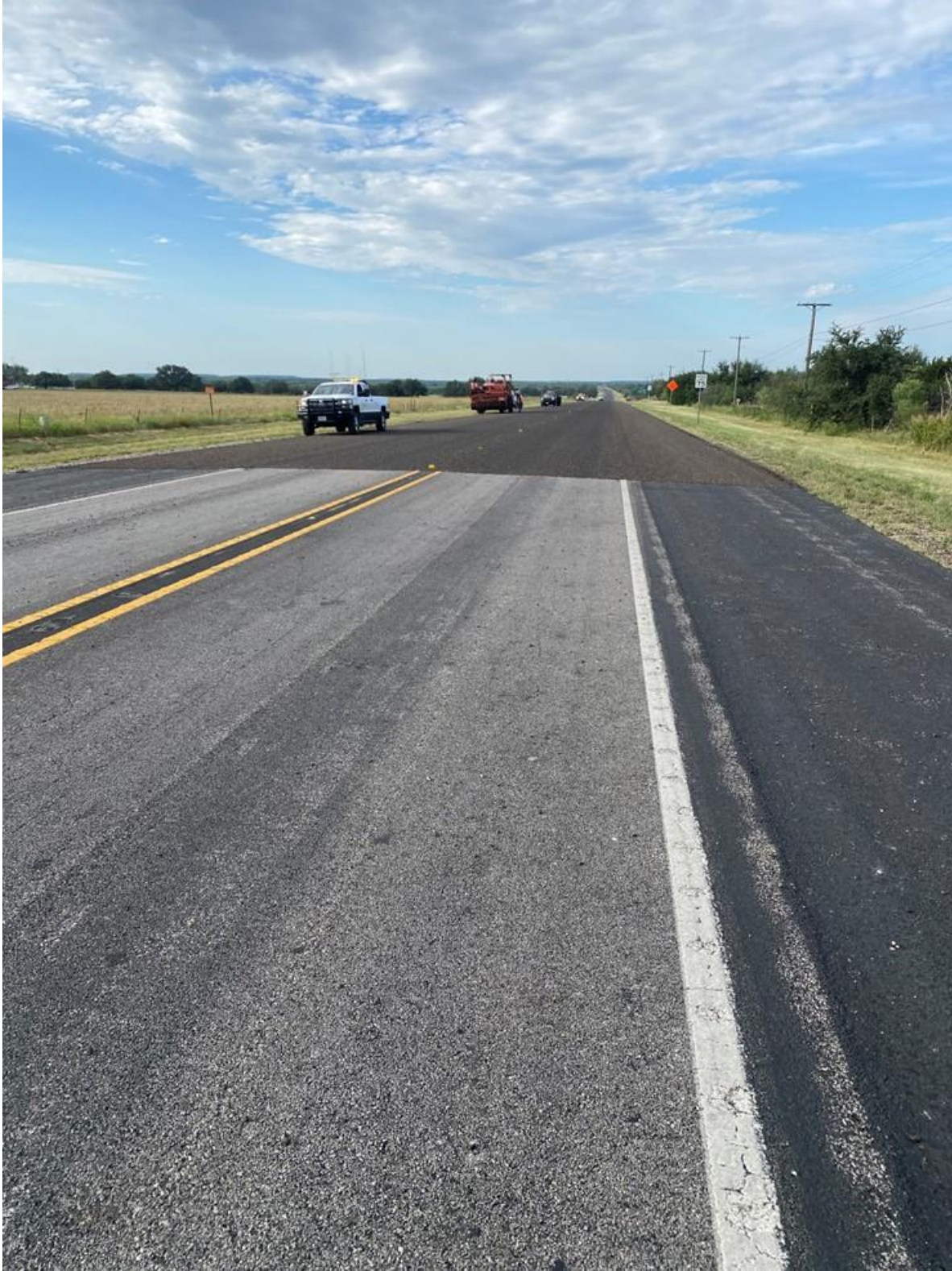
Figure 120. View of seal coat and PFC surface.
