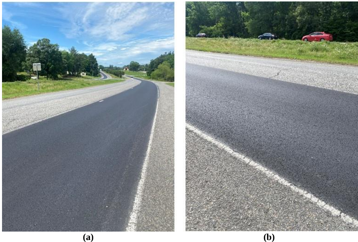
Figure 110. Other portions of the greater contract where old PFCs were milled and inlaid with Superpave C: (a) general view, (b) closeup view.
