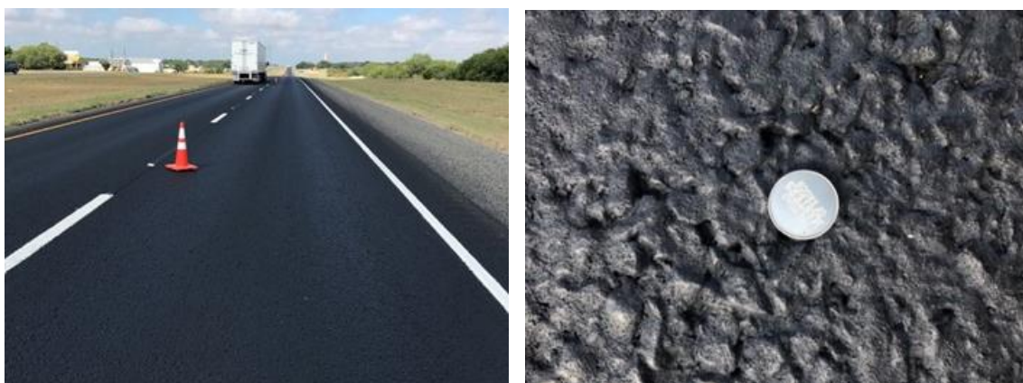
Figure 26. IH 35 PFC surfaced with Onyx.
