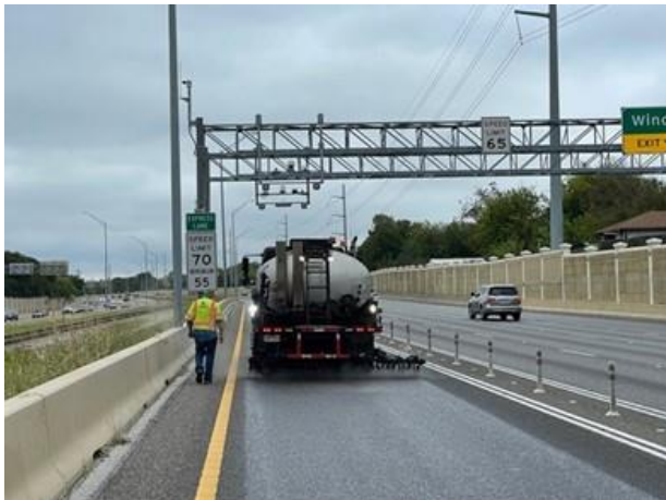
Figure 5. Rejuvenating fog seal application on PFC.
