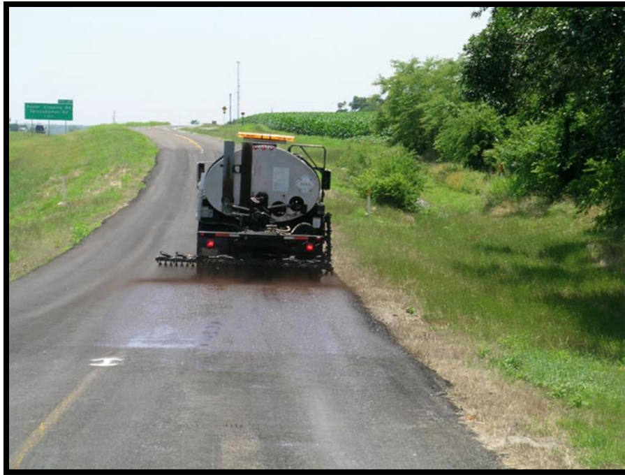
Figure 4. Fog Seal.
