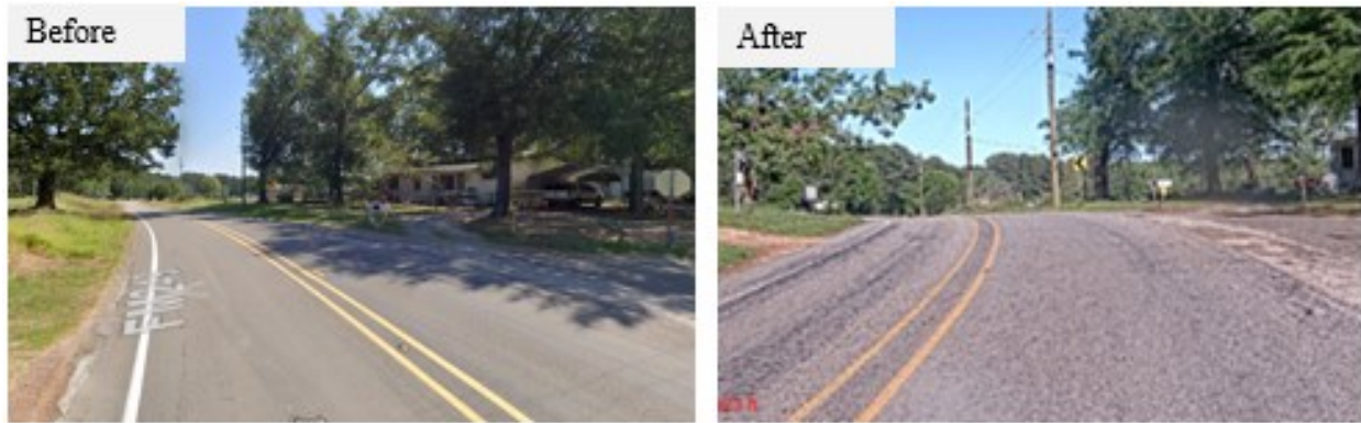
Figure 32. Site 3 Before [9] and After Seal Coat Construction.
