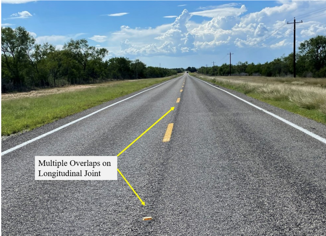
Figure 52. Example of Multiple Seal Coats Overlapping Along a Longitudinal Joint.
