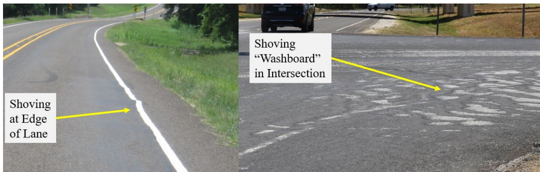
Figure 53. Examples of Shoving at an Edge Line and Intersection.
