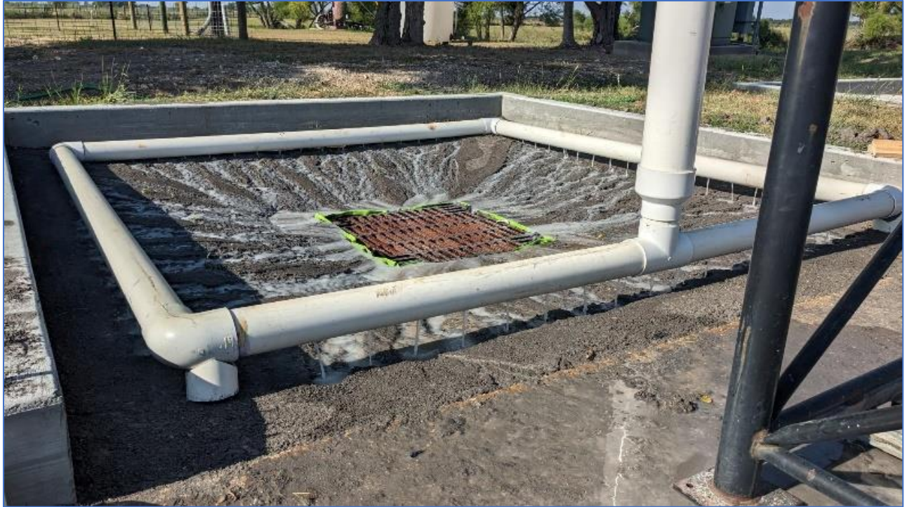
Figure 8. Soil Surface Drop Inlet Evaluation Test System.
