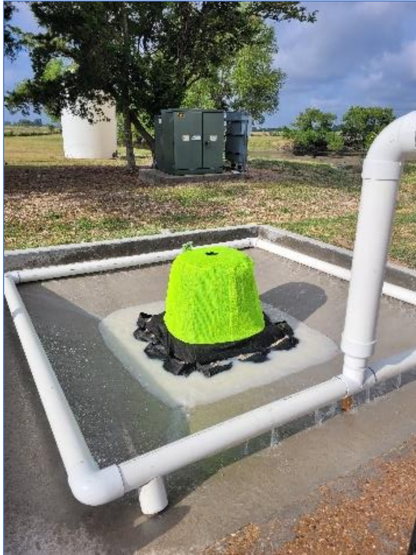
Figure 7. Concrete Drop Inlet Evaluation Test System.
