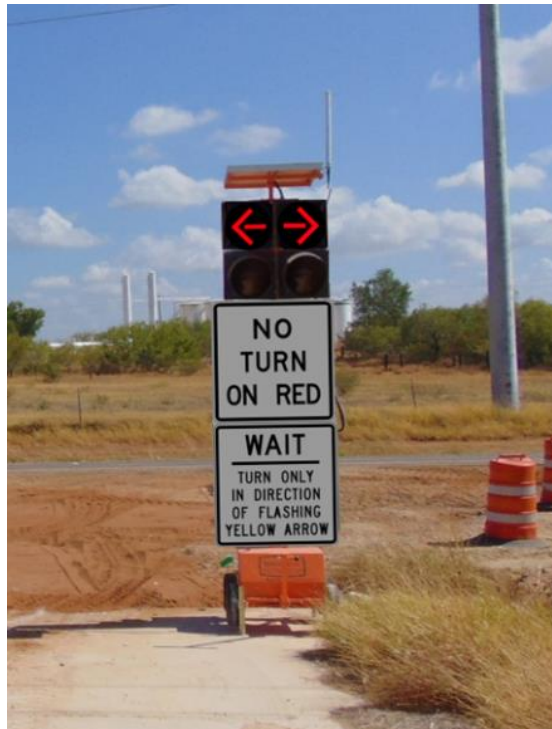
Figure 26. Stop Four-Section Stacked DAD.
