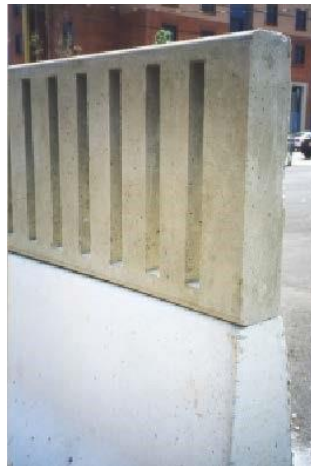
Figure 2.8. Modified Concrete Glare Screen (8).
