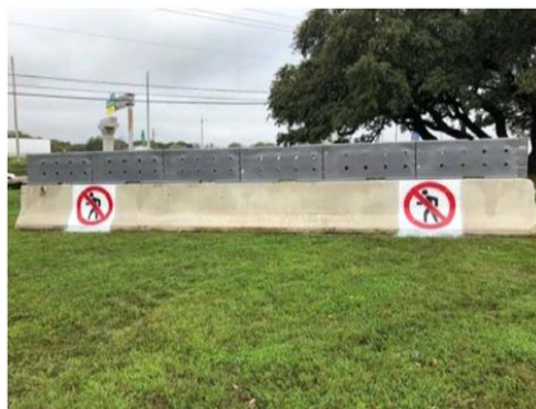
Figure 2.5. Barrier with Sign and Attachment (7).
