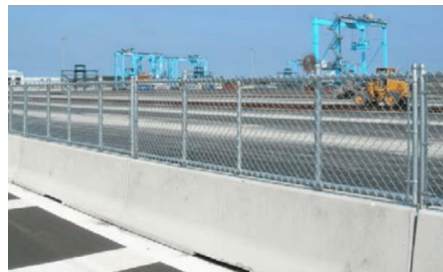
Figure 2.1. Chain-Link System for Concrete Barriers (4).
