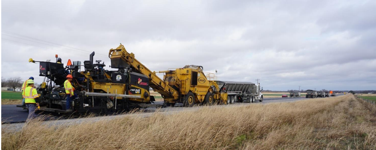
Figure 48. Paving Operation on US 183.
