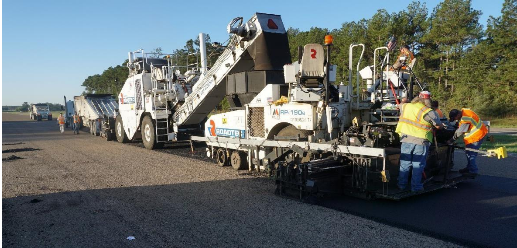
Figure 23. Paving Operation on US 69.
