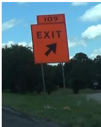
Figure 13. Exit Gore Sign for Exit 109.
