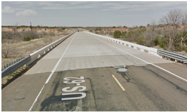
Figure 0.184. Concrete Deck of the Bridge (source: google maps)
