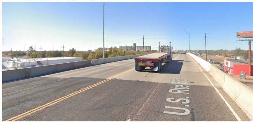
Figure 0.35. Concrete Deck of the Bridge (source: google maps)
