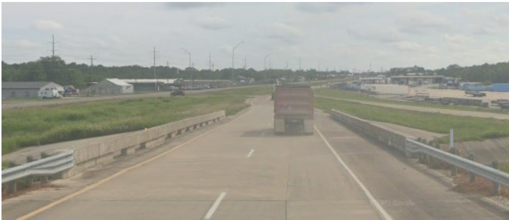
Figure 0.141. Concrete Deck of the Bridge (source: google maps)
