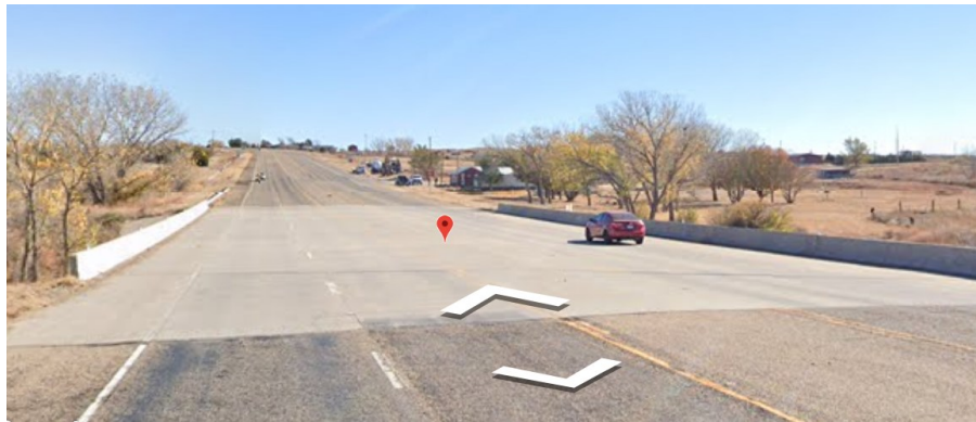
Figure B.9. Concrete Deck of the Bridge (source: google maps)
