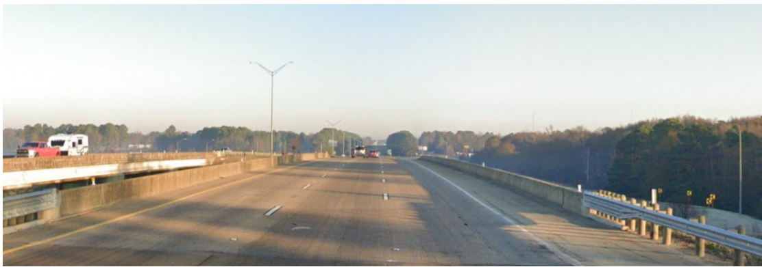
Figure 0.92. Concrete Deck of the Bridge (source: google maps)
