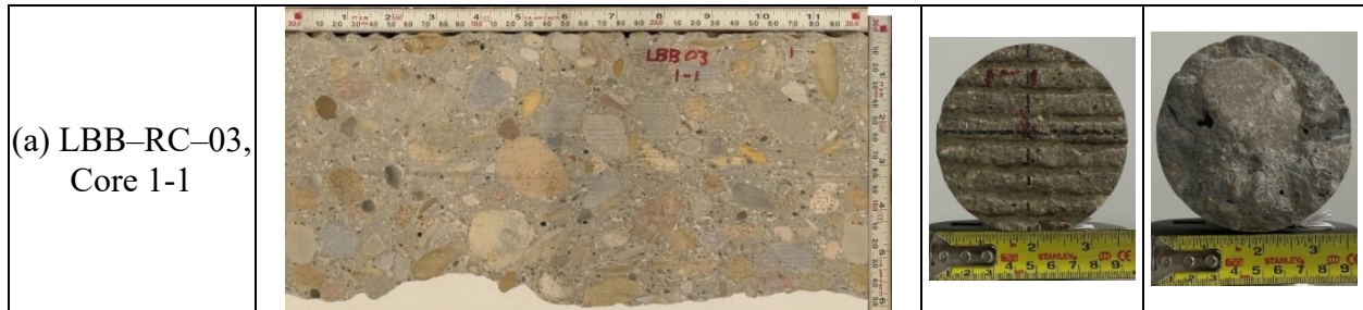
Figure 3.27. Pictures of Core 1-1 of LBB-RC-03 in Good Condition.
