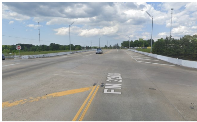
Figure 0.357. Concrete Deck of the Bridge (source: google maps)
