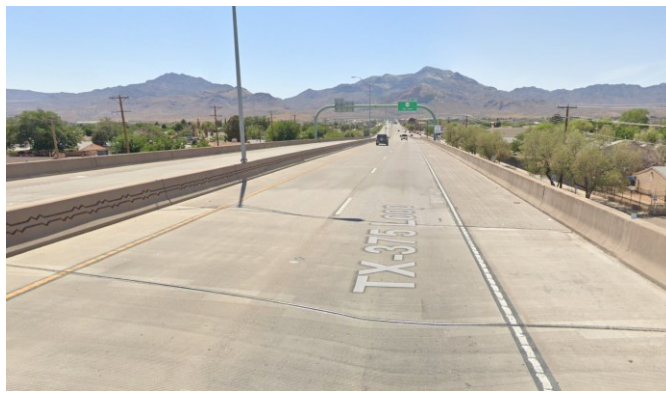
Figure 0.221. Concrete Deck of the Bridge (source: google maps)
