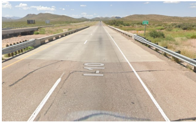
Figure 0.192. Concrete Deck of the Bridge (source: google maps)
