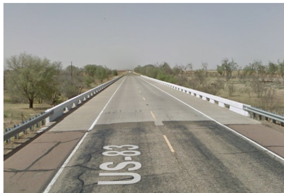
Figure 0.153. Concrete Deck of the Bridge (source: google maps)
