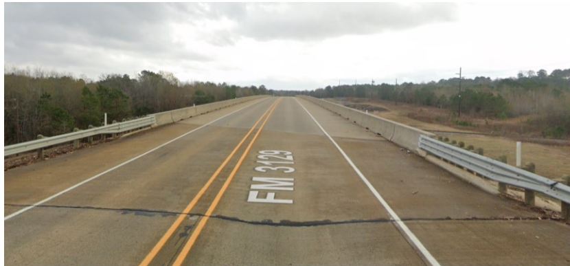
Figure 0.114. Concrete Deck of the Bridge (source: google maps)
