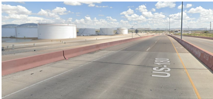
Figure 0.214. Concrete Deck of the Bridge (source: google maps)
