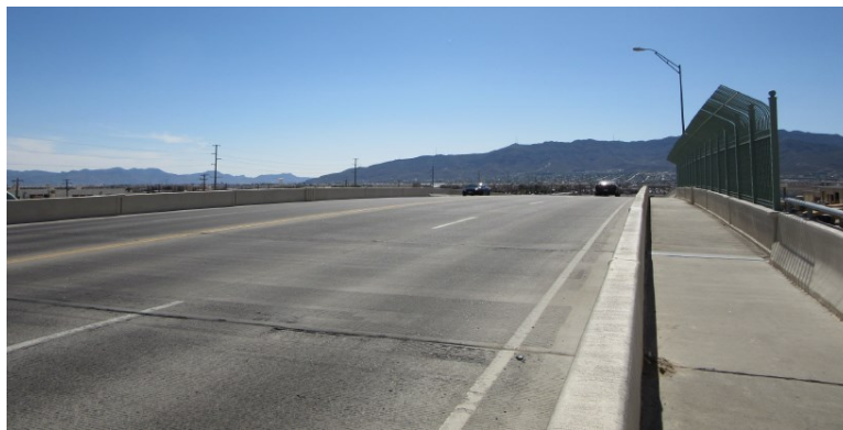
Figure 0.243. Concrete Deck of the Bridge
