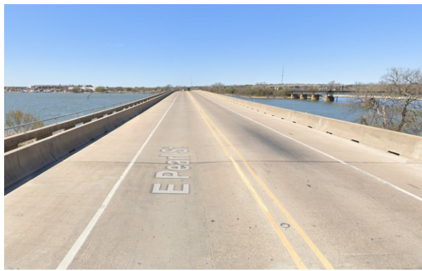
Figure 0.250. Concrete Deck of the Bridge (source: google maps)
