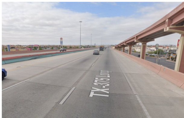
Figure 0.236. Concrete Deck of the Bridge (source: google maps)
