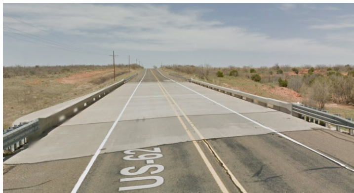
Figure 0.161. Concrete Deck of the Bridge (source: google maps)
