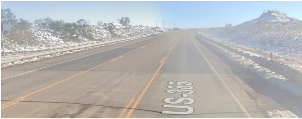
Figure B.21. Concrete Deck of the Bridge (source: google maps)
