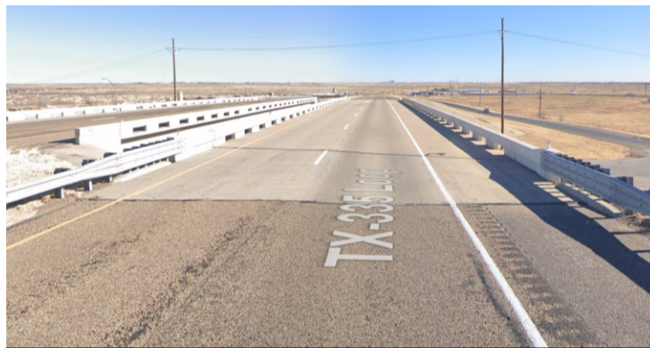
Figure 0.72. Concrete Deck of the Bridge (source: google maps)
