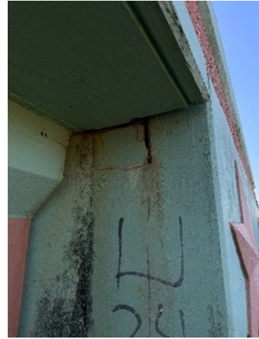
(a) Spalling at abutment wall (TYL-RC-03) (b) Crack at abutment wall (TYL-RC-03)
