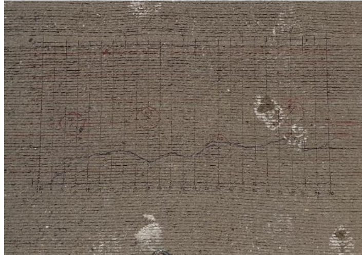
Figure 3.6. Grid on Concrete Deck.
