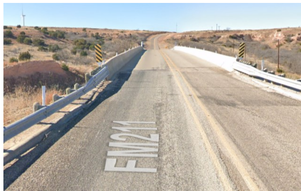
Figure 0.309. Concrete Deck of the Bridge (source: google maps)
