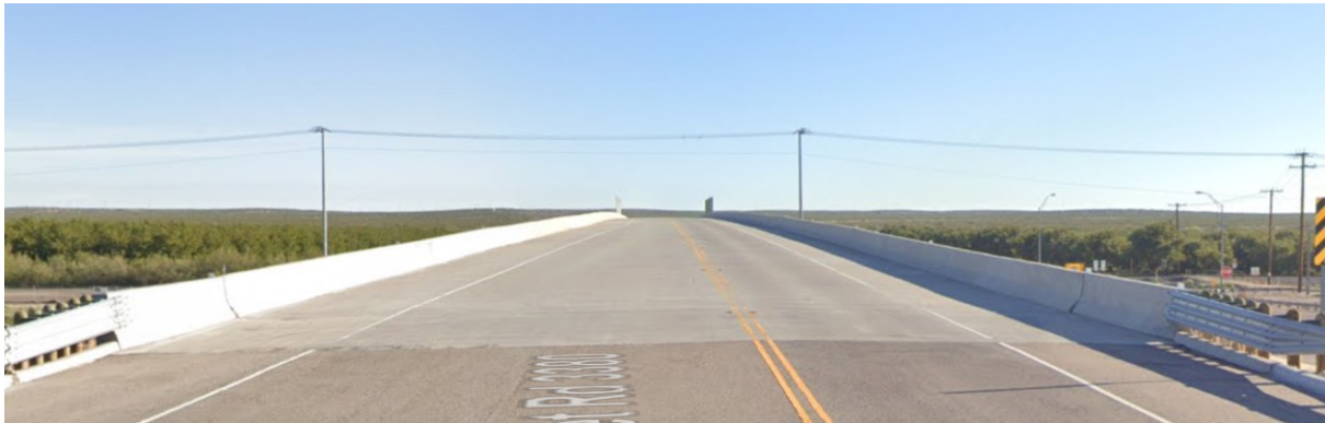
Figure 0.200. Concrete Deck of the Bridge (source: google maps)
