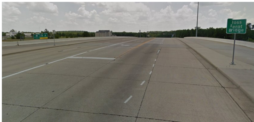
Figure 0.105. Concrete Deck of the Bridge (source: google maps)
