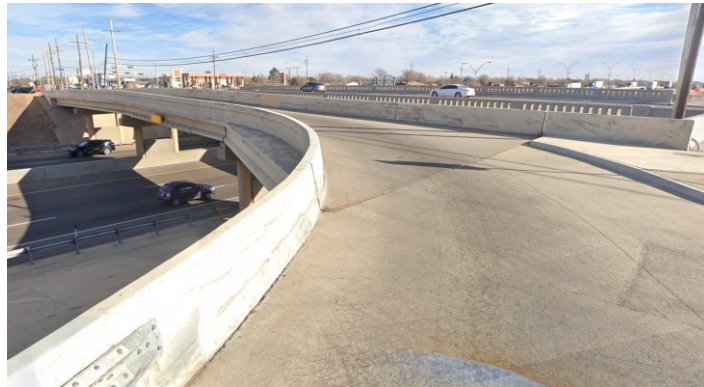
Figure 0.50. Concrete Deck of the Bridge (source: google maps)
