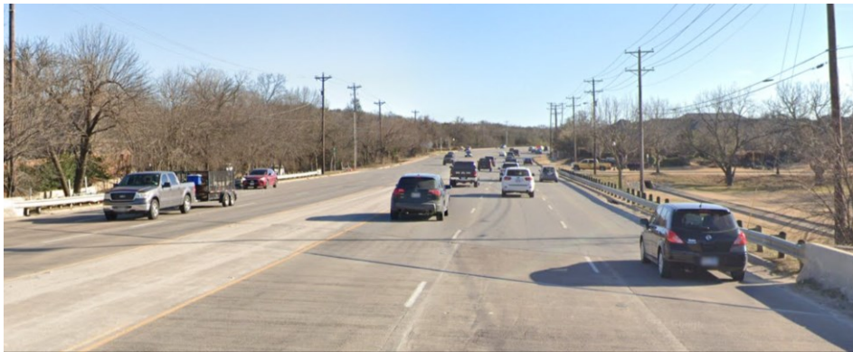
Figure 0.280. Concrete Deck of the Bridge (source: google maps)
