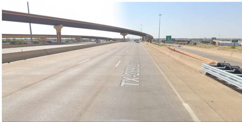
Figure 0.346. Concrete Deck of the Bridge (source: google maps)
