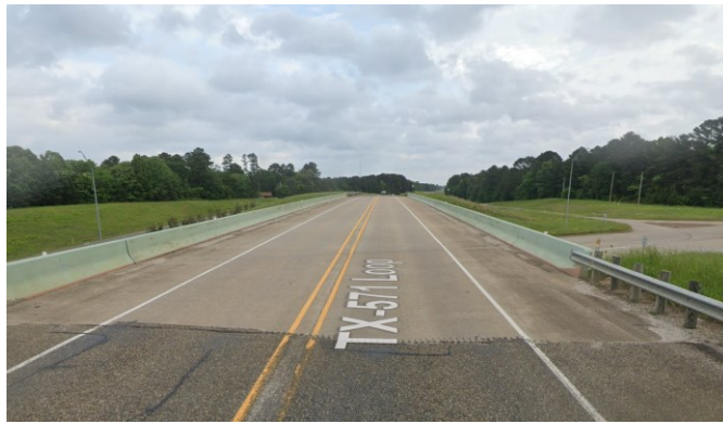
Figure 0.365. Concrete Deck of the Bridge (source: google maps)
