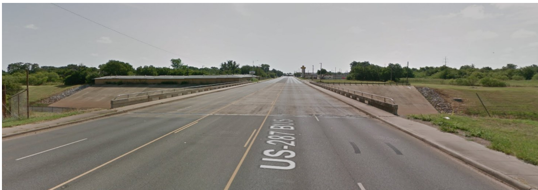
Figure 0.387. Concrete Deck of the Bridge (source: google maps)
