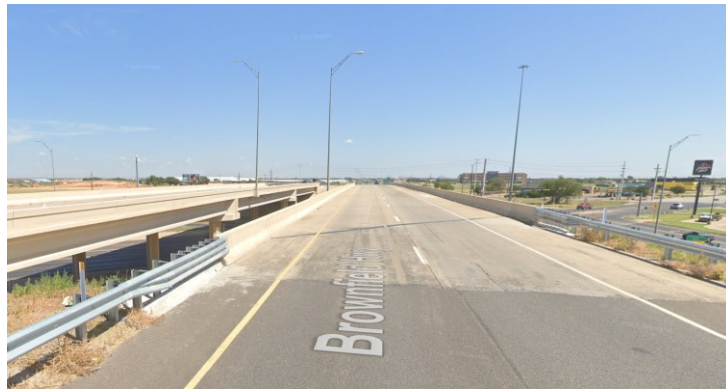
Figure 0.338. Concrete Deck of the Bridge (source: google maps)
