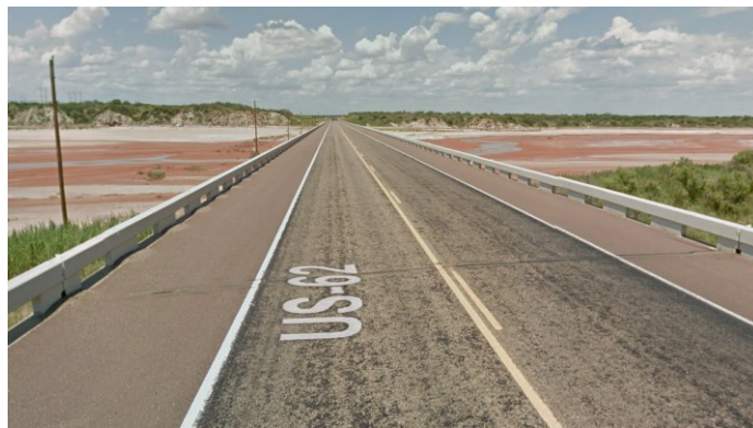
Figure 0.147. Concrete Deck of the Bridge (source: google maps)
