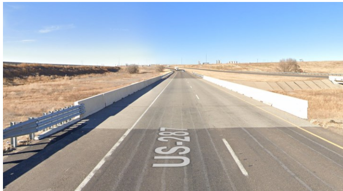
Figure 0.85. Concrete Deck of the Bridge (source: google maps)
