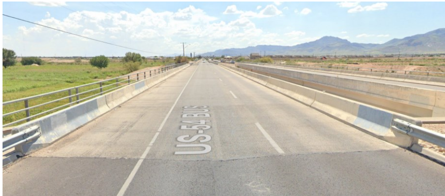
Figure 0.207. Concrete Deck of the Bridge (source: google maps)
