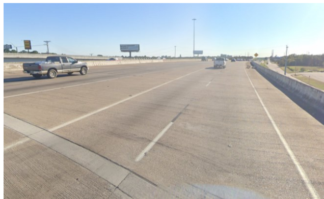
Figure 0.272. Concrete Deck of the Bridge (source: google maps)
