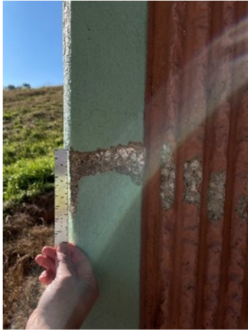
(a) Spalling at abutment wall (TYL-RC-03) (b) Crack at abutment wall (TYL-RC-03)
