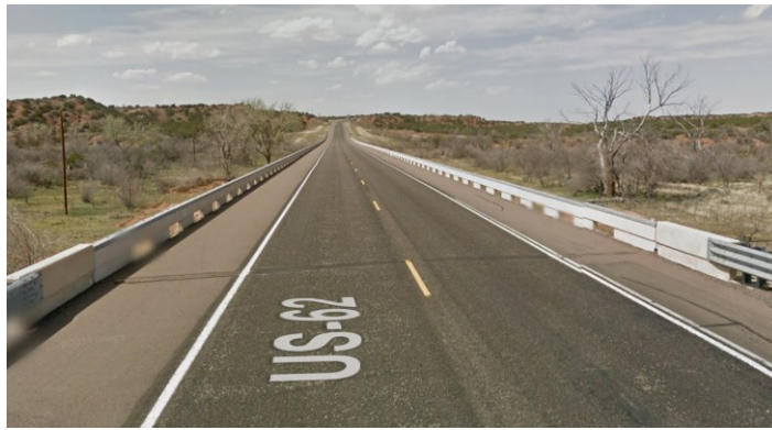
Figure 0.176. Concrete Deck of the Bridge (source: google maps)
