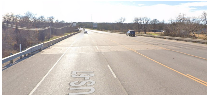
Figure 0.257. Concrete Deck of the Bridge (source: google maps)
