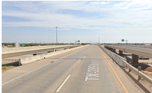
Figure 0.324. Concrete Deck of the Bridge (source: google maps)
