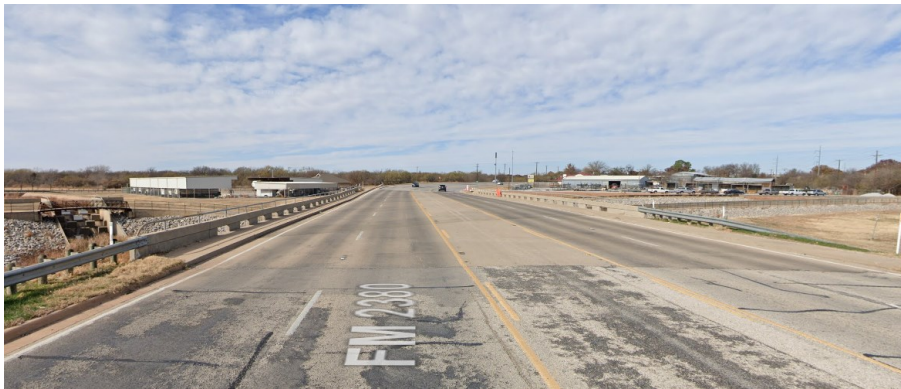
Figure 0.402. Concrete Deck of the Bridge (source: google maps)
