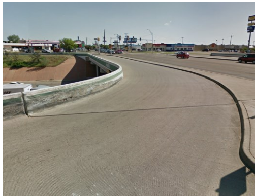
Figure 0.42. Concrete Deck of the Bridge (source: google maps)
