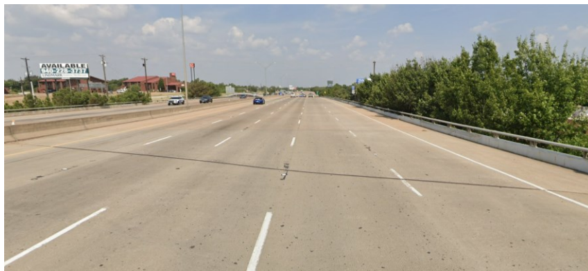
Figure 0.373. Concrete Deck of the Bridge (source: google maps)
