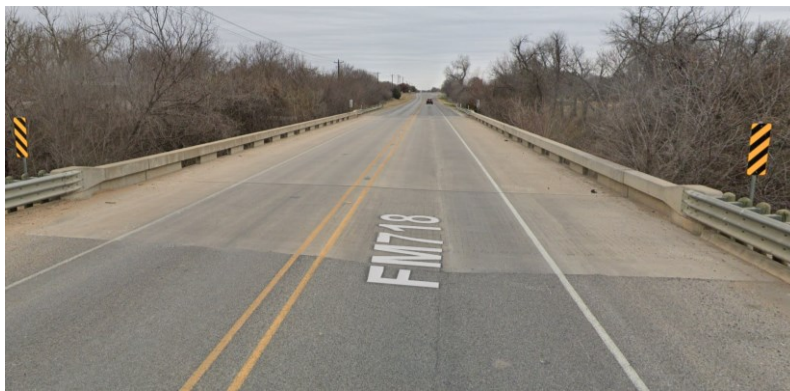
Figure 0.295. Concrete Deck of the Bridge (source: google maps)
