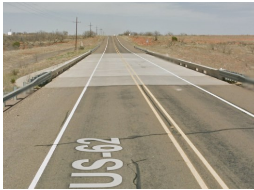
Figure 0.168. Concrete Deck of the Bridge (source: google maps)
