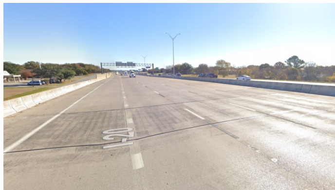
Figure 0.265. Concrete Deck of the Bridge (source: google maps)
