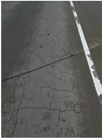
(a) Map cracks propagating from a joint (ELP-RC-01)
