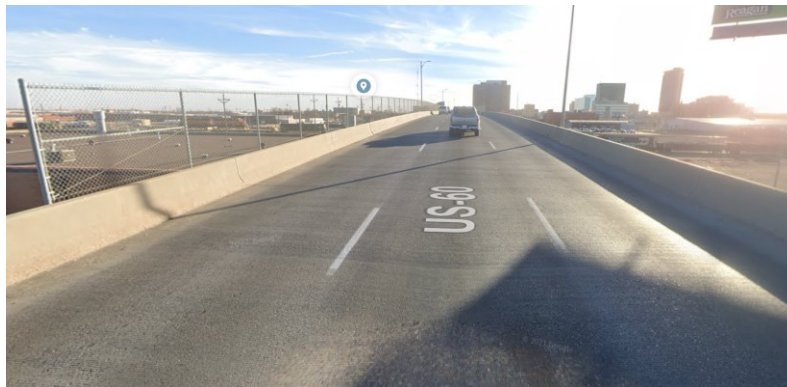
Figure B.27. Concrete Deck of the Bridge (source: google maps)
