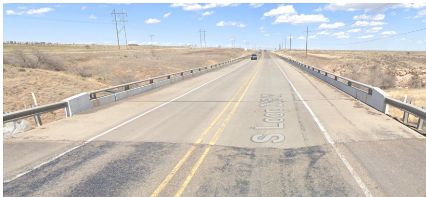
Figure 0.65. Concrete Deck of the Bridge (source: google maps)
