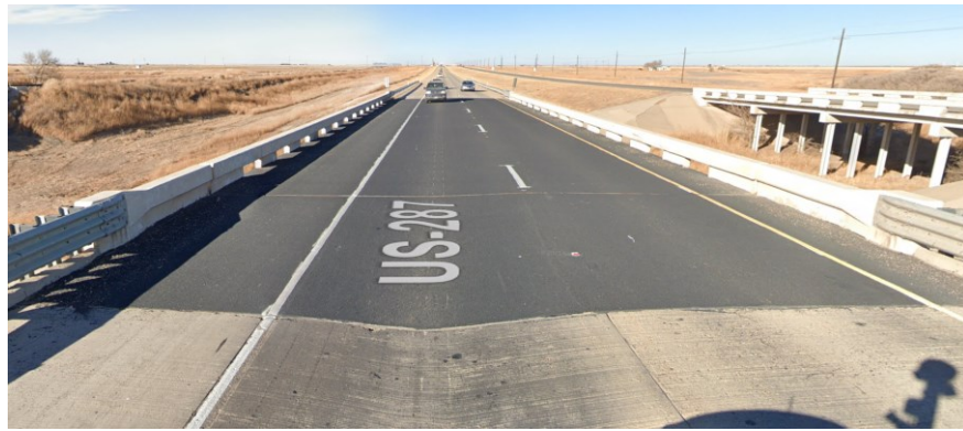
Figure 0.78. Concrete Deck of the Bridge (source: google maps)
