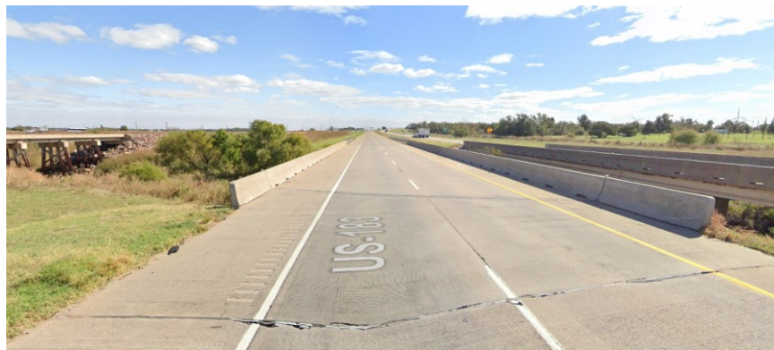
Figure 0.410. Concrete Deck of the Bridge (source: google maps)
