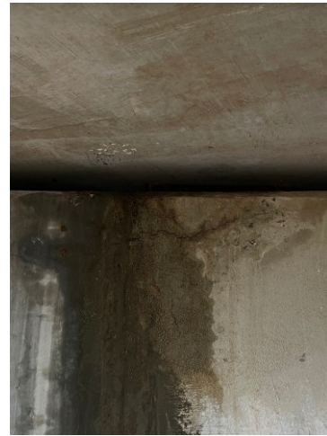
(b) Water leakage from crack at abutment (ELP-RC-01)
