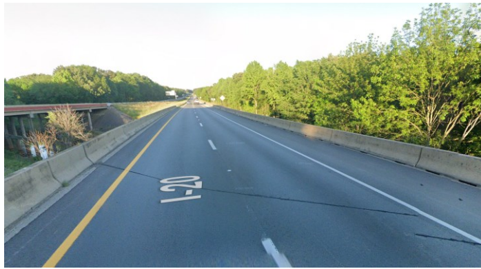
Figure 0.353. Concrete Deck of the Bridge (source: google maps)
