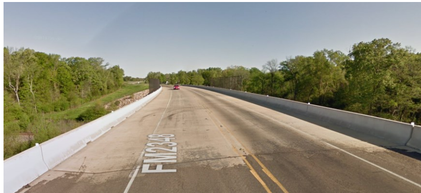
Figure 0.127. Concrete Deck of the Bridge (source: google maps)
