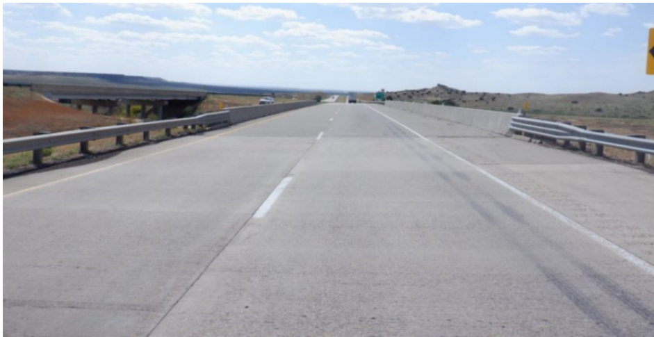
Figure B.14. Concrete Deck of the Bridge (source: google maps)
