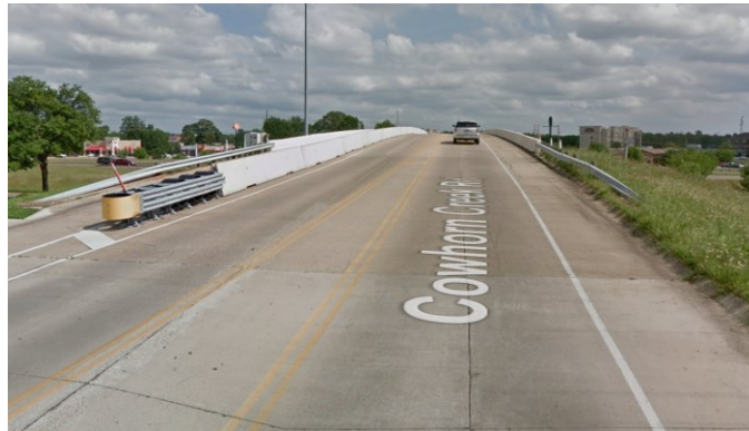
Figure 0.99. Concrete Deck of the Bridge (source: google maps)
