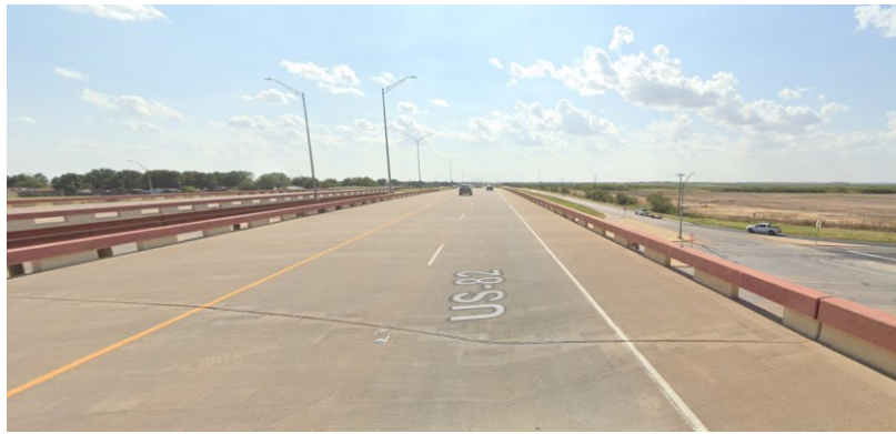
Figure 0.394. Concrete Deck of the Bridge (source: google maps)
