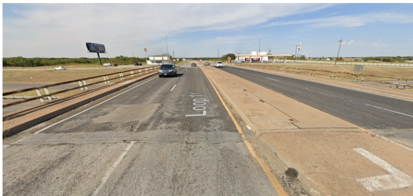
Figure 0.416. Concrete Deck of the Bridge (source: google maps)
