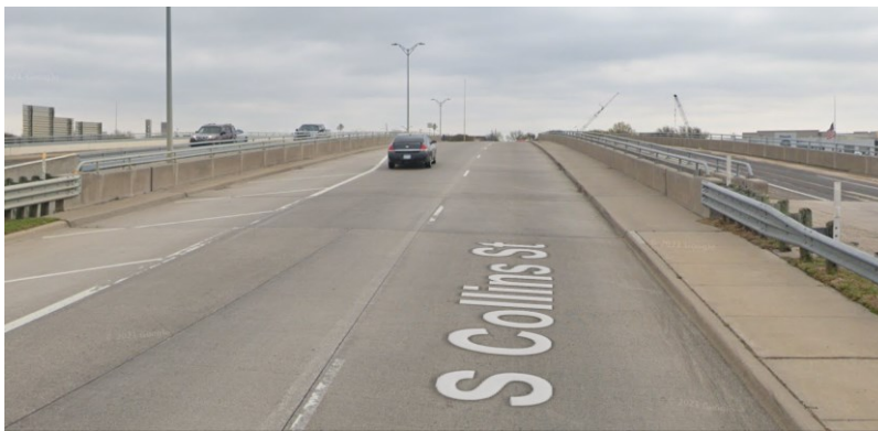
Figure 0.288. Concrete Deck of the Bridge (source: google maps)
