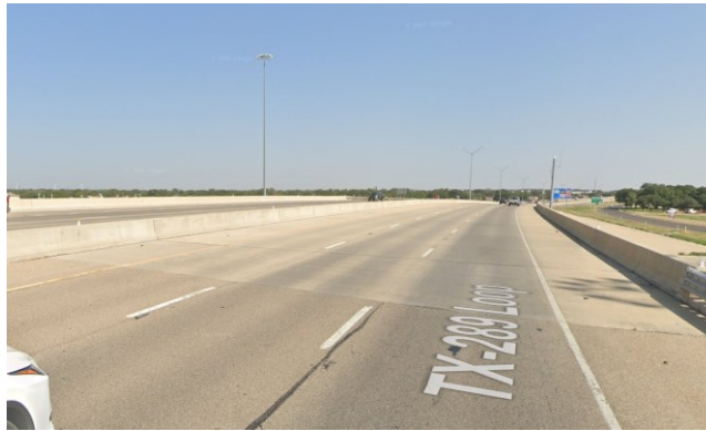
Figure 0.331 Concrete Deck of the Bridge (source: google maps)
