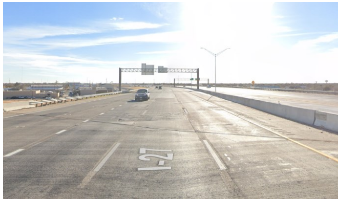
Figure 0.317. Concrete Deck of the Bridge (source: google maps)
