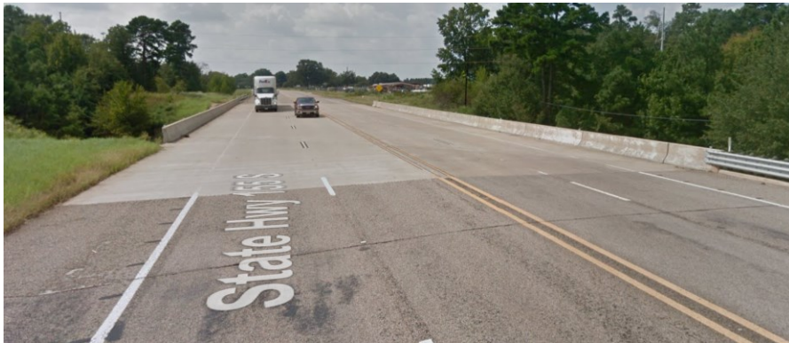
Figure 0.134. Concrete Deck of the Bridge (source: google maps)
