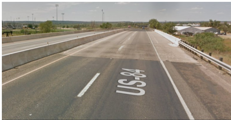
Figure 0.302. Concrete Deck of the Bridge (source: google maps)
