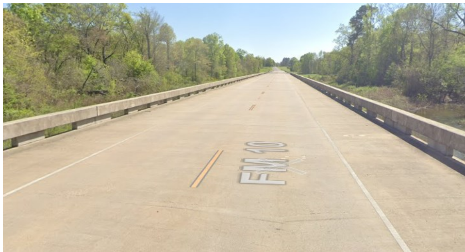
Figure 0.120. Concrete Deck of the Bridge (source: google maps)
