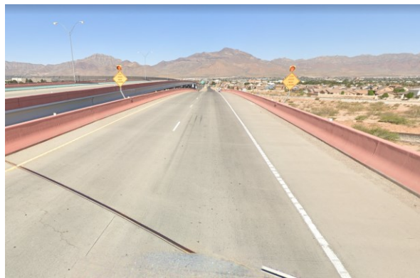
Figure 0.228. Concrete Deck of the Bridge (source: google maps)
