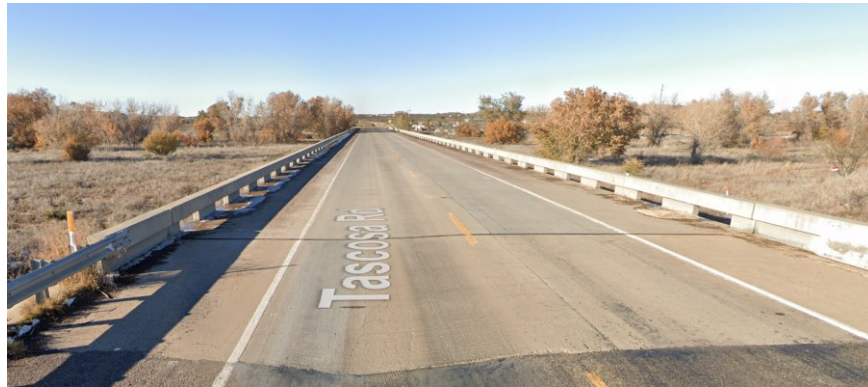
Figure 0.56. Concrete Deck of the Bridge (source: google maps)
