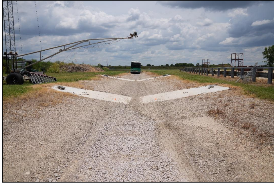
Figure 11.1. Crash Site after Test 440211-01-5.
