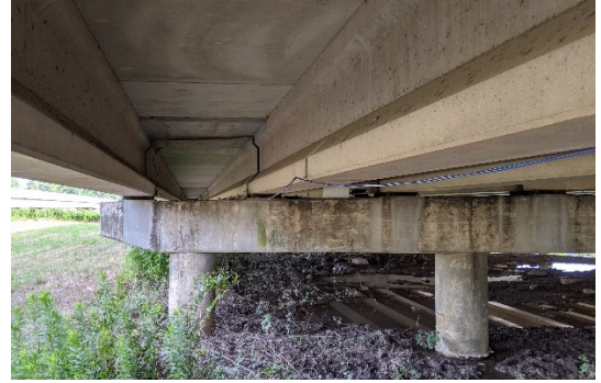
(b) View beneath bridge
