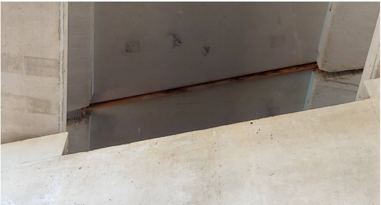
Figure 6.14. Lubbock District bridge with skewed girder end details.
