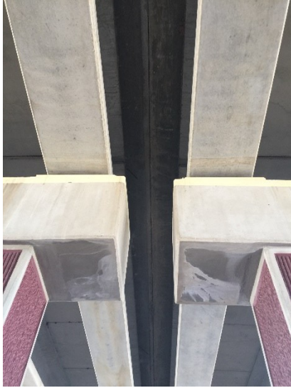
(a) CIP deck between northbound and southbound lanes
