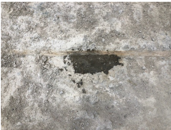
(c) Patched hole
