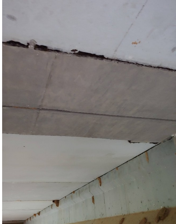
(b) Bottom of CIP region between girders
