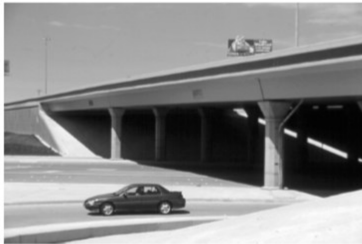
Figure 2.19. Louetta bridge, reprinted from Gross and Burns (2000).
