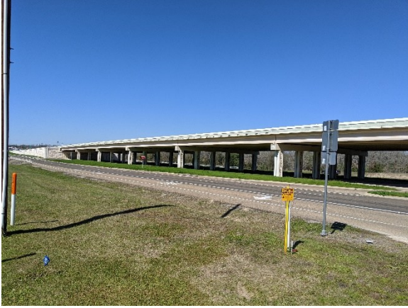
(a) Elevation view of bridge
