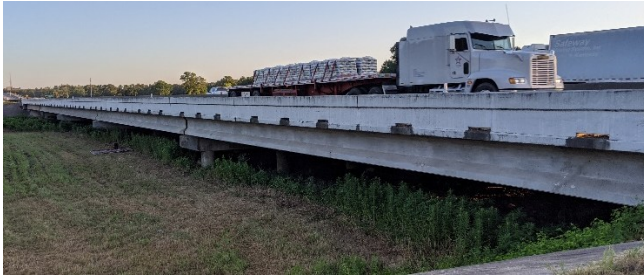
(a) Elevation view of bridge
