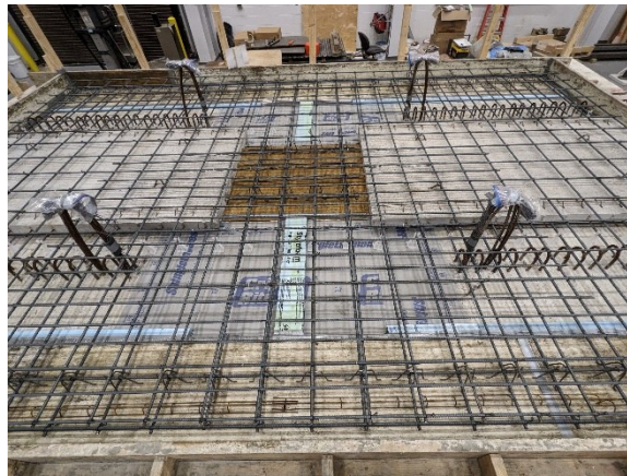
Figure 9.32. PBJ-OP2 formwork with all rebar (the north girder is at bottom and has supplemental top bars).
