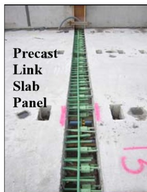
(a) Reinforced continuity provided by mechanical couplers
