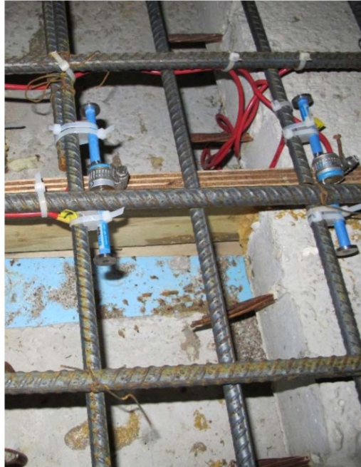
Figure 2.33. Gage attachment on reinforcement, reprinted from Munsterman (2017).
