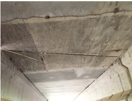
(a) CIP at continuous deck detail
