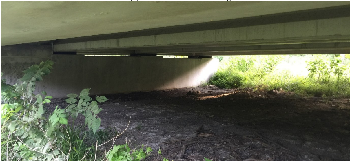
(b) View beneath bridge
