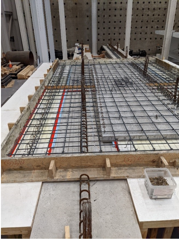
(a) Looking west
