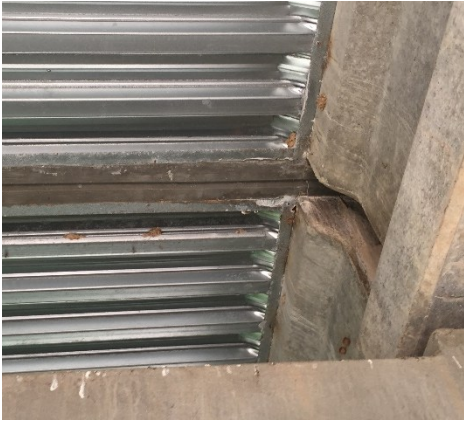
(a) PMDF at continuous deck
