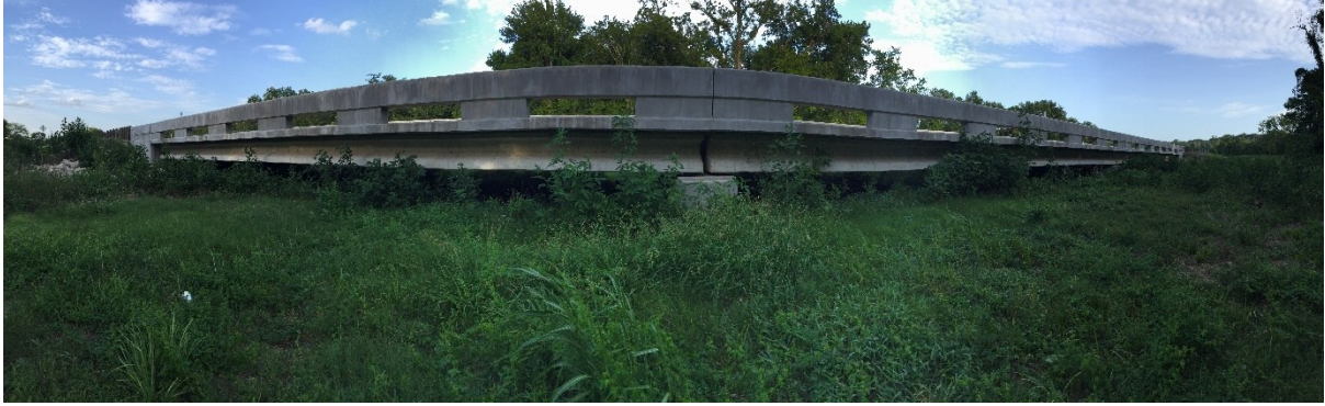
(a) Elevation view of bridge
