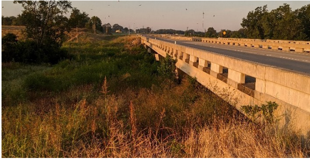
(a) Elevation view of bridge
