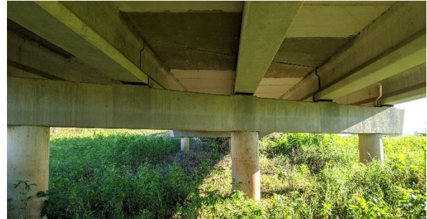
(b) View beneath bridge
