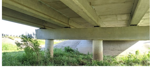
(b) View beneath bridge
