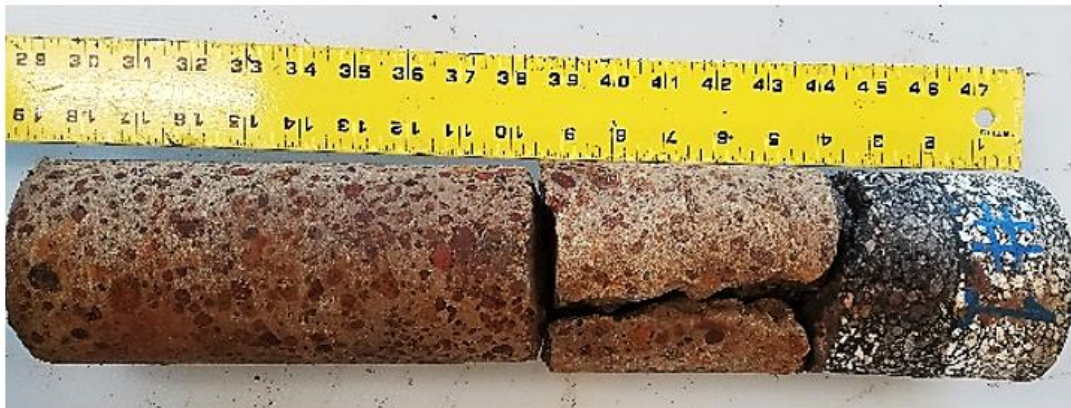
Figure 27. Main Pavement Core.
