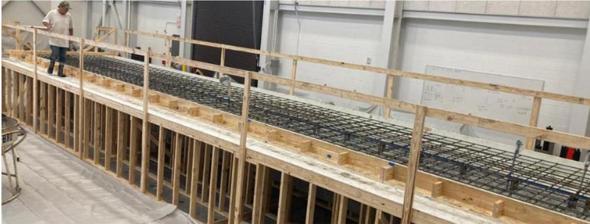
*Tx34-1 Deck Formwork and Reinforcement Mesh*
