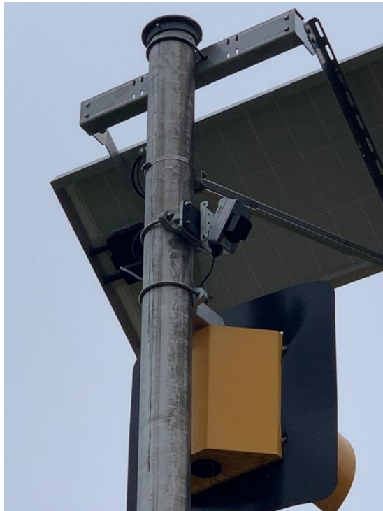
Figure 35. Example of a Sensor on the RFBA to Detect Vehicles Approaching on the Major Street.
