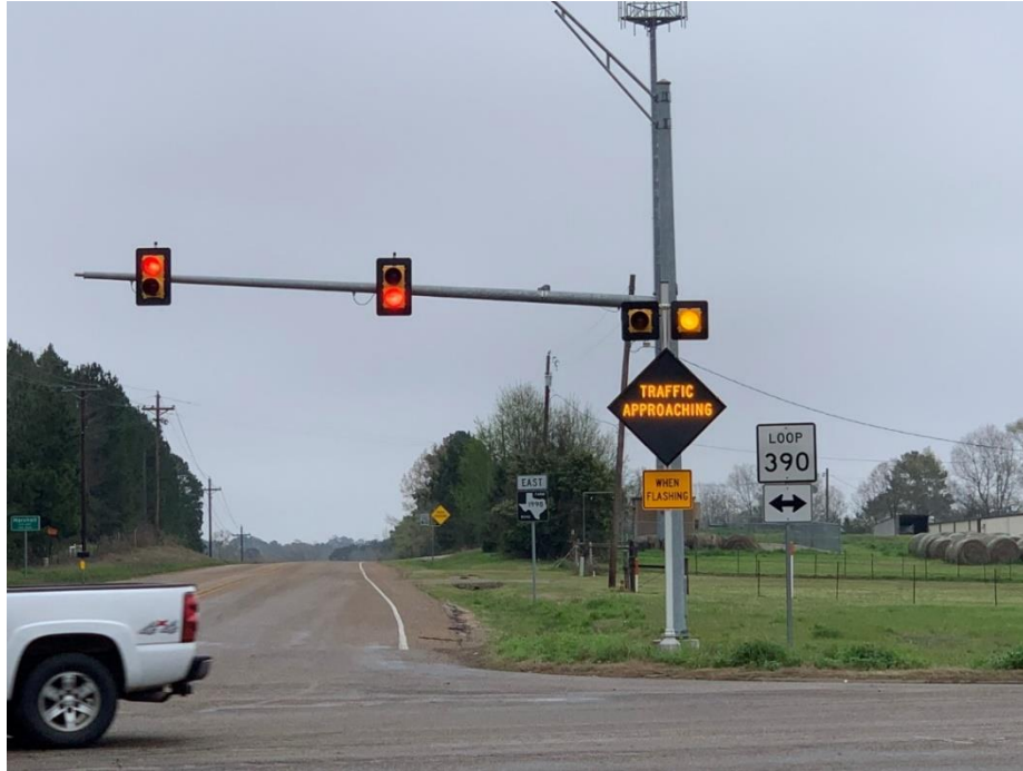
Figure 36. Example of a Warning Sign Assembly on the Minor Street (System Activated).
