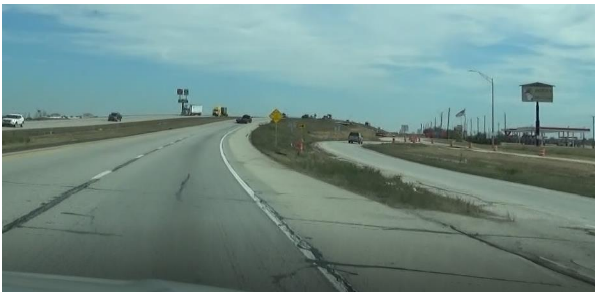
Figure 56. Exit Gore Sign Missing at Site 4.
