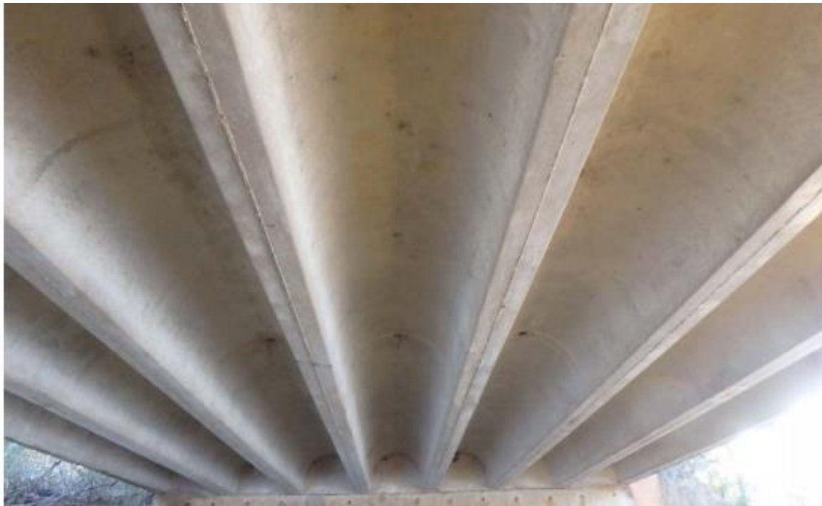
(b) Underside Superstructure View
