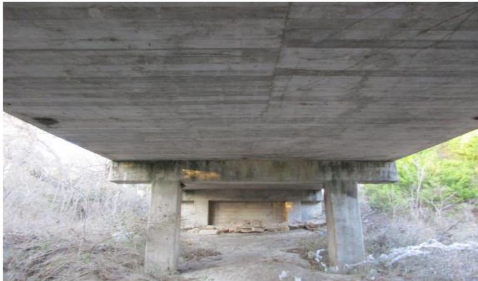
(c) Underside Superstructure View
