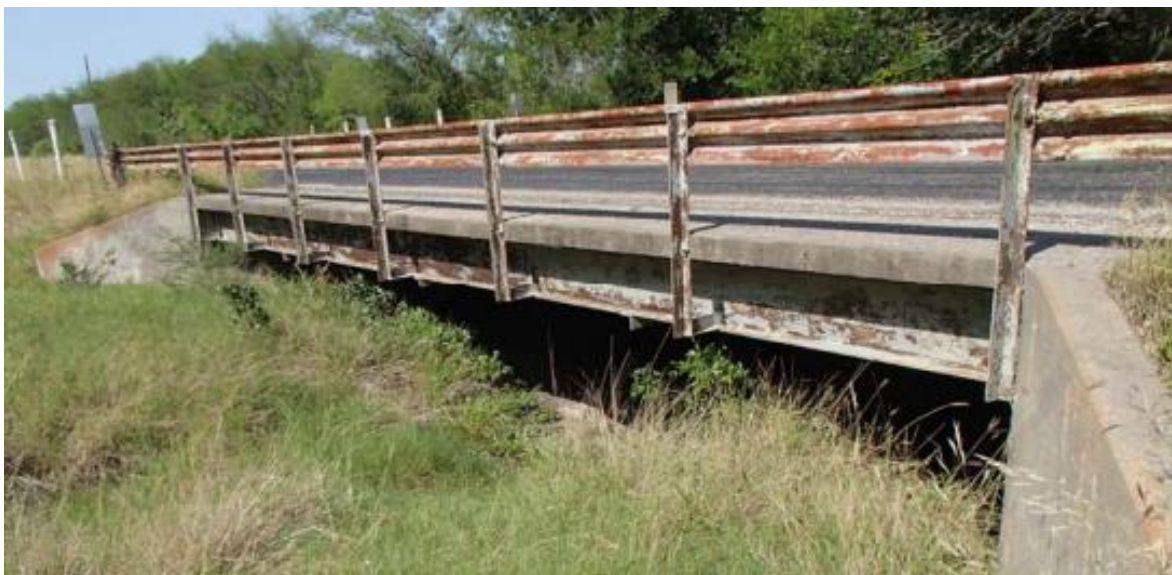
Figure B.1. Bridge SM-1 (TxDOT 2018c)
