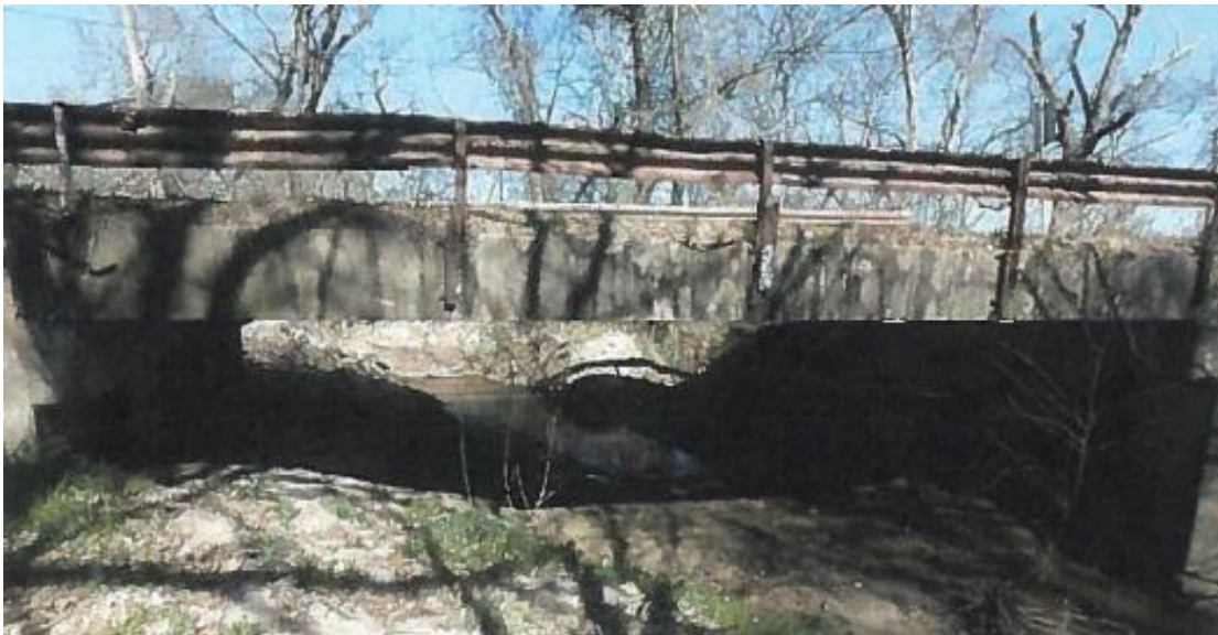
Figure 7.7. Bridge CM-5 (TxDOT 2018c)
