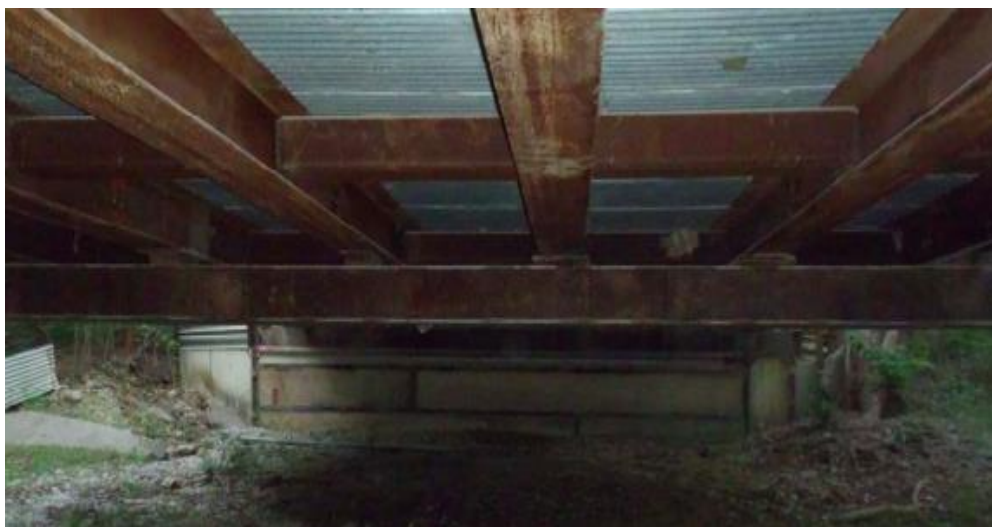
(c) Underside Superstructure View
