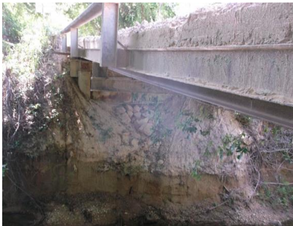
Figure B.35. Bridge SM-18 (TxDOT 2018c)
