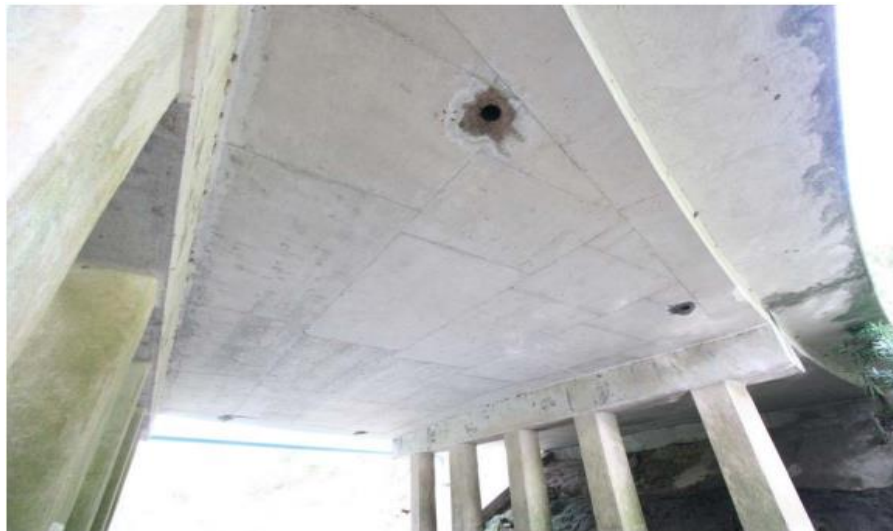
(c) Underside Superstructure View
