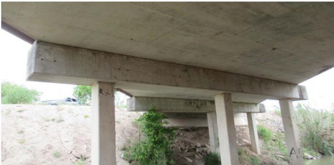
(c) Underside Superstructure View
