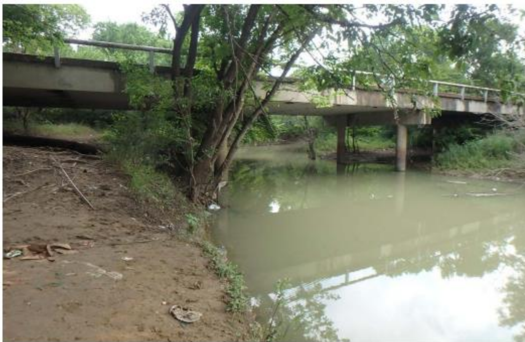
Figure C.59. Bridge CM-7 (TxDOT 2018c)
