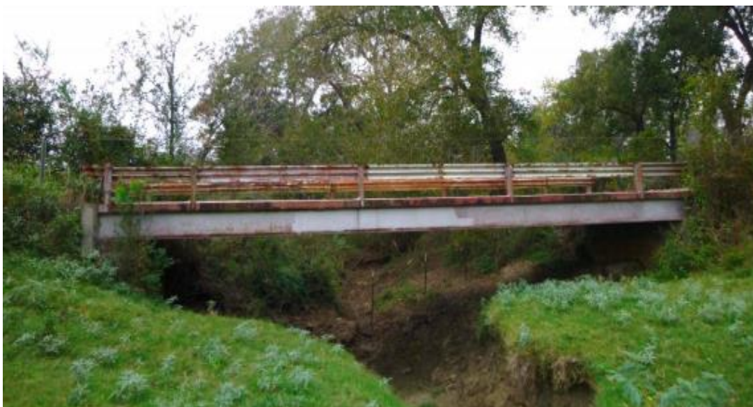
Figure B.45. Bridge SM-23 (TxDOT 2018c)
