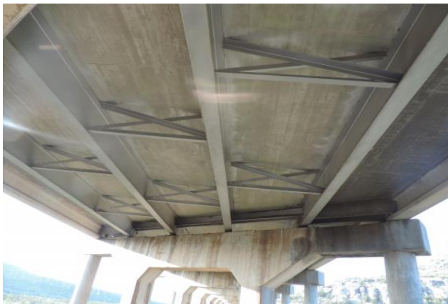
(c) Underside Superstructure View
