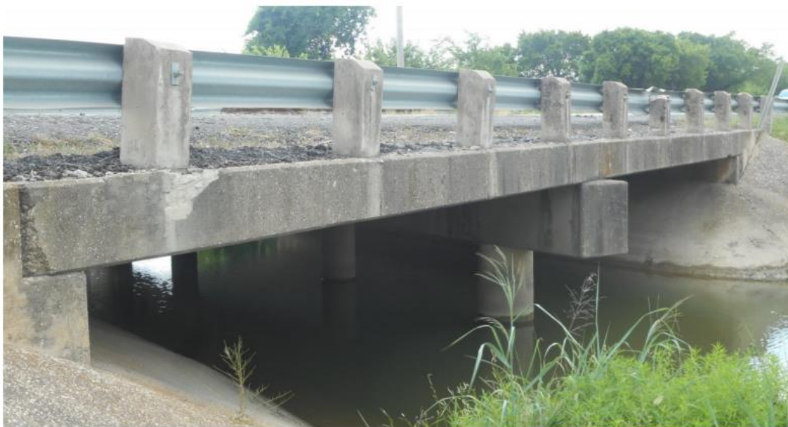
Figure C.19. Bridge CS-10 (TxDOT 2018c)
