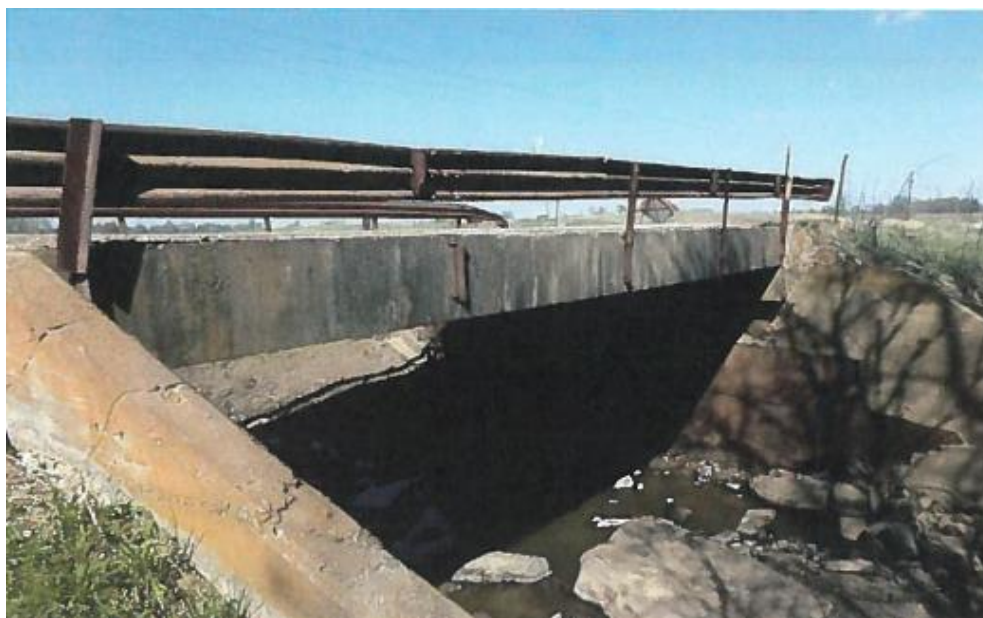
Figure C.53. Bridge CM-4 (TxDOT 2018c)
