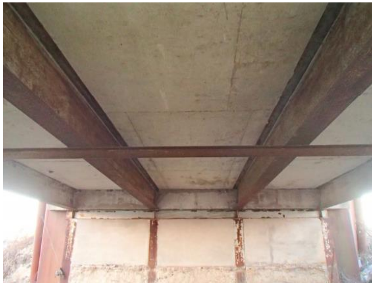
(c) Underside Superstructure View
