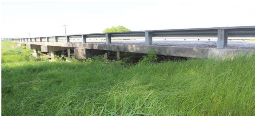
Figure C.35. Bridge CS-18 (TxDOT 2018c)
