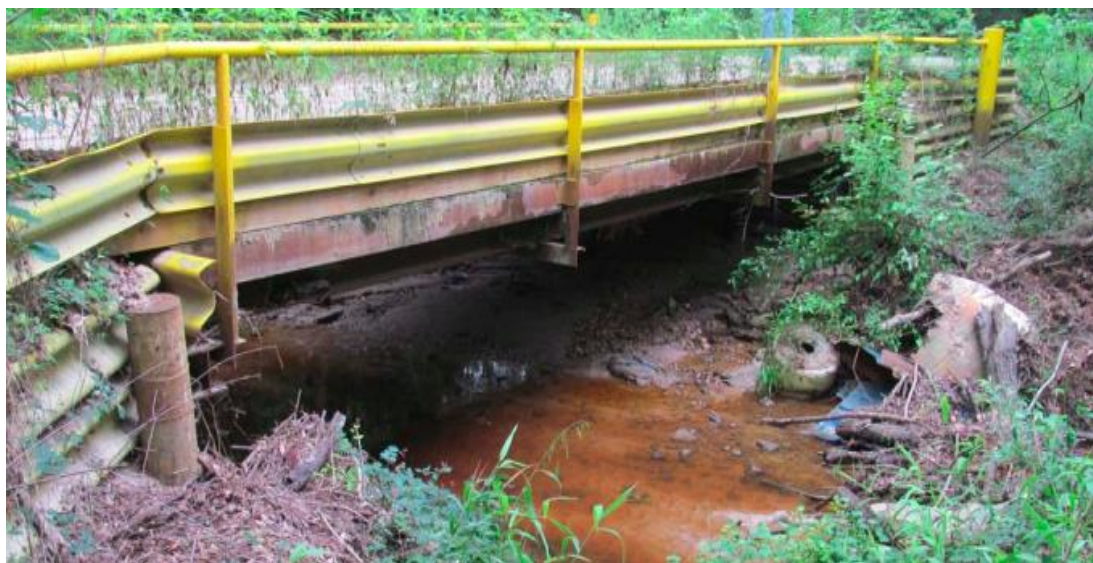
Figure B.47. Bridge SM-24 (TxDOT 2018c)
