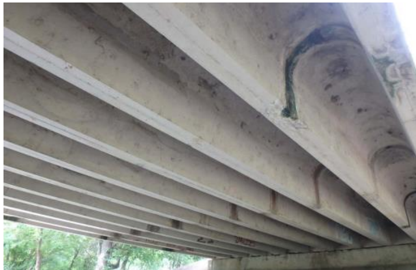
(c) Underside Superstructure View
