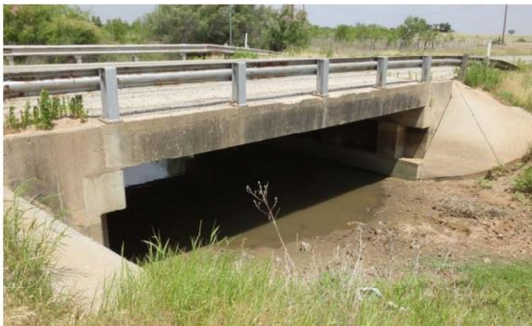
Figure C.47. Bridge CM-1 (TxDOT 2018c)
