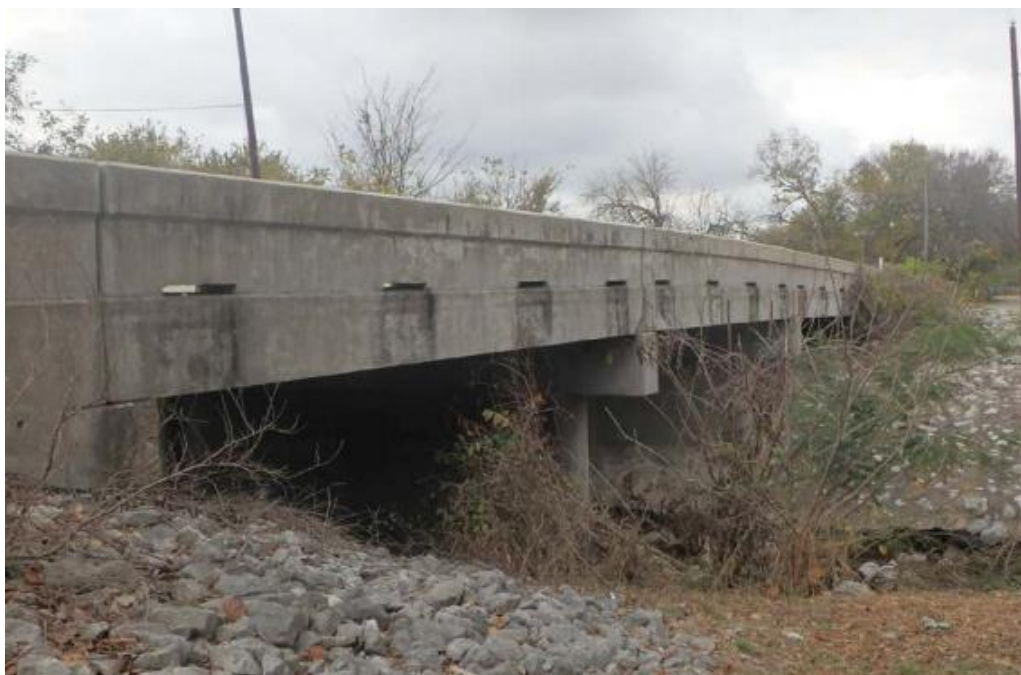
Figure C.73. Bridge CM-14 (TxDOT 2018c)
