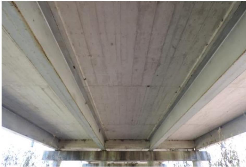
(c) Underside Superstructure View
