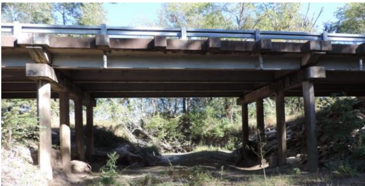
Figure B.7. Bridge SM-4 (TxDOT 2018c)
