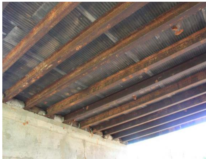
(c) Underside Superstructure View
