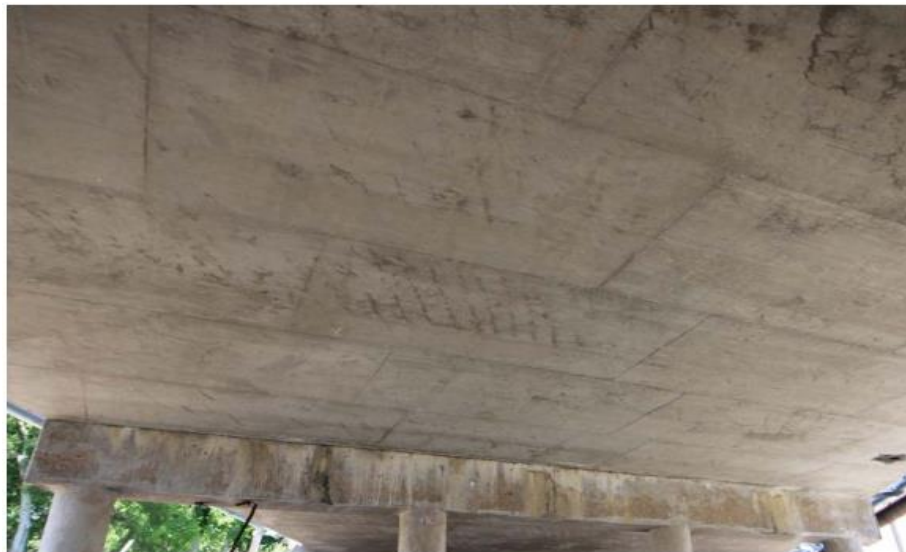
(c) Underside Superstructure View
