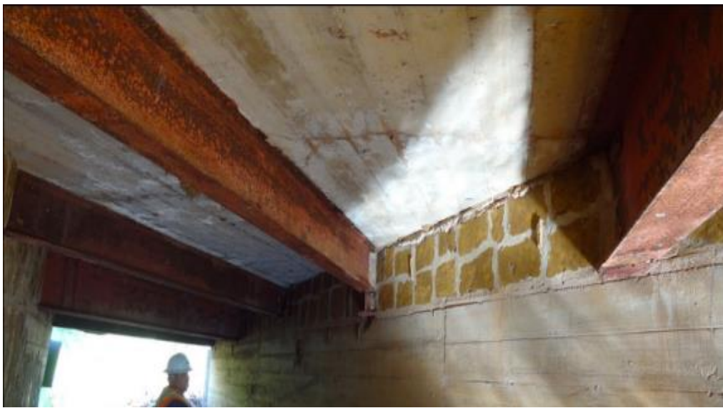
(c) Underside Superstructure View
