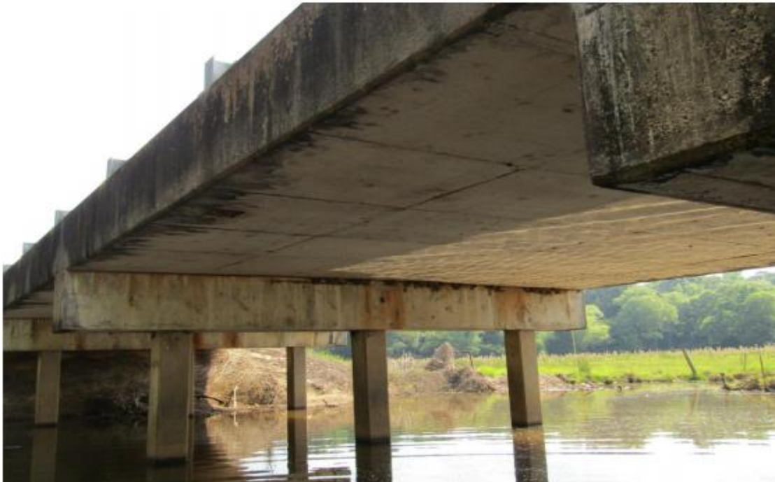
(c) Underside Superstructure View
