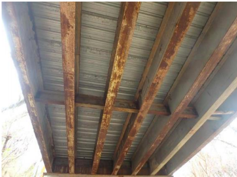
(c) Underside Superstructure View
