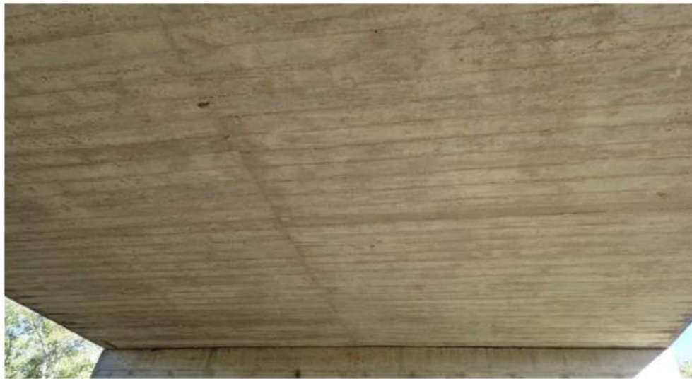
(c) Underside Superstructure View
