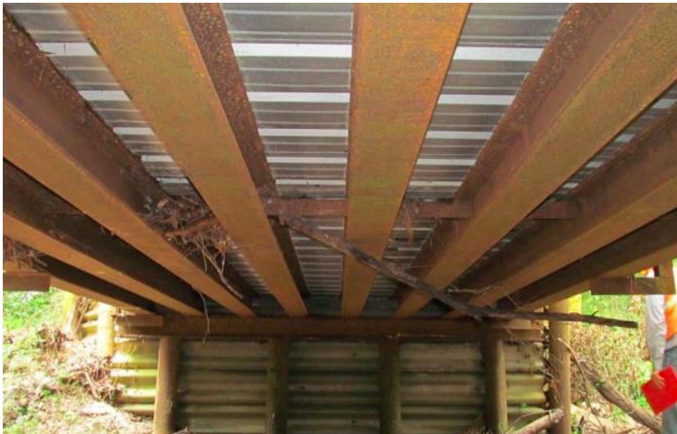
(c) Underside Superstructure View
