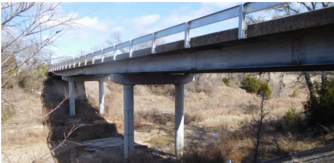
Figure 7.3. Bridge SC-12 (TxDOT 2018c)
