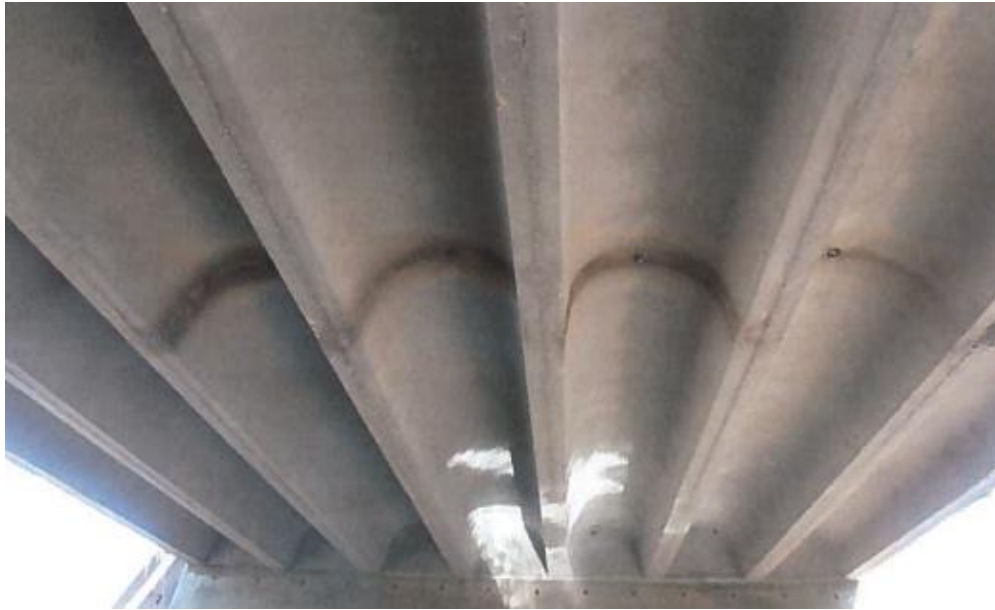
(c) Underside Superstructure View
