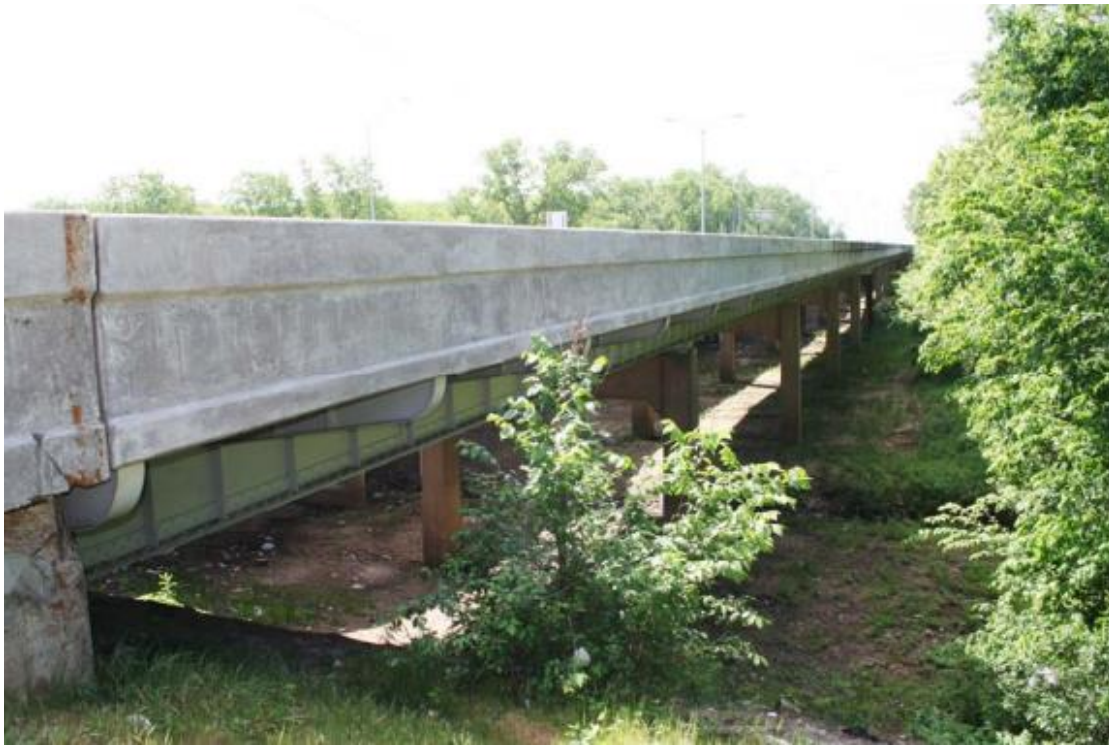
Figure B.69. Bridge SC-10 (TxDOT 2018c)
