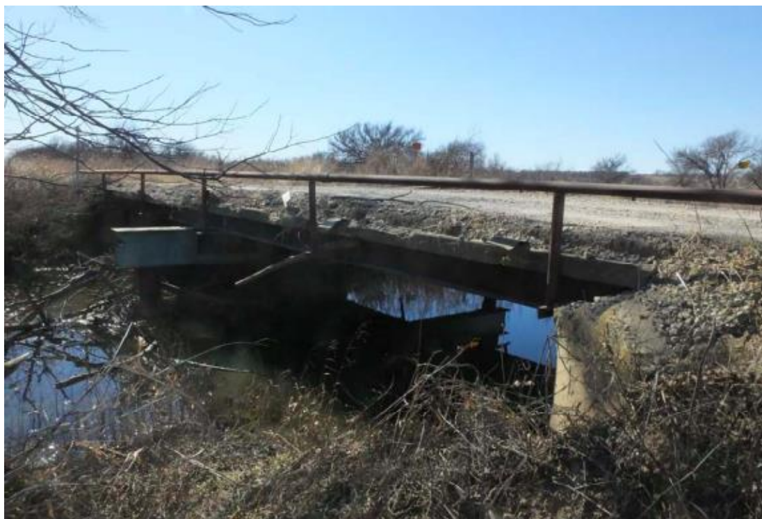
Figure B.57. Bridge SC-4 (TxDOT 2018c)
