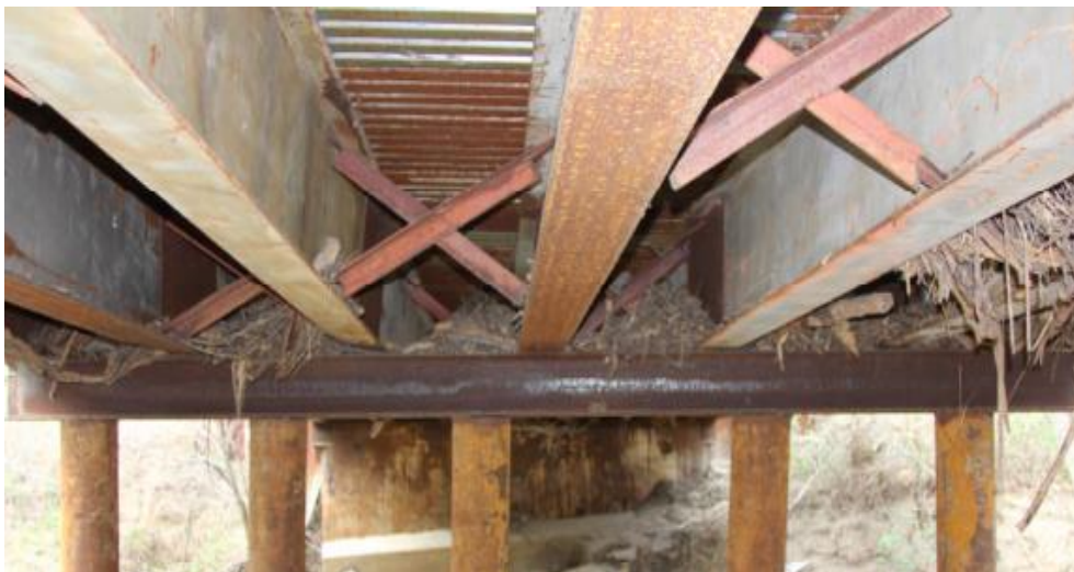
(c) Underside Superstructure View
