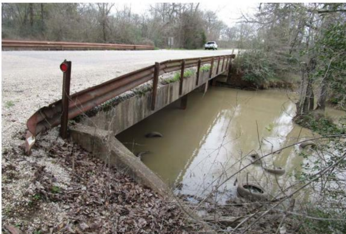
Figure C.49. Bridge CM-2 (TxDOT 2018c)
