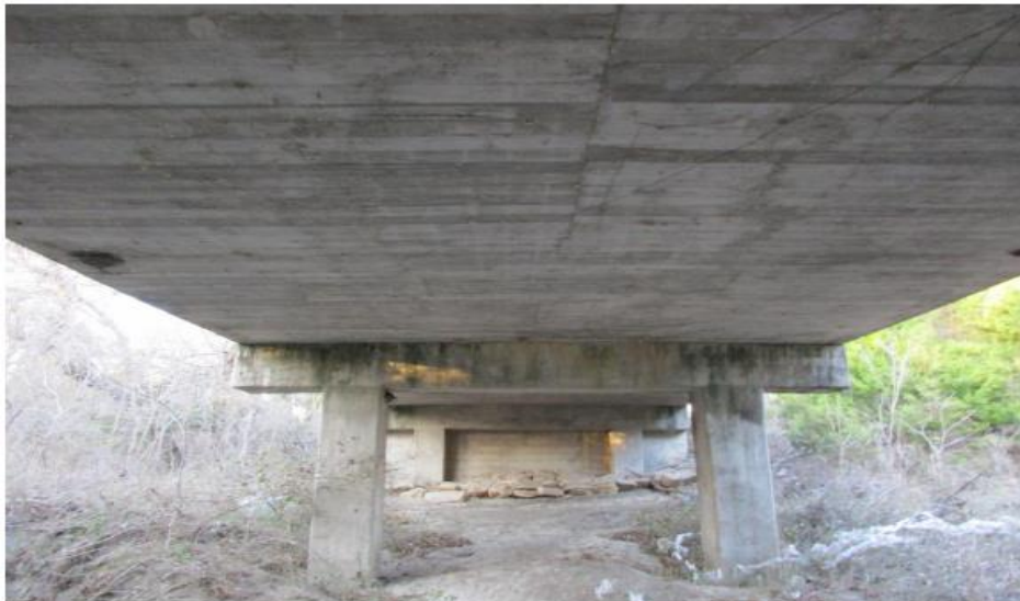
(c) Underside Superstructure View
