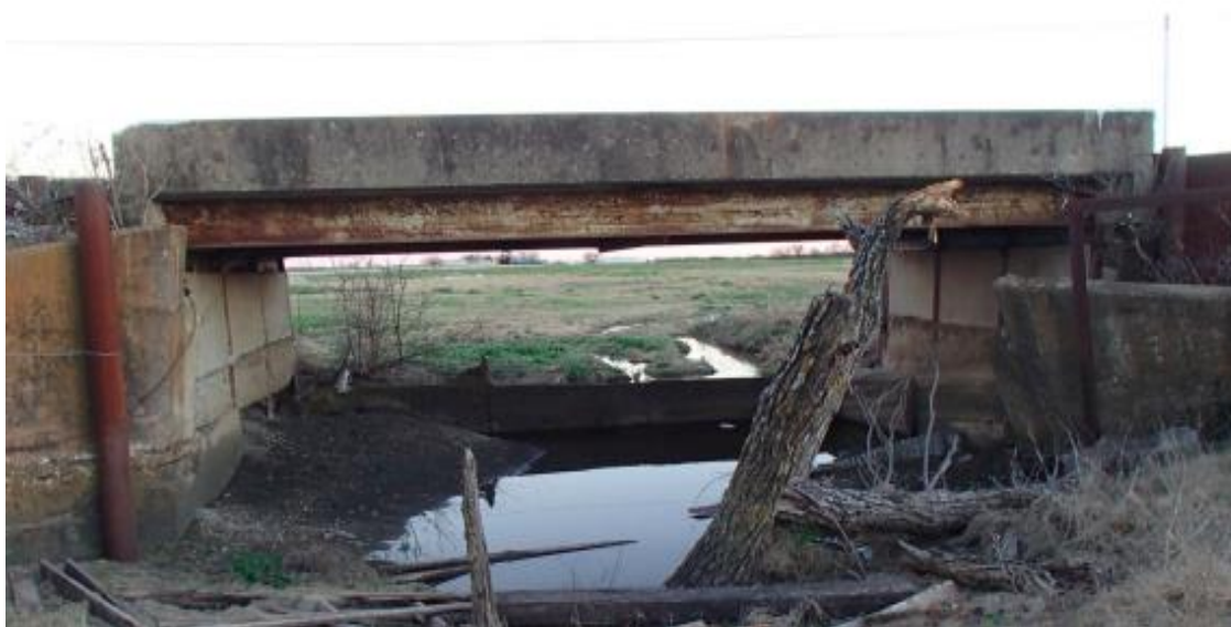
Figure B.23. Bridge SM-12 (TxDOT 2018c)
