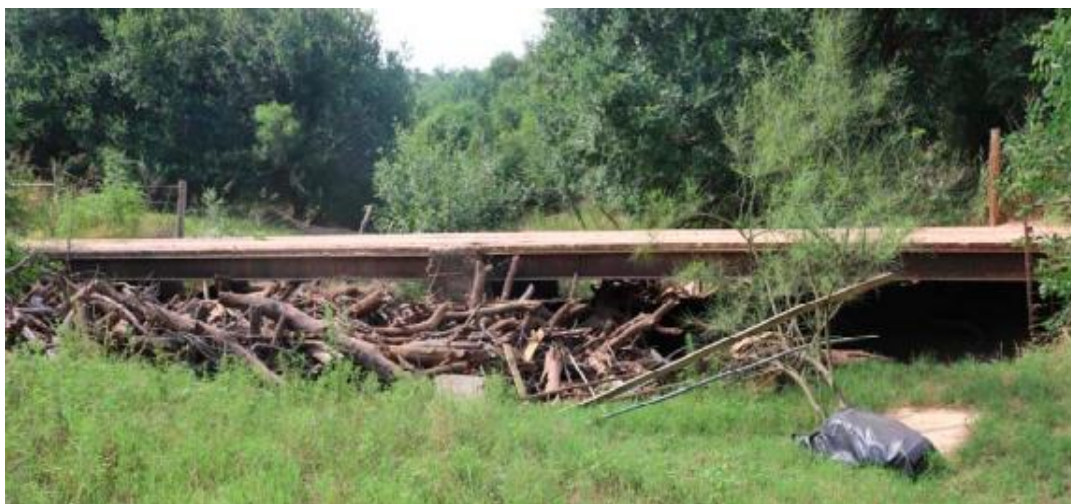
Figure B.53. Bridge SC-2 (TxDOT 2018c)
