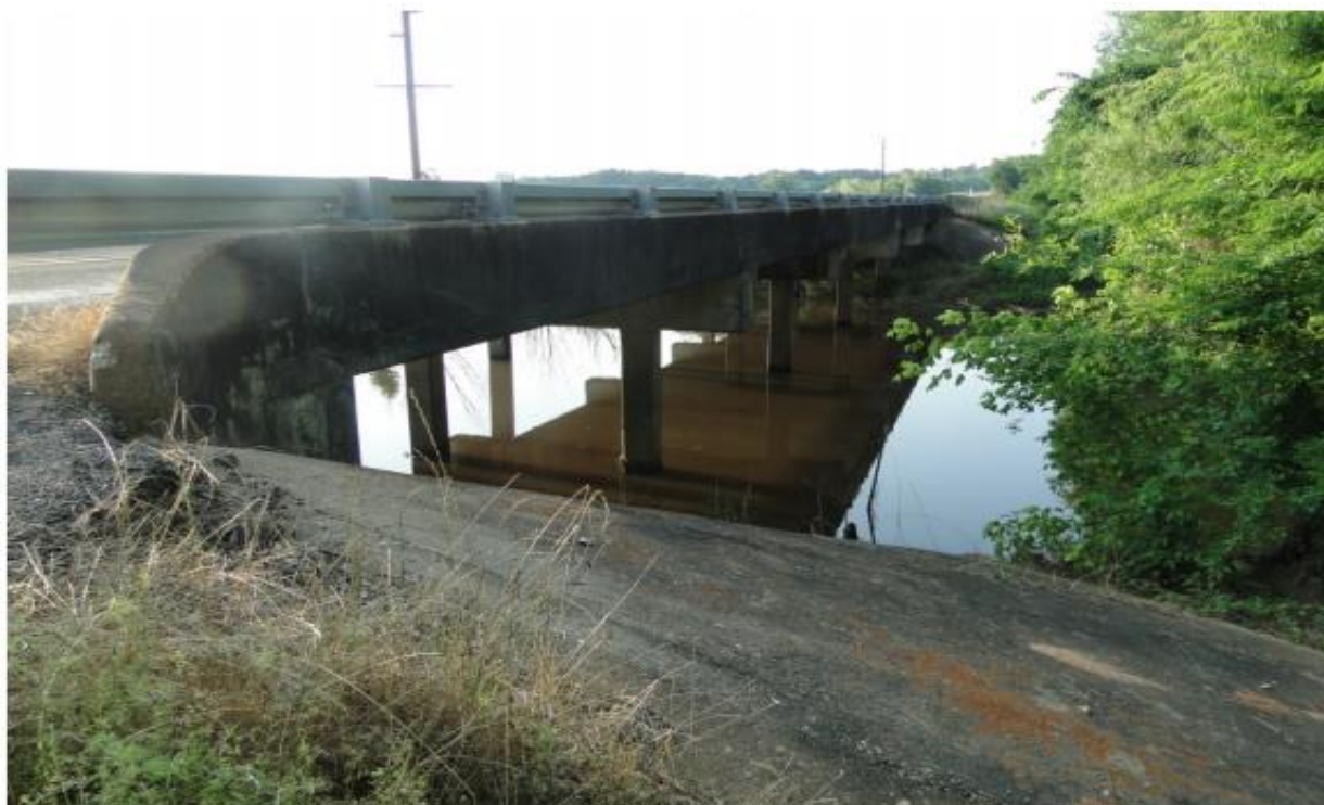
Figure C.29. Bridge CS-15 (TxDOT 2018c)
