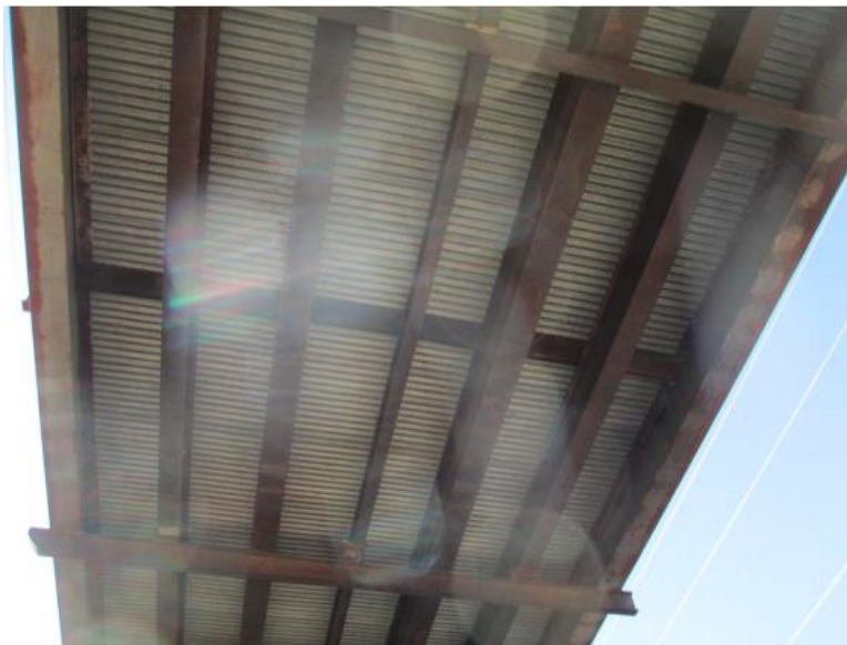
(c) Underside Superstructure View
