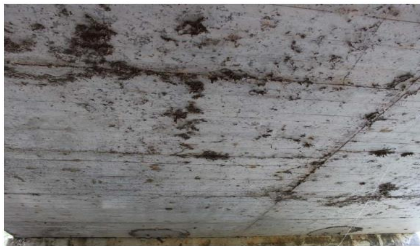
(c) Underside Superstructure View
