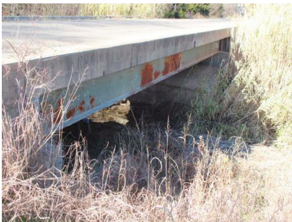
Figure B.43. Bridge SM-22 (TxDOT 2018c)
