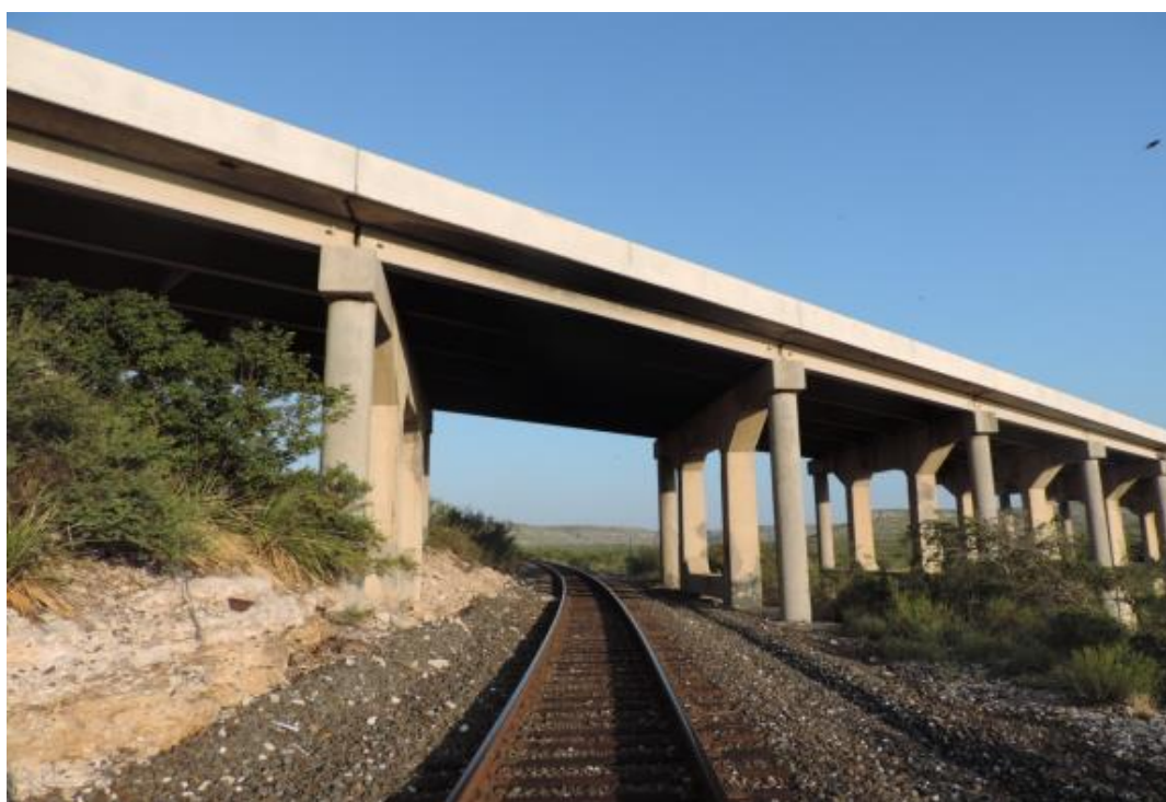
Figure B.21. Bridge SM-11 (TxDOT 2018c)
