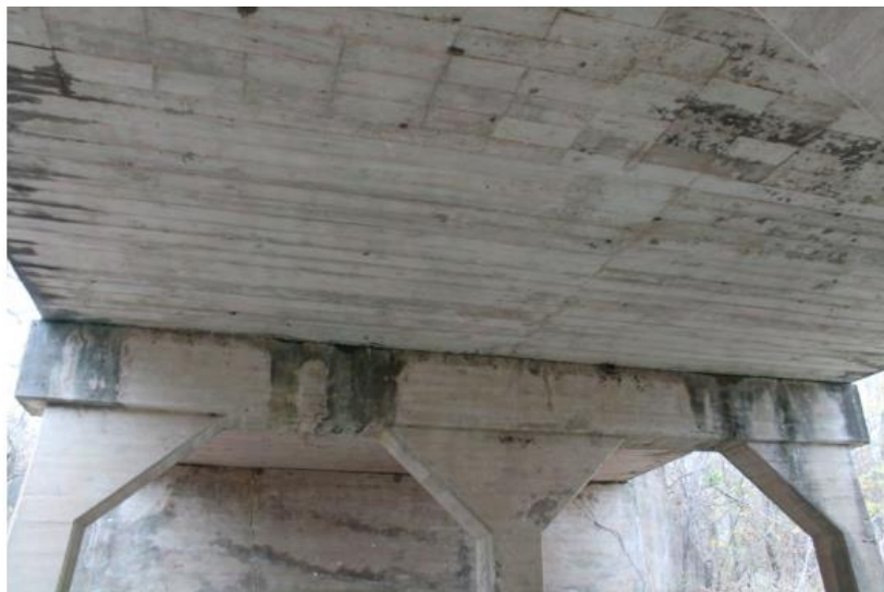
(c) Underside Superstructure View
