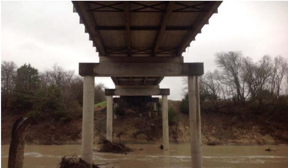
(c) Underside Superstructure View
