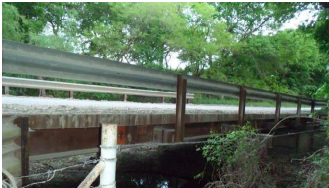
Figure B.79. Bridge SC-15 (TxDOT 2018c)
