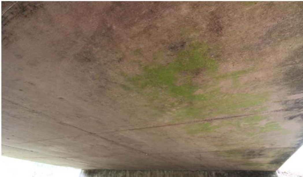
(c) Underside Superstructure View
