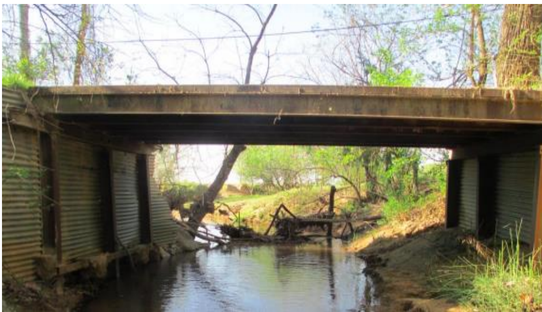
Figure B.37. Bridge SM-19 (TxDOT 2018c)
