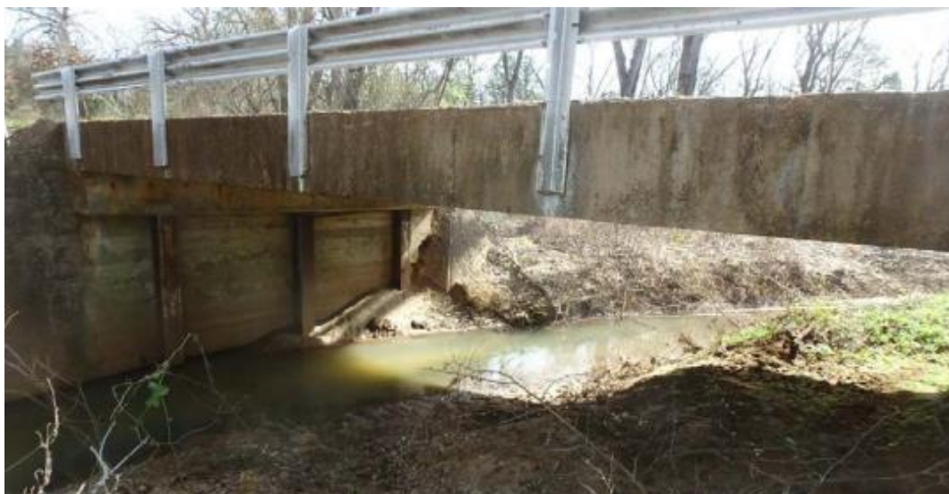
Figure C.61. Bridge CM-8 (TxDOT 2018c)
