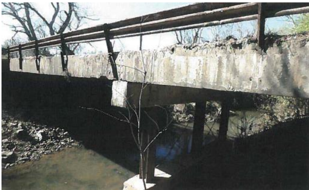
Figure C.51. Bridge CM-3 (TxDOT 2018c)
