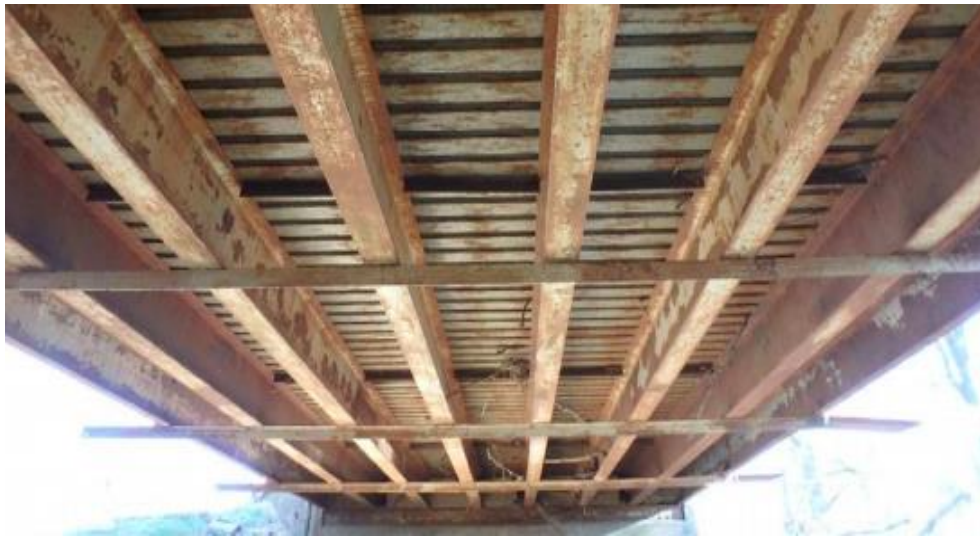
(c) Underside Superstructure View
