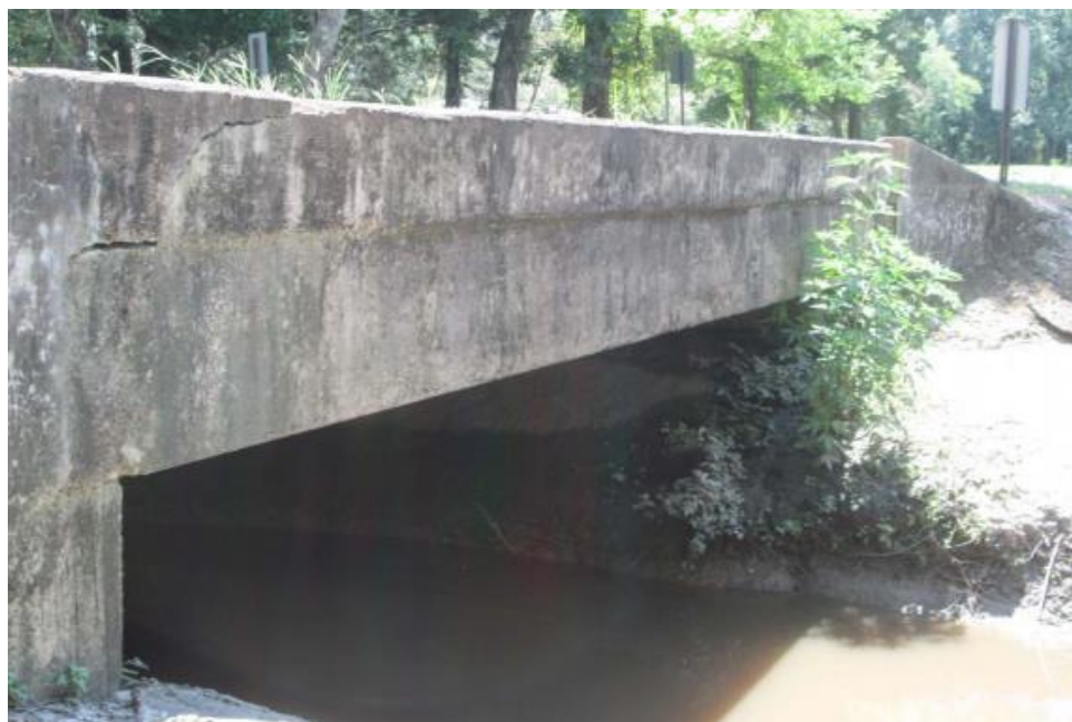
Figure C.63. Bridge CM-9 (TxDOT 2018c)
