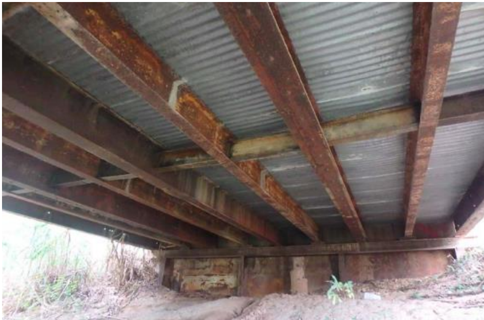
(c) Underside Superstructure View
