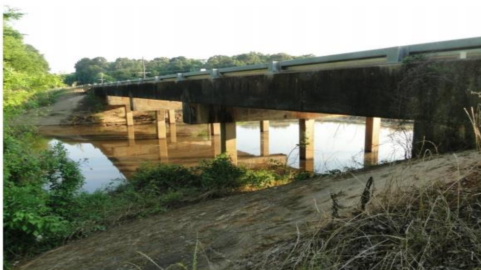
Figure C.31. Bridge CS-16 (TxDOT 2018c)
