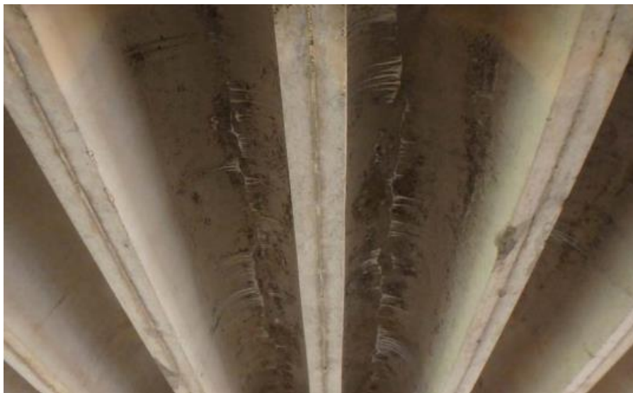
(c) Underside Superstructure View
