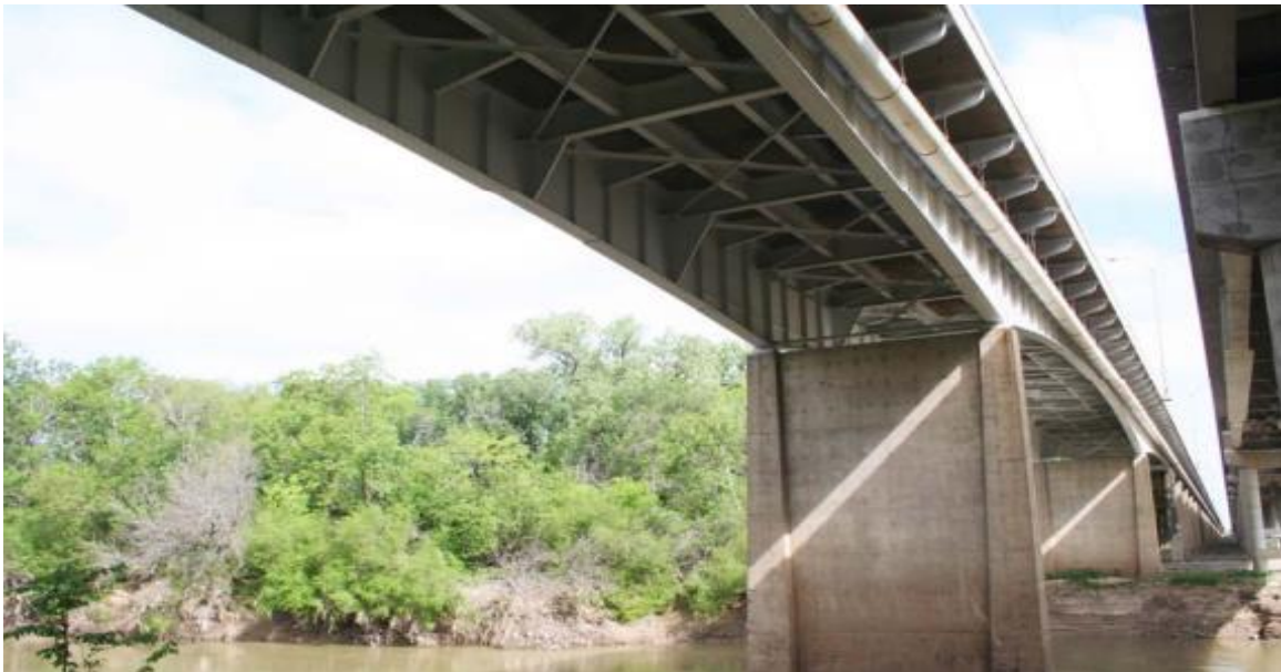
(c) Underside Superstructure View
