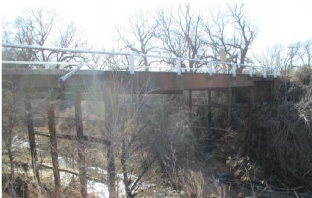
Figure B.17. Bridge SM-9 (TxDOT 2018c)
