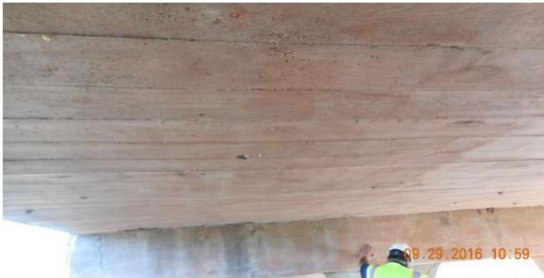
(c) Underside Superstructure View
