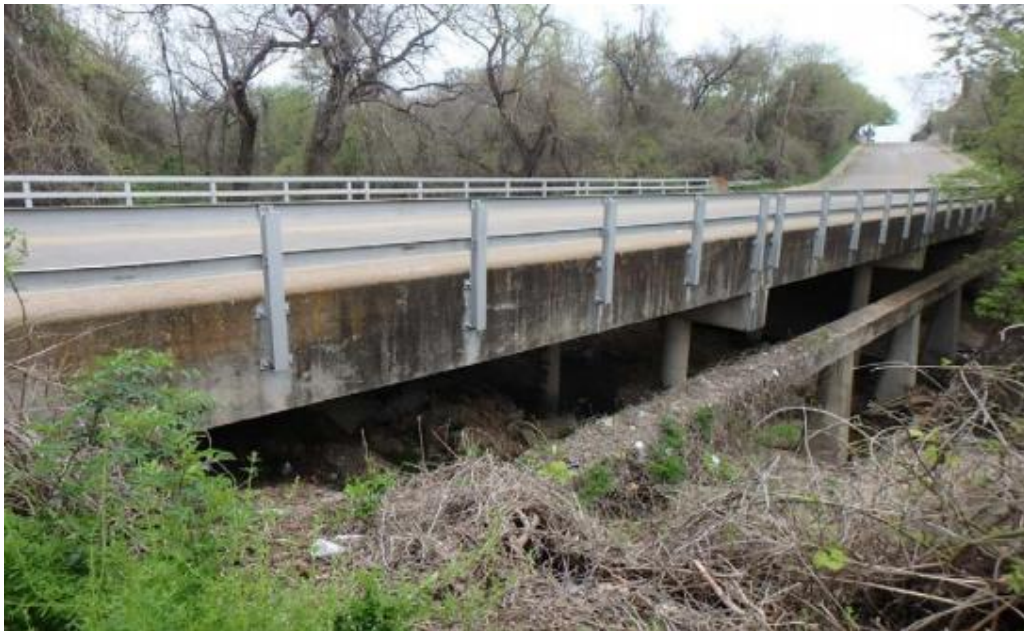
Figure C.67. Bridge CM-11 (TxDOT 2018c)
