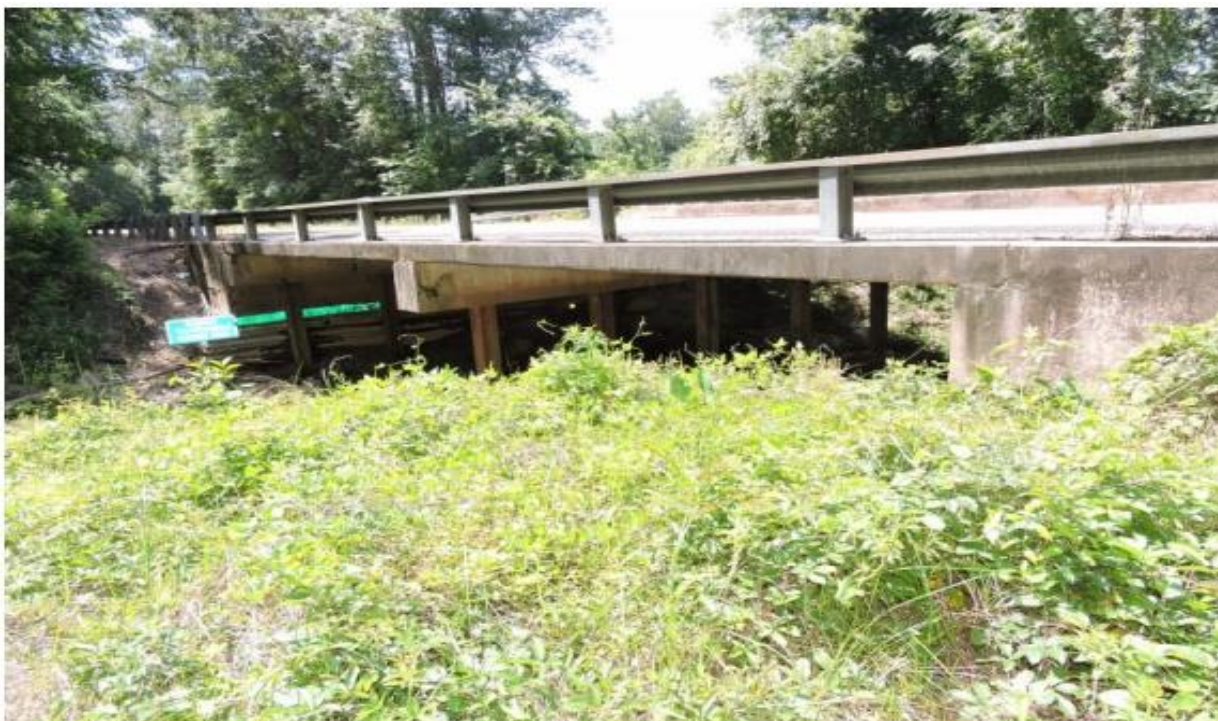
Figure C.37. Bridge CS-19 (TxDOT 2018c)
