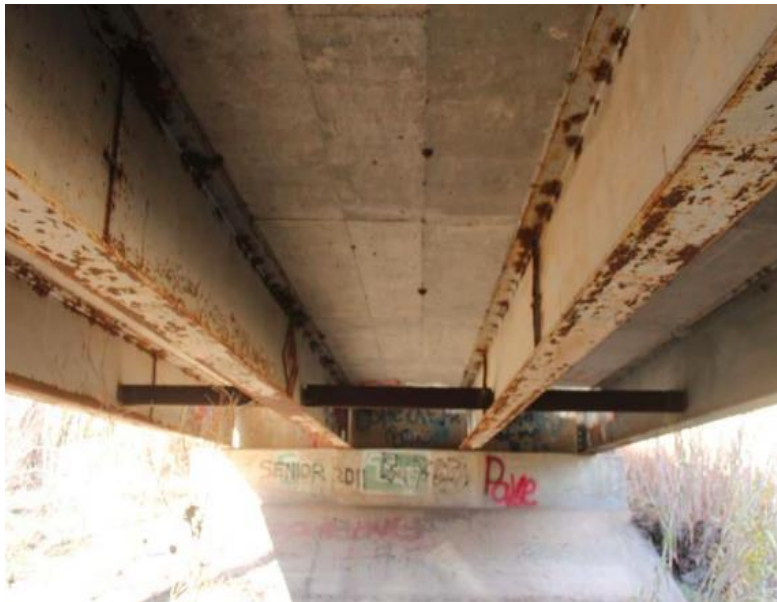
(c) Underside Superstructure View
