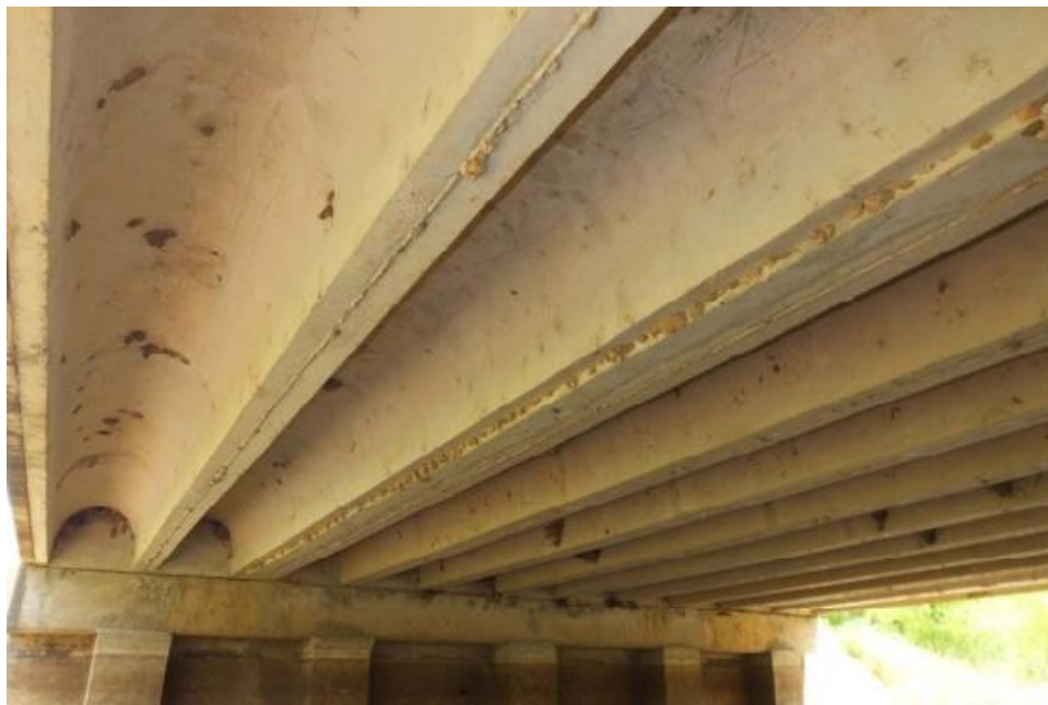
(b) Underside Superstructure View
