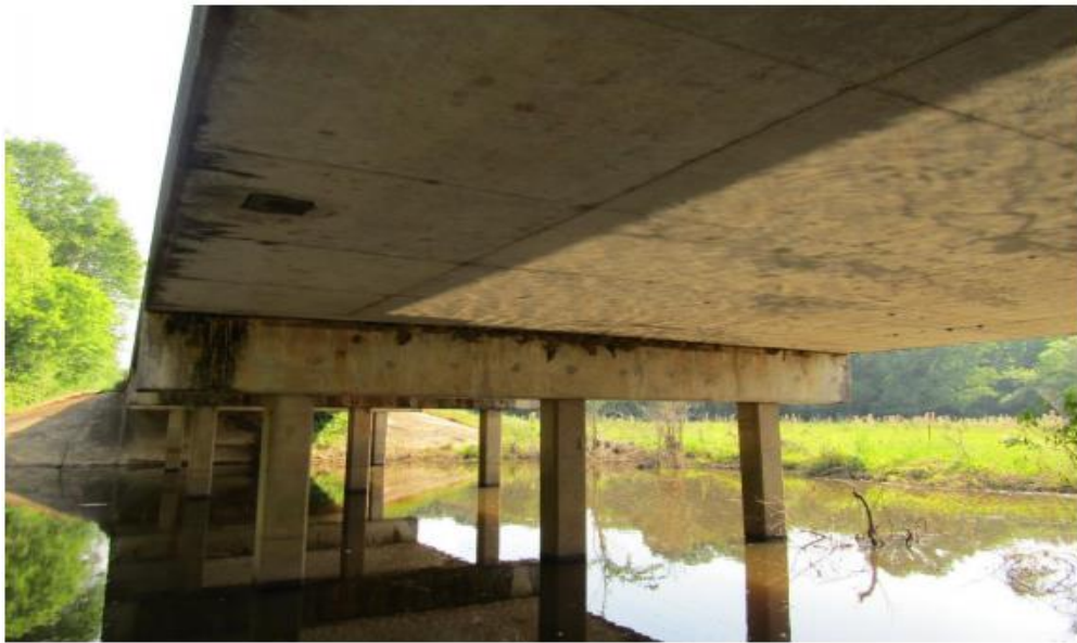
(c) Underside Superstructure View
