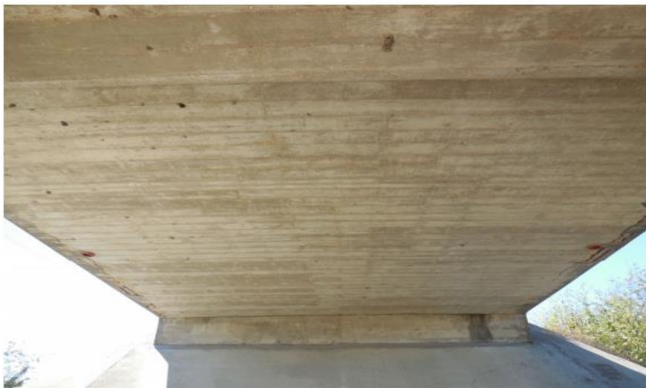
(c) Underside Superstructure View
