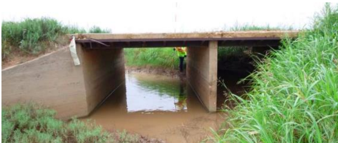
Figure B.67. Bridge SC-9 (TxDOT 2018c)
