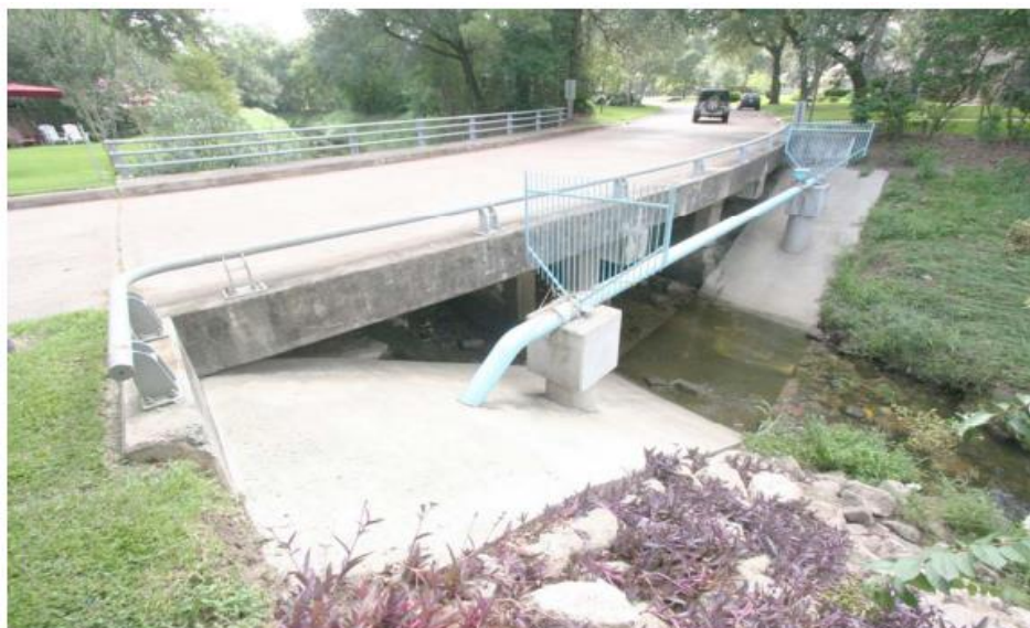
Figure C.43. Bridge CS-22 (TxDOT 2018c)
