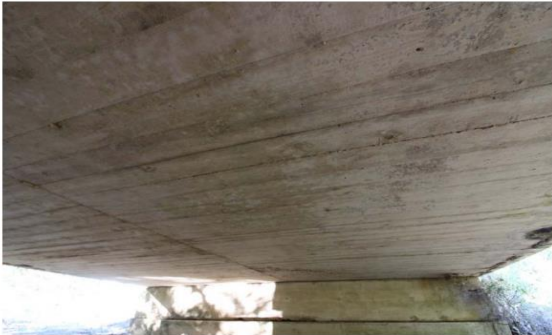
(c) Underside Superstructure View
