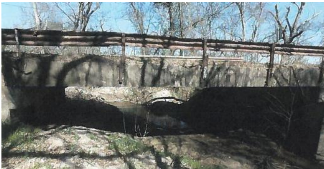
Figure C.55. Bridge CM-5 (TxDOT 2018c)
