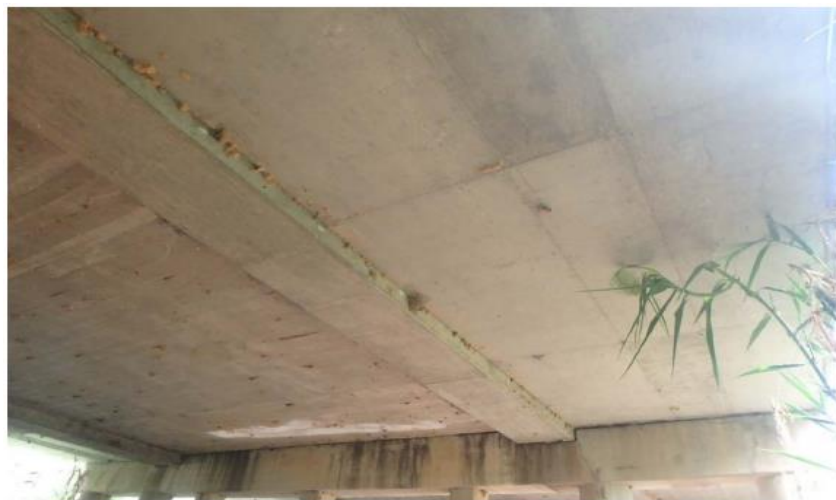
(c) Underside Superstructure View
