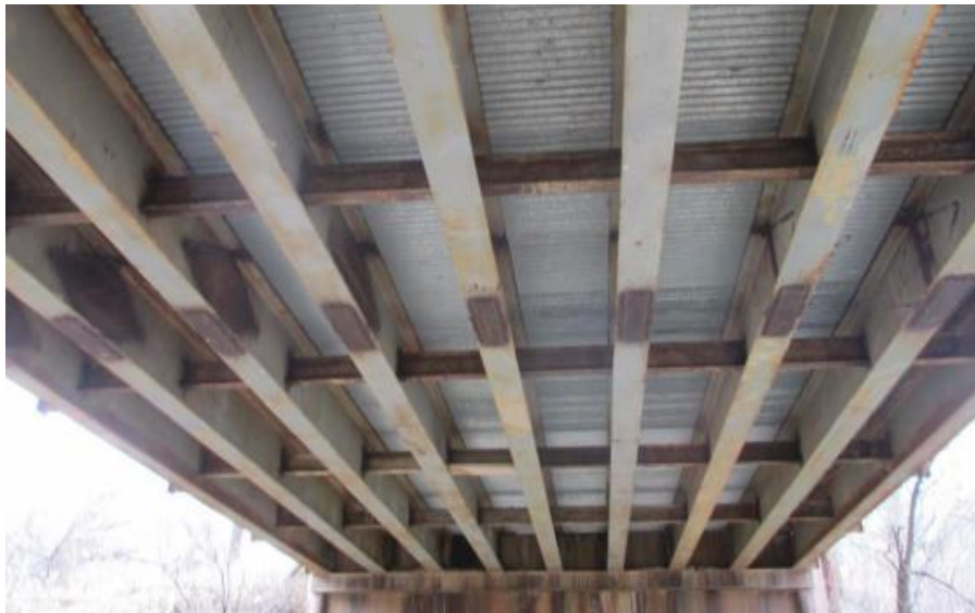
(c) Underside Superstructure View
