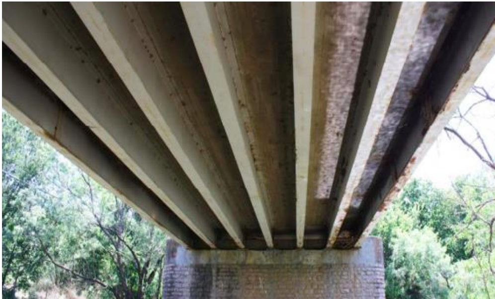
(c) Underside Superstructure View
