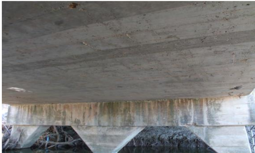
(c) Underside Superstructure View
