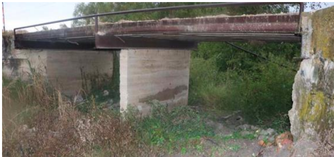
Figure B.51. Bridge SC-1 (TxDOT 2018c)
