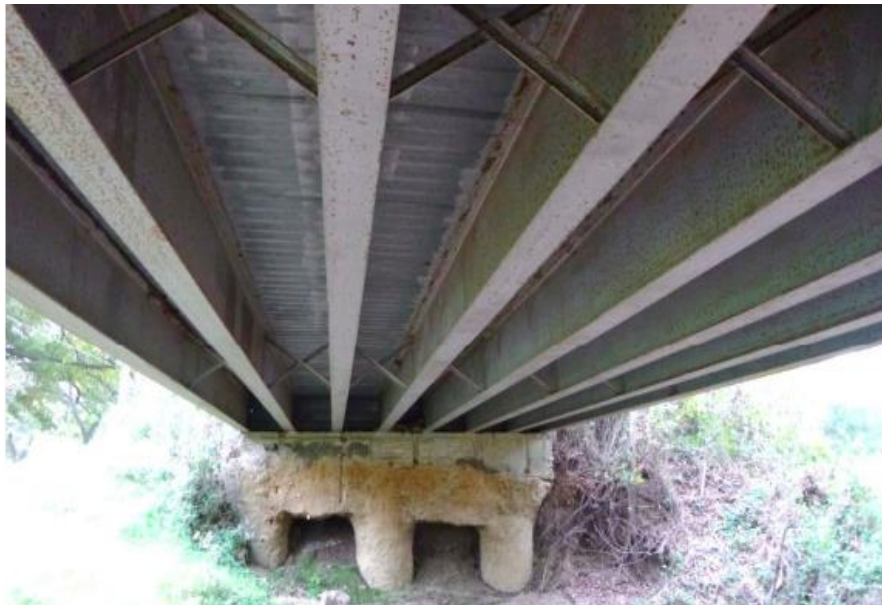
(c) Underside Superstructure View
