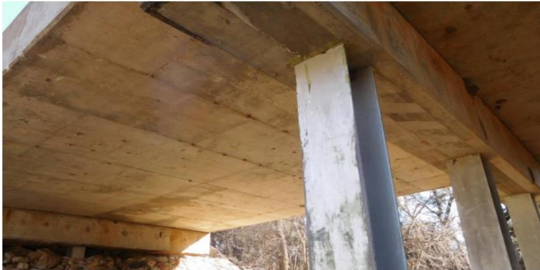
(c) Underside Superstructure View
