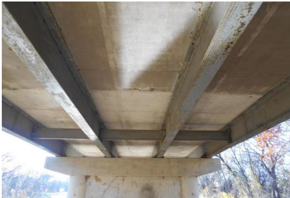
(c) Underside Superstructure View
