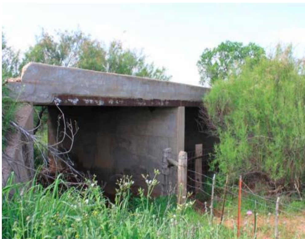
Figure B.71. Bridge SC-11 (TxDOT 2018c)
