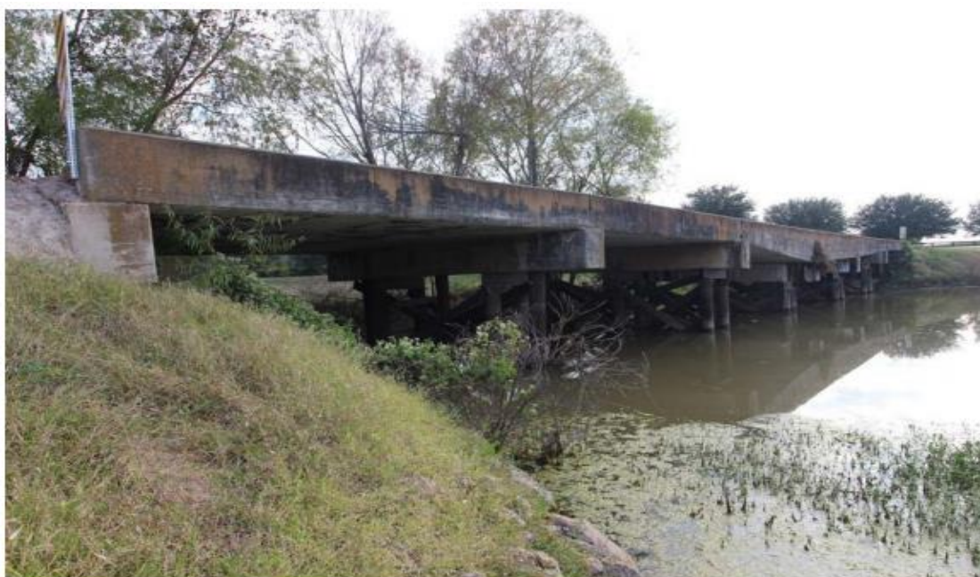
Figure C.13. Bridge CS-7 (TxDOT 2018c)
