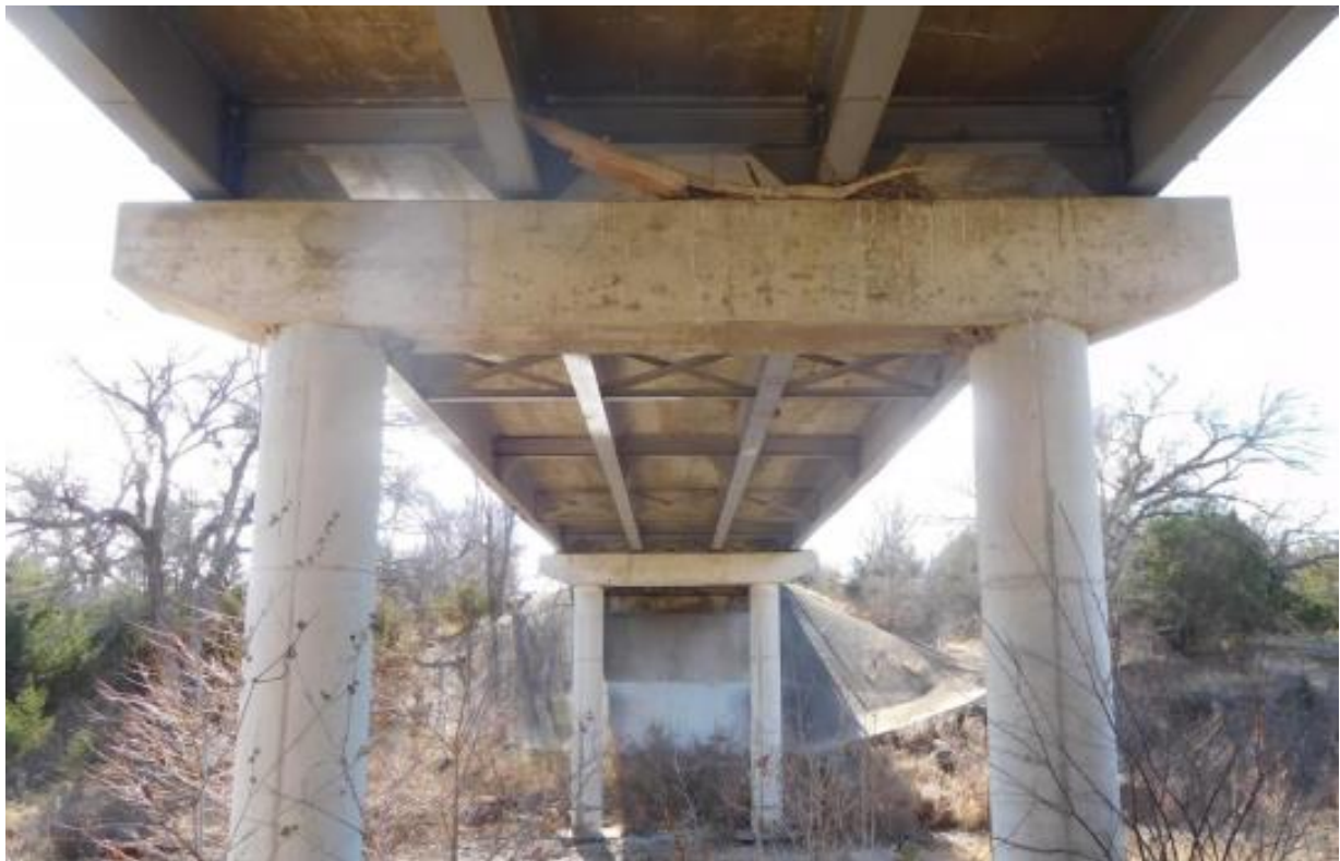
(c) Underside Superstructure View
