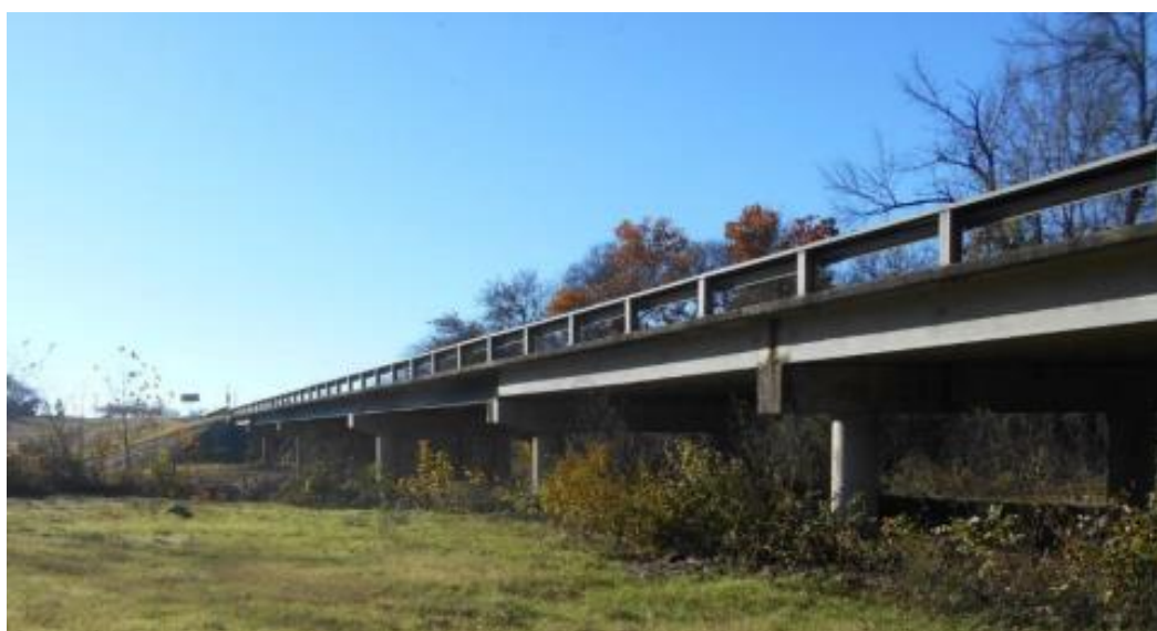
Figure B.75. Bridge SC-13 (TxDOT 2018c)
