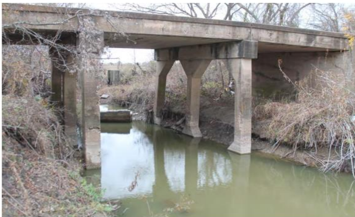
Figure C.1. Bridge CS-1 (TxDOT 2018c)
