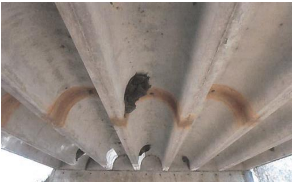
(c) Underside Superstructure View
