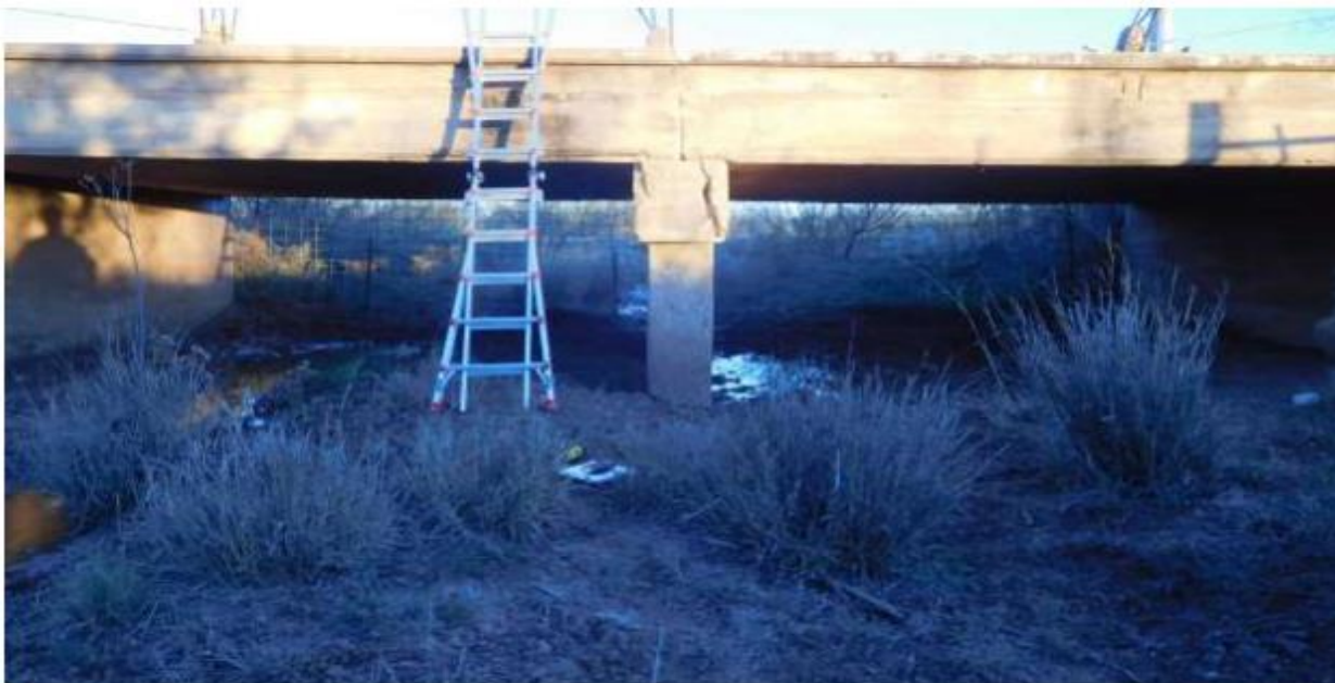
Figure C.3. Bridge CS-2 (TxDOT 2018c)
