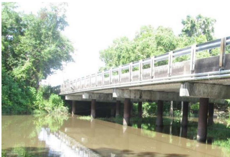
Figure C.65. Bridge CM-10 (TxDOT 2018c)
