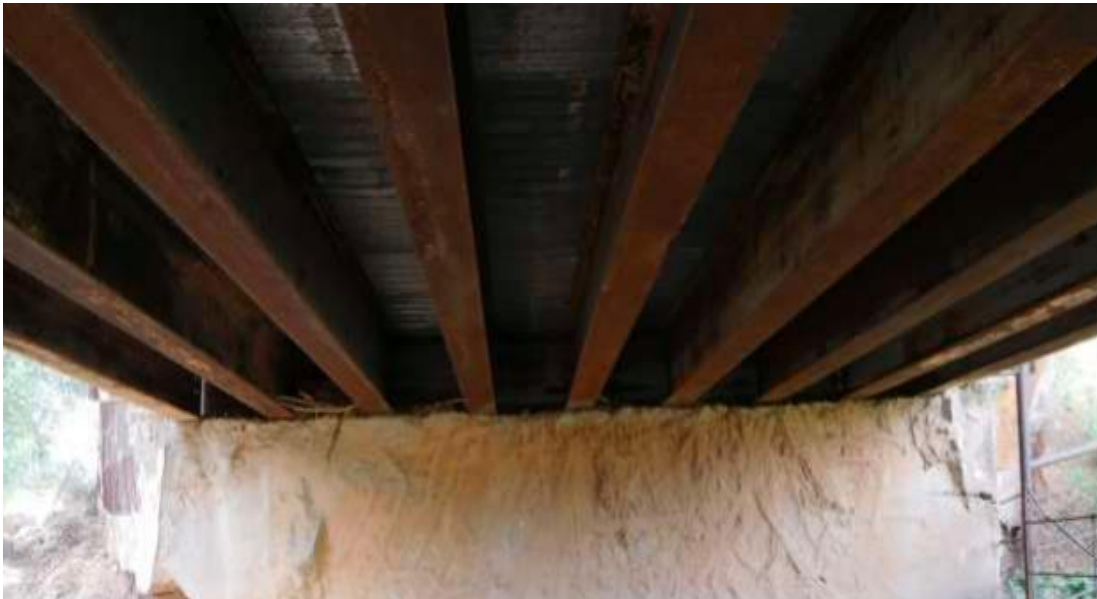
(c) Underside Superstructure View
