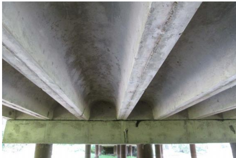
(c) Underside Superstructure View
