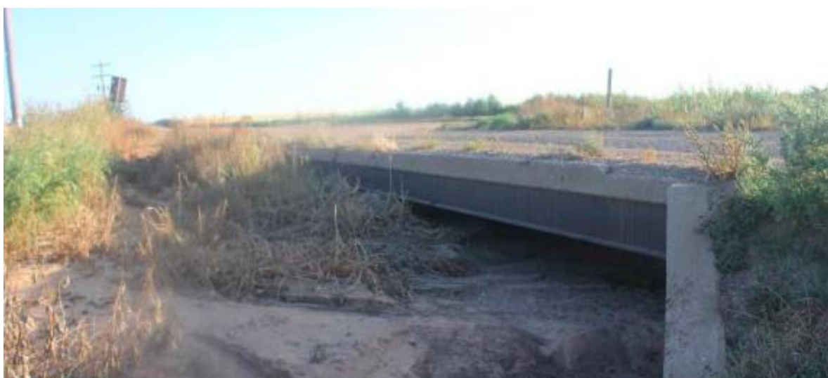
Figure B.11. Bridge SM-6 (TxDOT 2018c)
