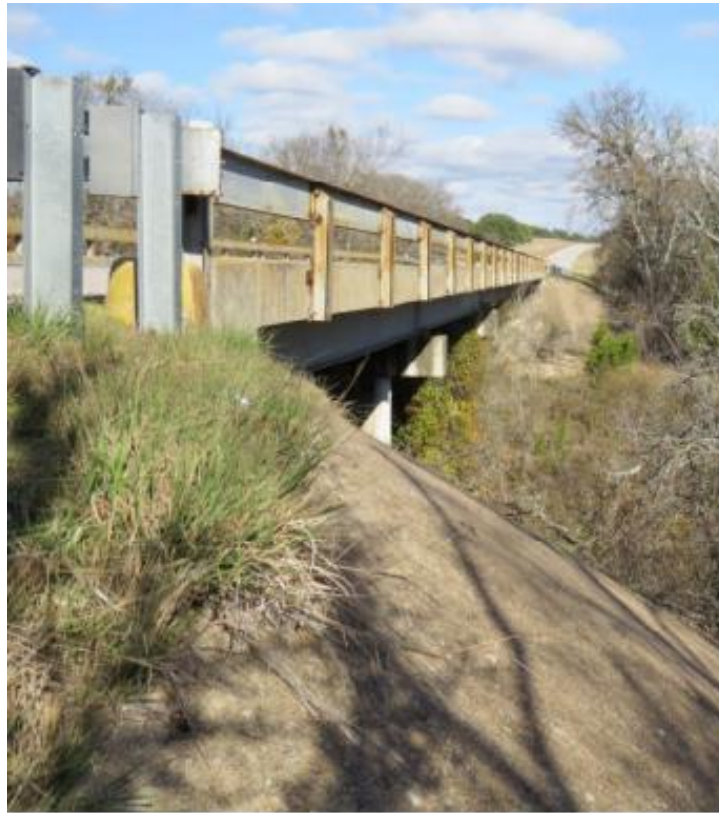
Figure B.29. Bridge SM-15 (TxDOT 2018c)
