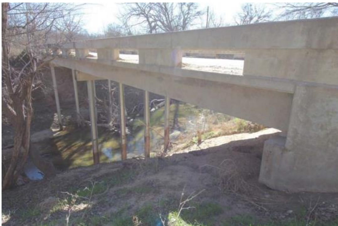
Figure C.71. Bridge CM-13 (TxDOT 2018c)
