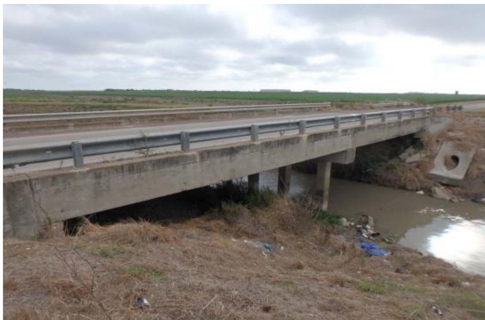
Figure C.69. Bridge CM-12 (TxDOT 2018c)
