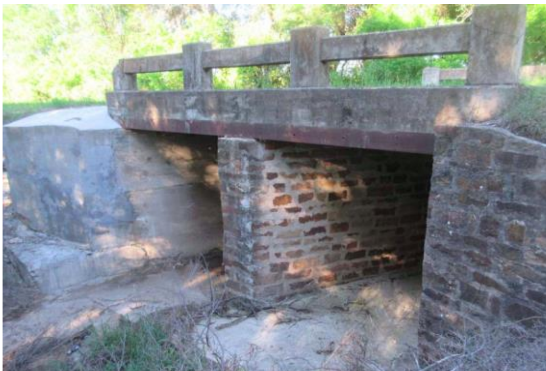
Figure B.63. Bridge SC-7 (TxDOT 2018c)
