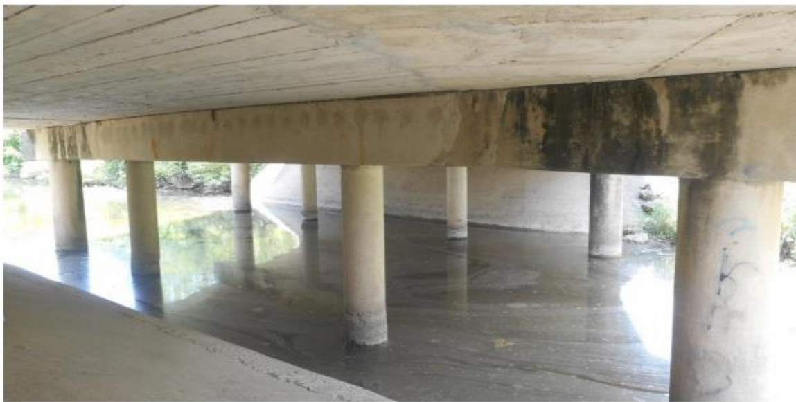
(c) Underside Superstructure View
