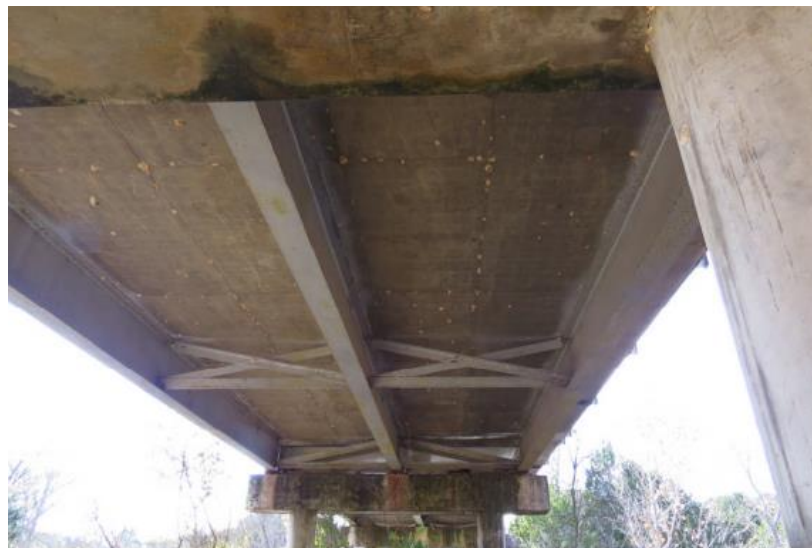
(c) Underside Superstructure View
