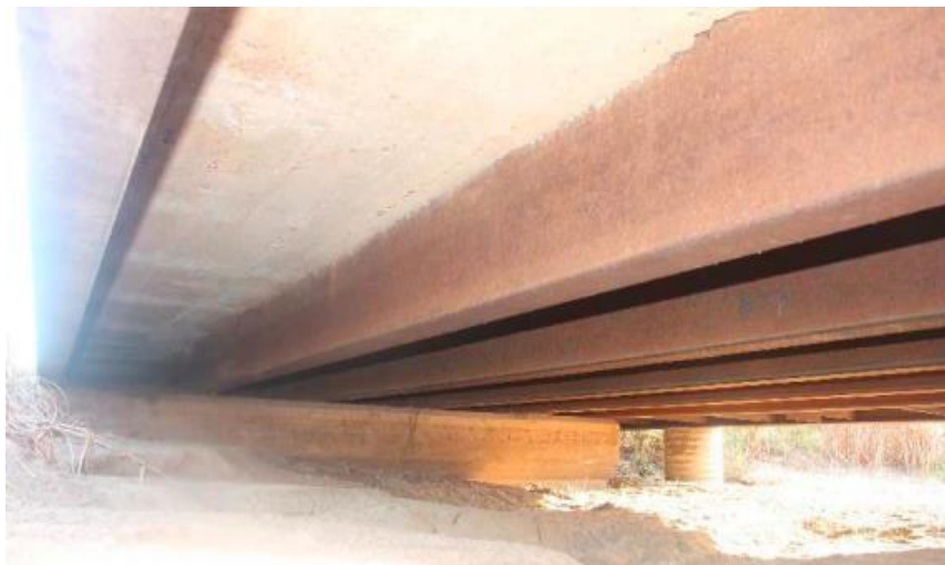
(c) Underside Superstructure View
