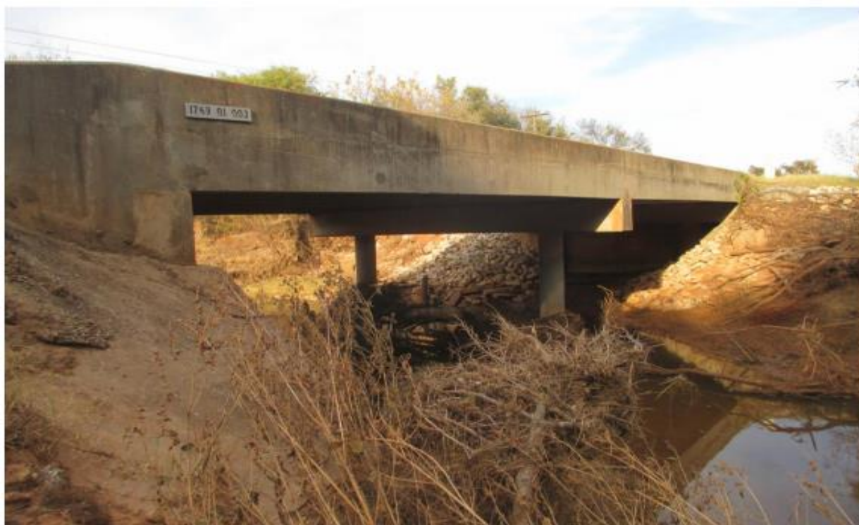
Figure C.57. Bridge CM-6 (TxDOT 2018c)
