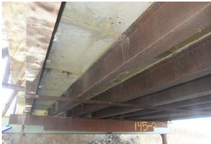
(c) Underside Superstructure View
