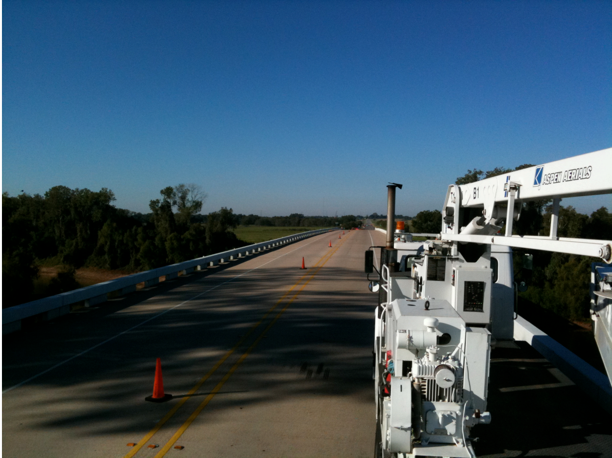
Figure 5.15. Traffic Control (toward Bellville).
