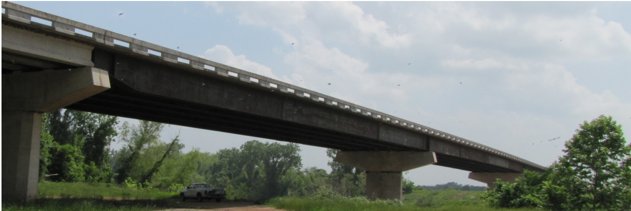
Figure 4.1. SH 159 Brazos River Bridge.
