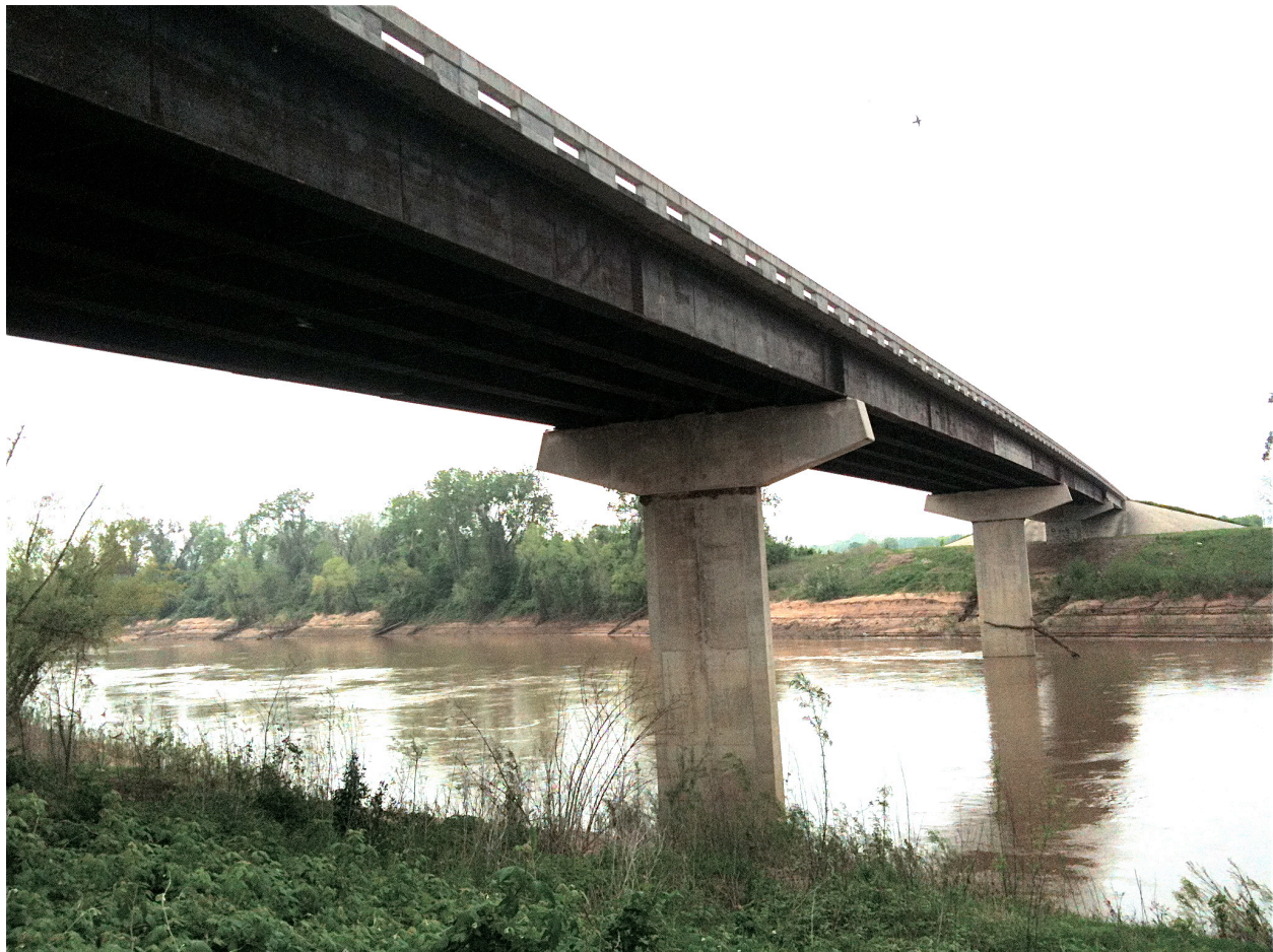
Figure 5.11. SH 159 Brazos River Bridge (Study Bridge).
