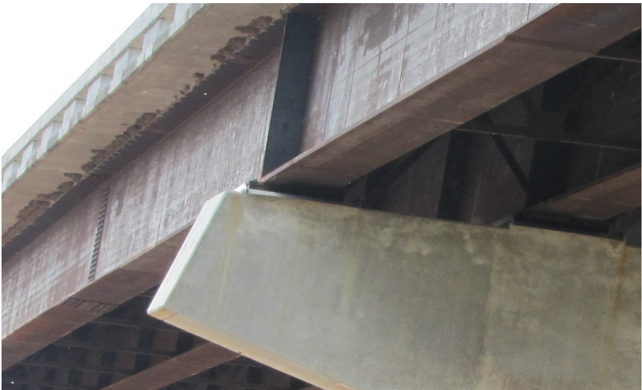
Figure 4.3. Flange Supports.
