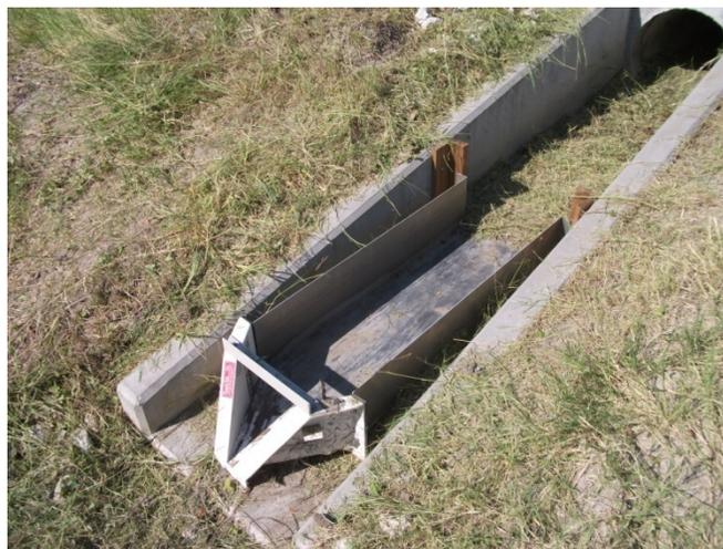
**Figure 9. H-Flume at the Influent Location to Measure Flow.**
