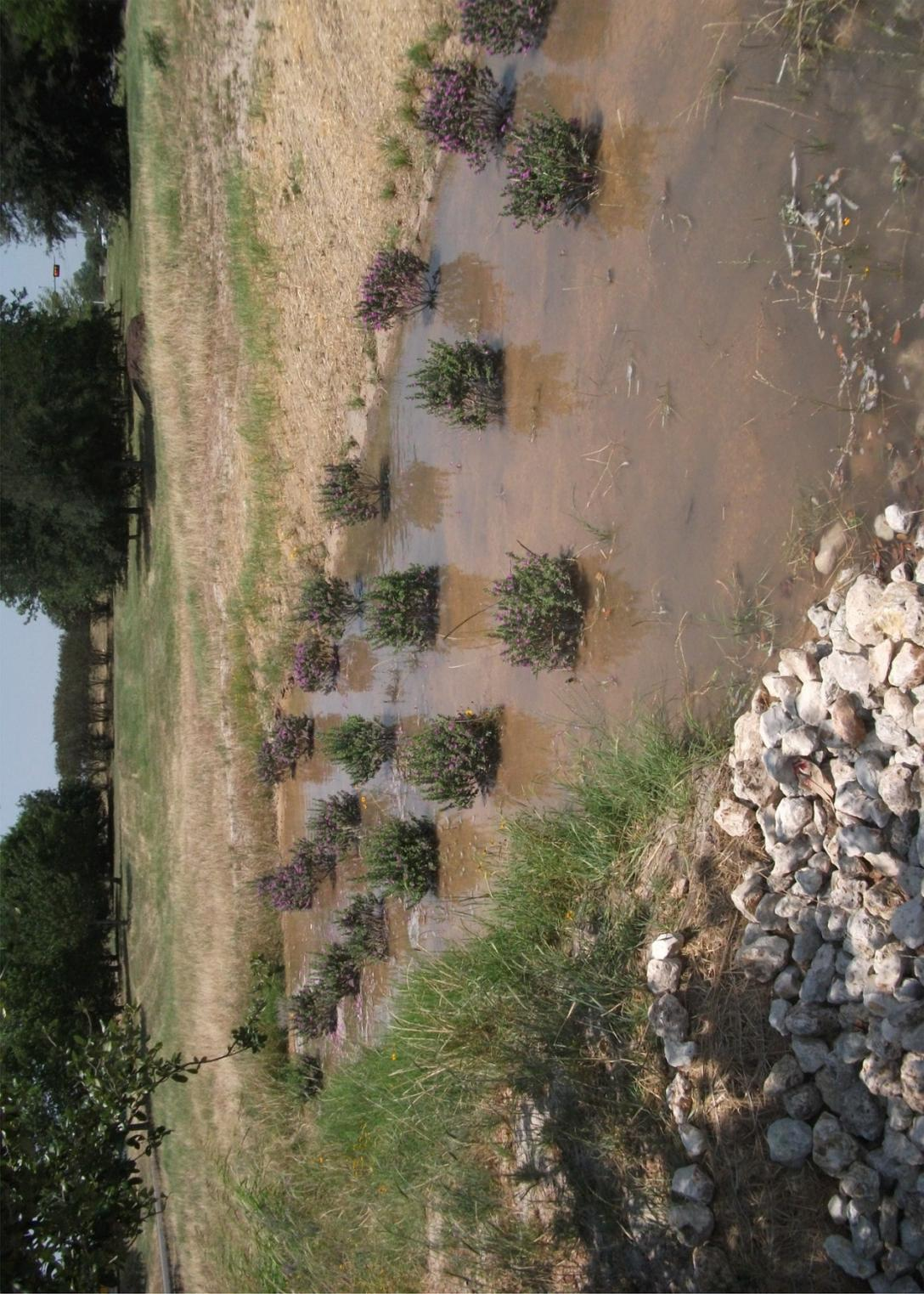
**Figure 8. Flood Irrigation of Bioretention Cell (Photo Taken in June 2011).**
