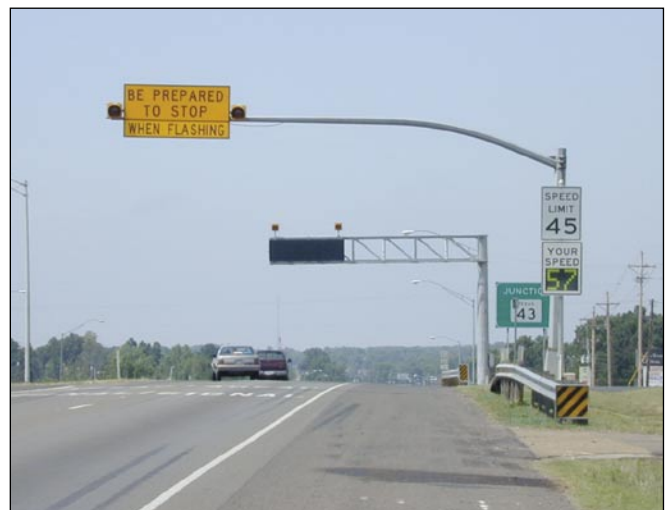
Figure 3. DSDS effect may be enhanced at a restricted sight distance location.
