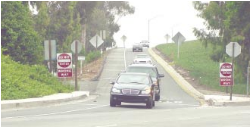
Three states use lowered signs mounted on the same posts to increase visibility.
