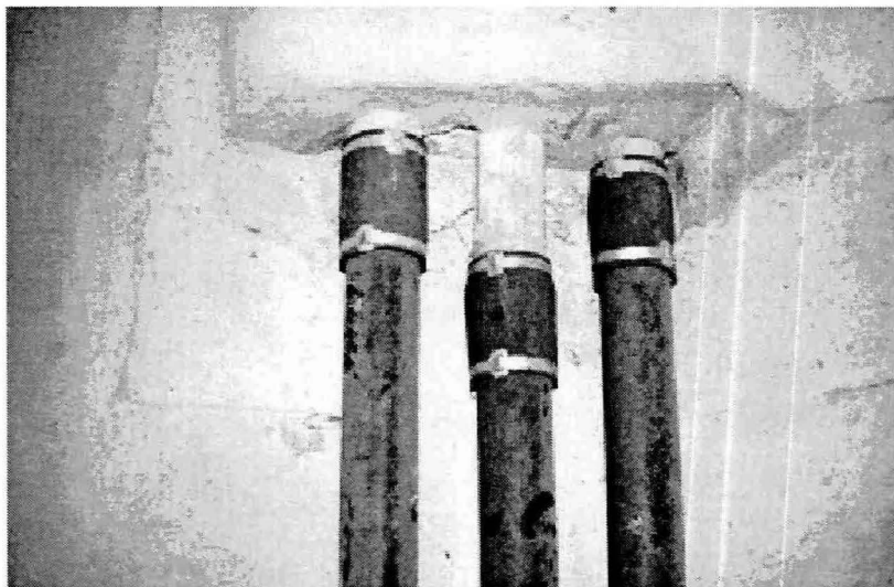
Figure 2.5 Plan View of Slipped Tendon at Deviation Saddle – Niles Channel Bridge 16
