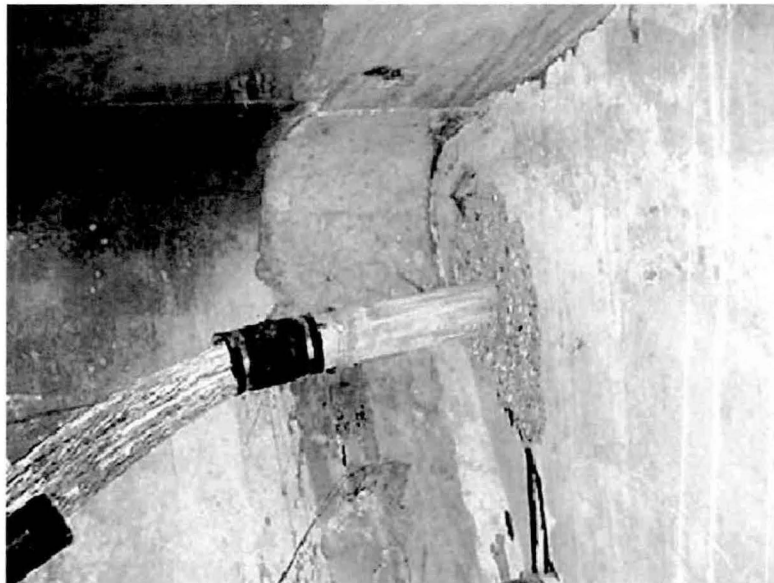
Figure 2.9 Failure of Tendon 57-1 on the Mid-Bay Bridge at Expansion Joint Diaphragm 16
