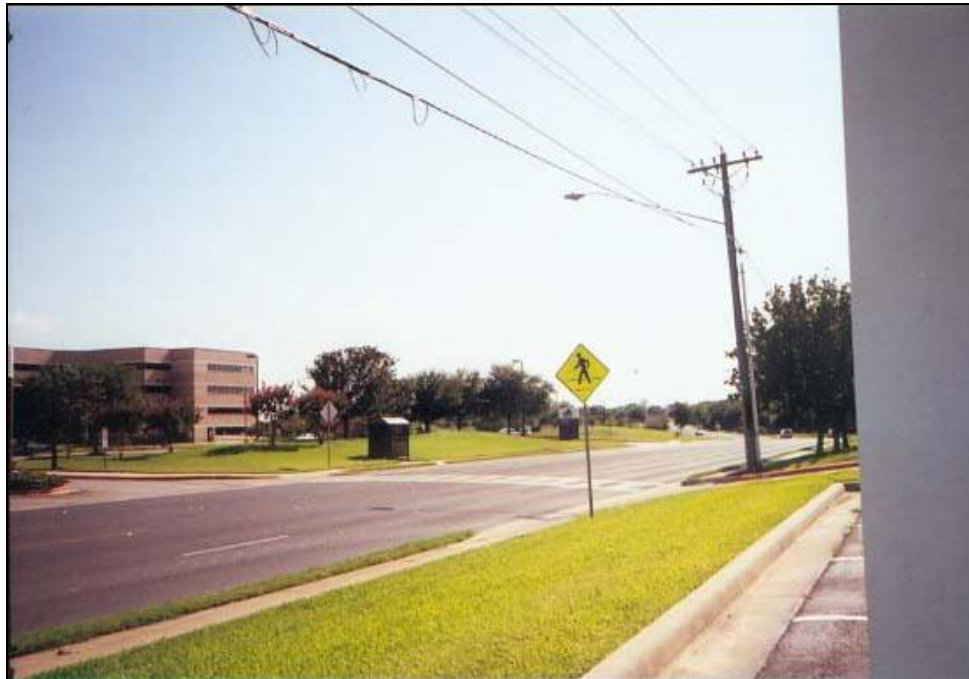
Figure 14. Westward View of Rock Prairie Crosswalk
