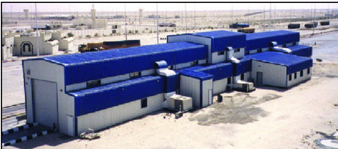
Figure 5. Inspection System at Middle East Port Facility ( 17 )
