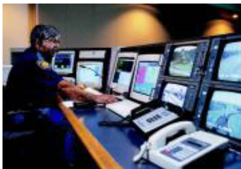
Figure 5. Police Co-Location at TransGuide in San Antonio
