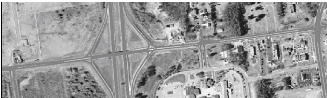
Figure 1. Existing Route 67 Corridor
