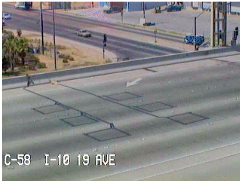
Figure 2. Inductive Loop Detectors in Pavement for Traffic Flow Data
