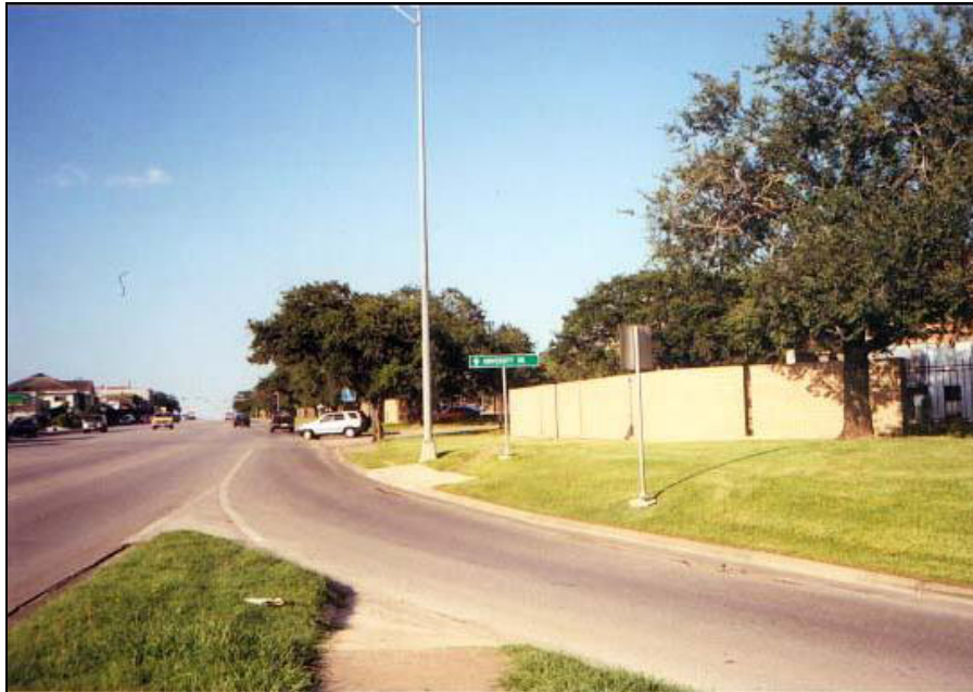
Figure 18. Eastward View of Wellborn Rd. at University Dr.
