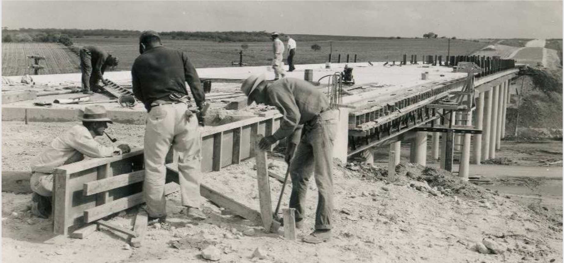
T&NO Railroad Overpass, Karnes County Let November 1956 • Completed June 20, 1957
