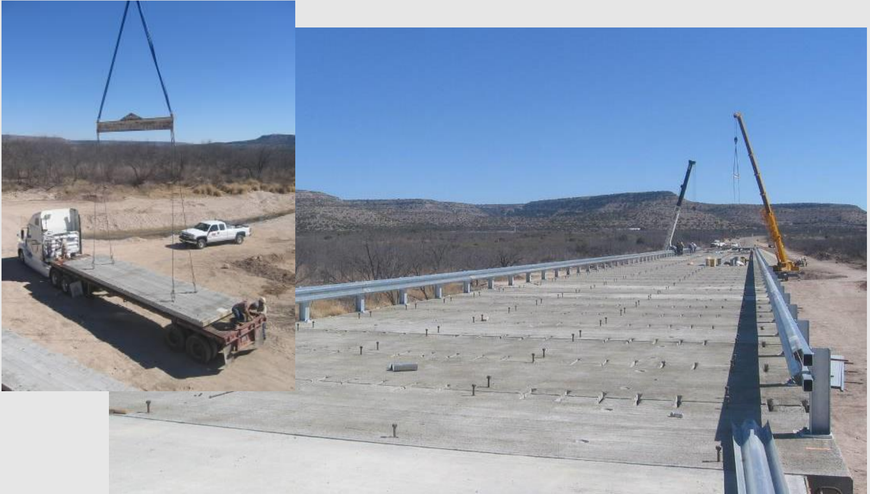
Precast Full-depth and Full-width Deck Panels
