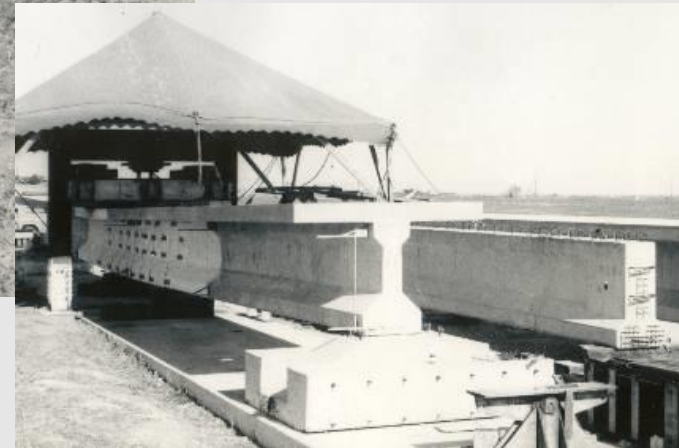
Full scale pretensioned beam tests, 1959
