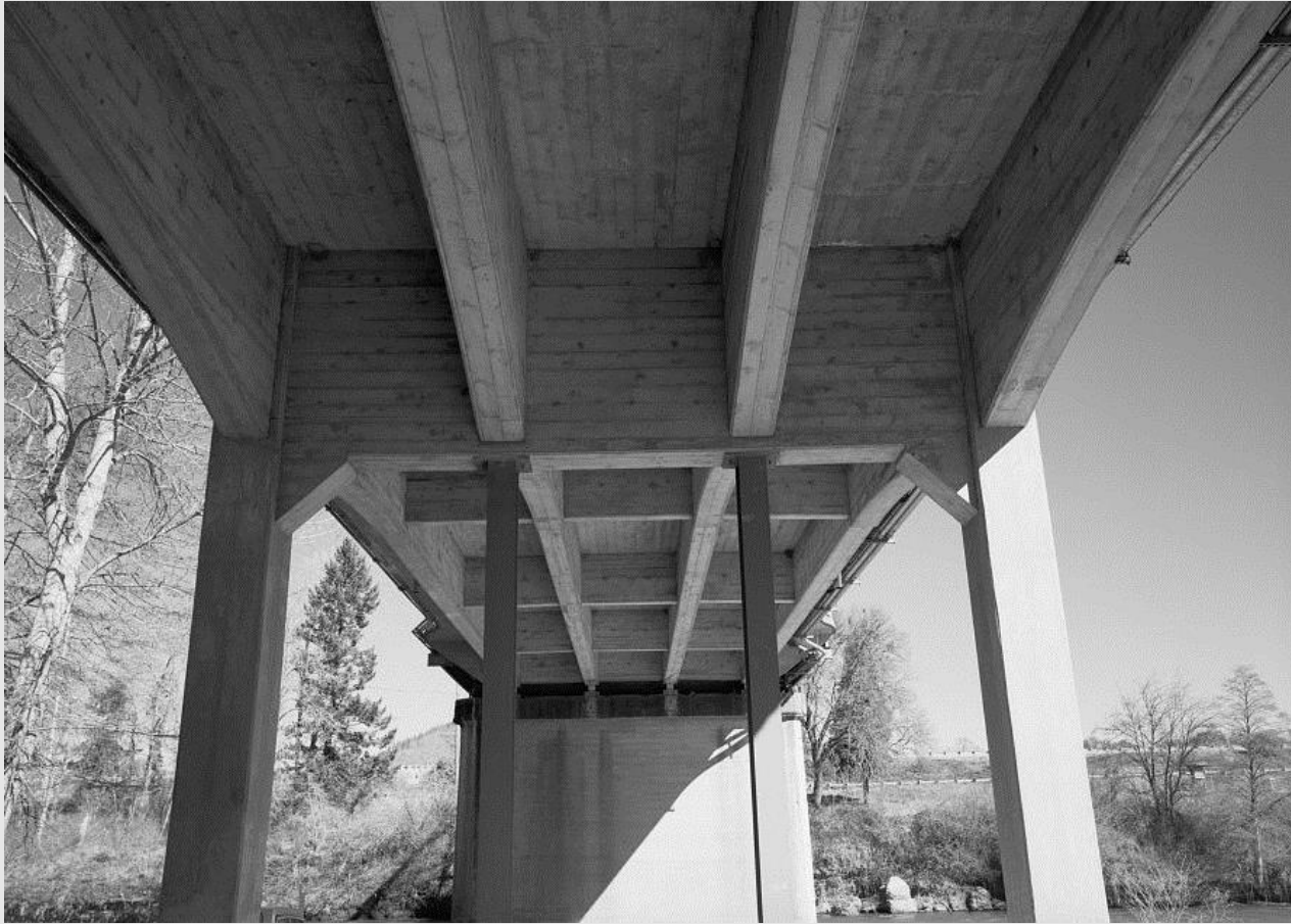
1900s - T Beam Bridges
