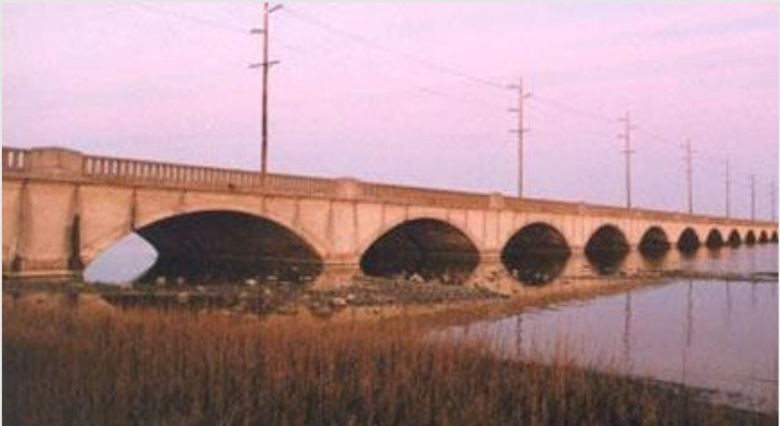
1900s – Reinforced Concrete Arch Bridges
