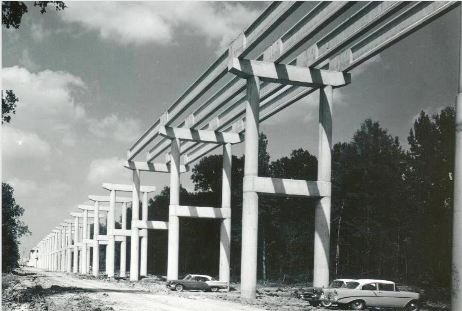
Angelina River Bridge construction, SH 147, 1958
