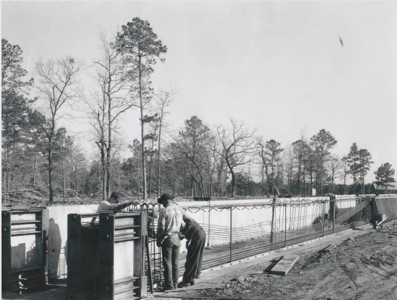
Prestressed concrete plant operations, Lufkin
