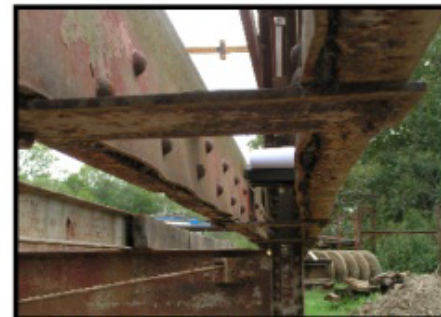
PACK RUST ON UNDERSIDE OF STRINGER
