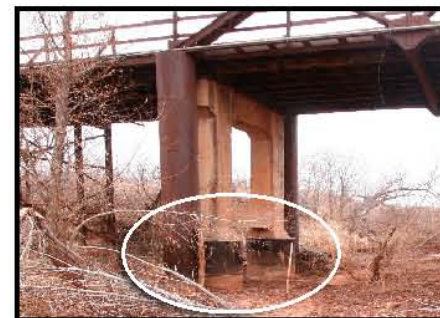
SEVERE EROSION AT BRIDGE BENT
