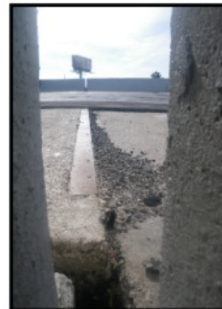
DEBRIS AND RUBBLE IN DECK JOINT
