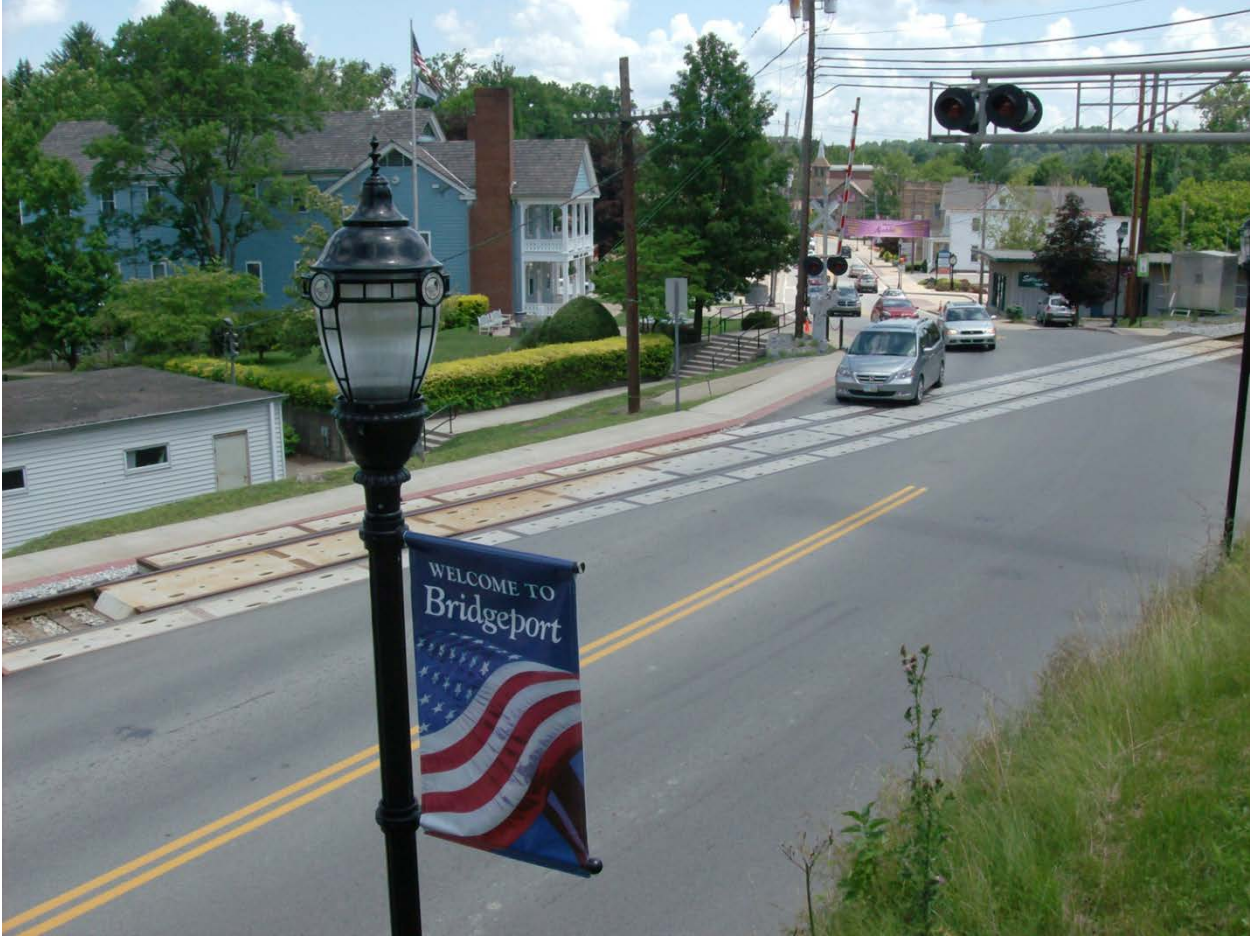
Figure 8. Recently Completed 144-ft (44-m) long Crossing on US 50 on CSX Line in Bridgeport, WV.
